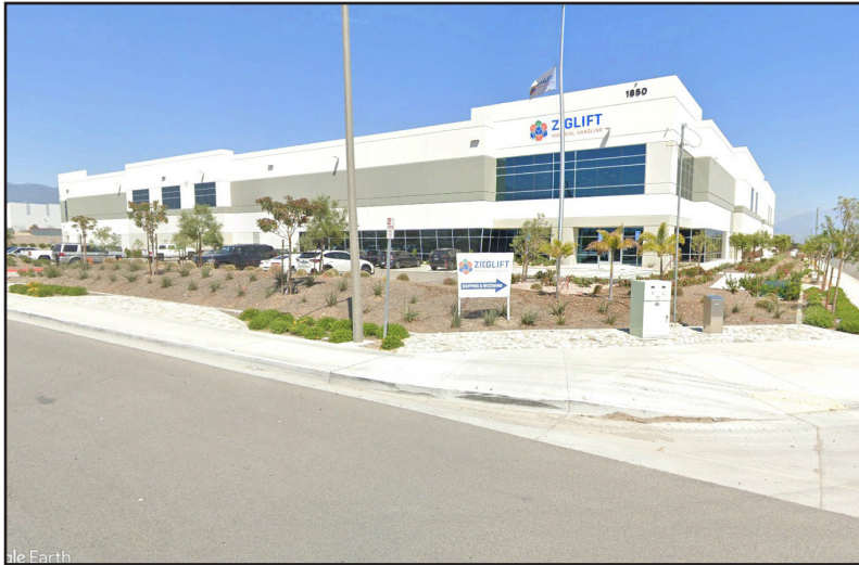
E. Looking at the industrial use north of the site, north of Vineyard Avenue
