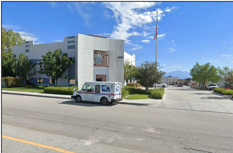
C. Looking at the north building at 2271 N. Locust Avenue from Locust Avenue
