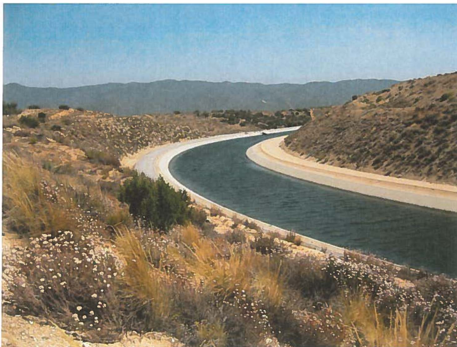
EBA Canal near Hesperia, facing south
