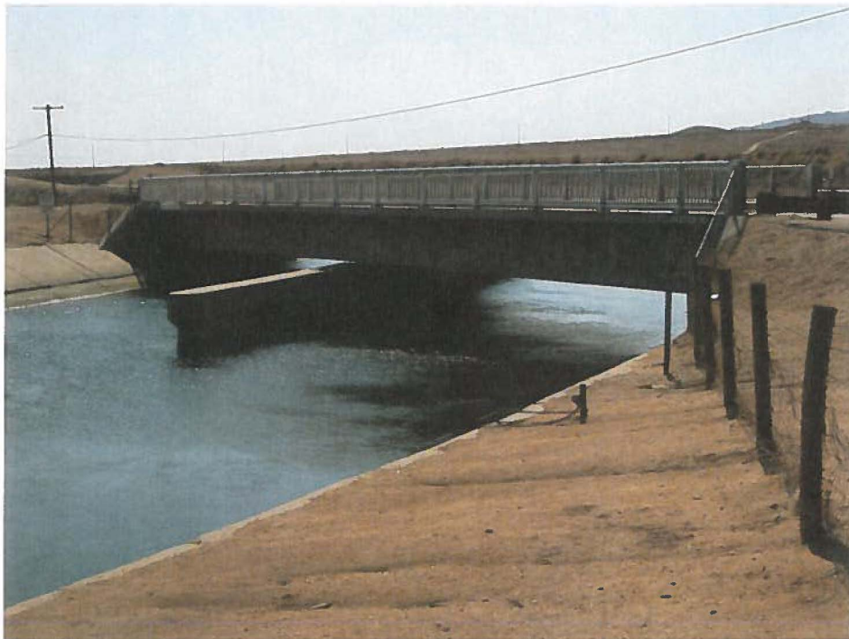
Lancaster Bridge and EBA Canal, facing northwest
