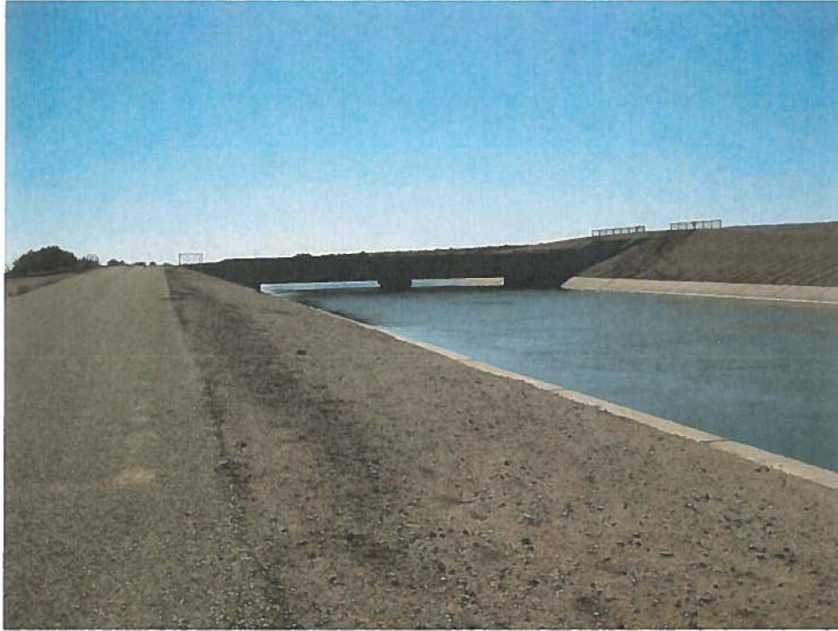
EBA canal and double overchute, facing southwest
