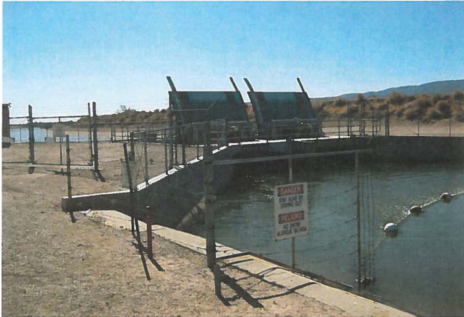
Figure 2. Canal Check Structure, facing southwest
