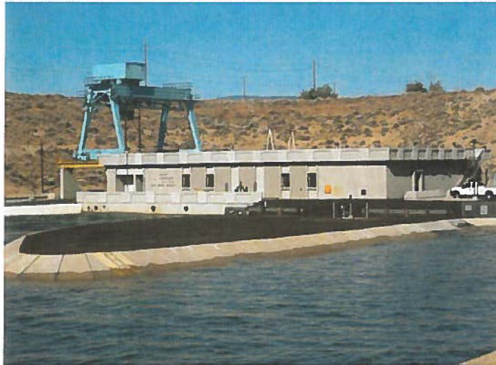
Figure 7. Alamo Power Plant, facing northwest
