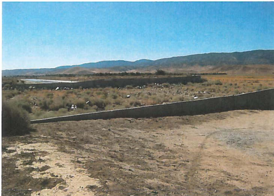
Figure 2. Box Siphon, facing southwest
