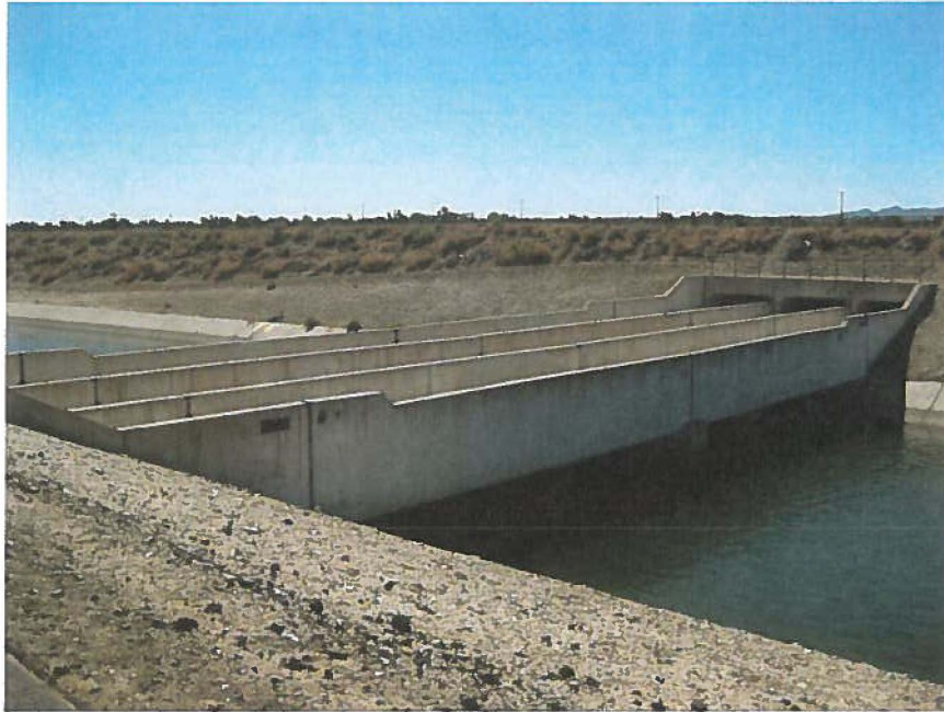
Figure 5. Triple Overchute, facing southwest
