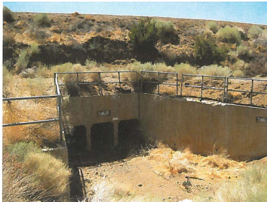
Figure 6. Triple Box Culvert, facing south
