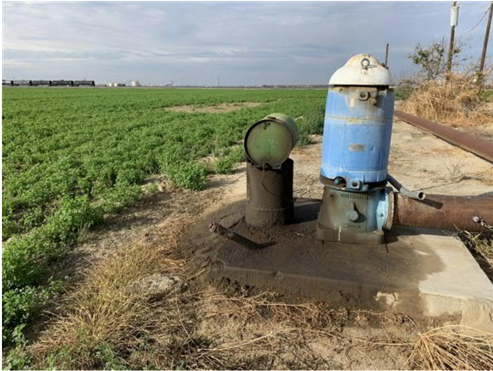
Photo 5: View of the water well located along the eastern boundary within the northeastern part of the subject site. A lube-oil drum is present and the wellhead concrete pad is oil stained. Minor staining of the soil was noted around the concrete pad. A pole-mounted transformer (background right) provides electrical power to the water well.
