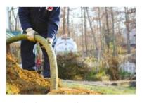
closest to the house). Use a shovel to push the scum layer away from the side of the tank to estimate its thickness. If the scum layer is more than one foot thick, have your tank pumped immediately! Replace the manhole cover and wash your hands and shovel. Yearly inspection of the septic tank is strongly recommended. Check your phone book yellow pages for a licensed Septic Tank Pumper. If your tank does not have risers to grade, install them over both chambers.
