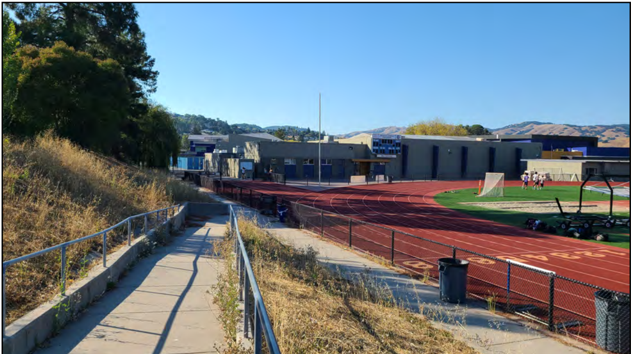
Facing west from the ramp between the track and field stadium and baseball field with a view of Building K and the portable structure (Building Q/R) that is proposed for removal.
