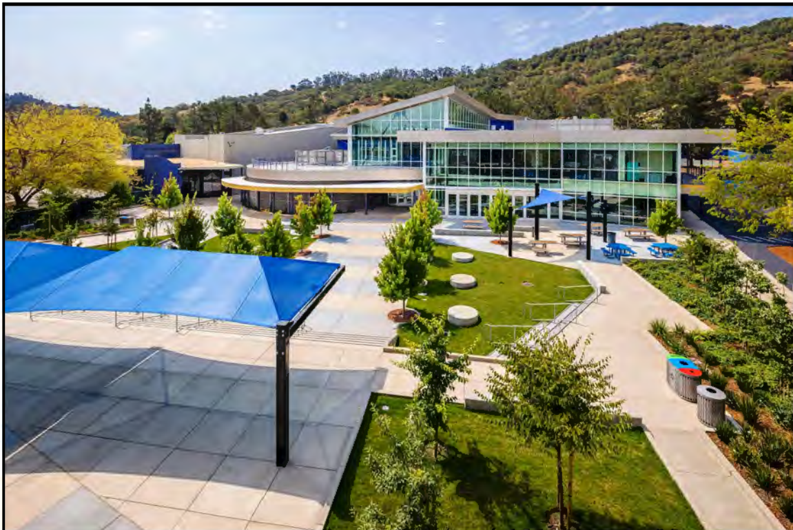
Facing south with a view of the school courtyard and the north side of the Student Commons. The north-facing side of Sorich Park is in the background.
