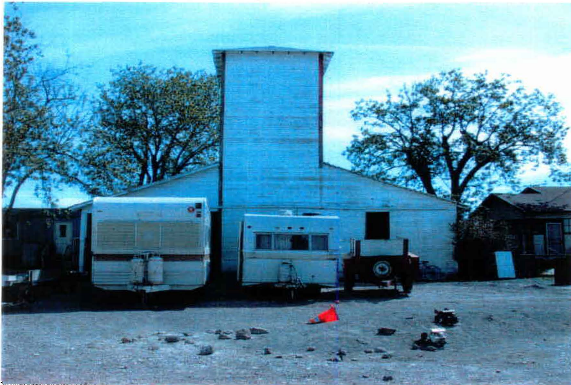
Photograph No. 5. View of old well/pump house used to provide drinking water to the residences living on the Mistler property. Tower of building previously housed a water storage tank.
