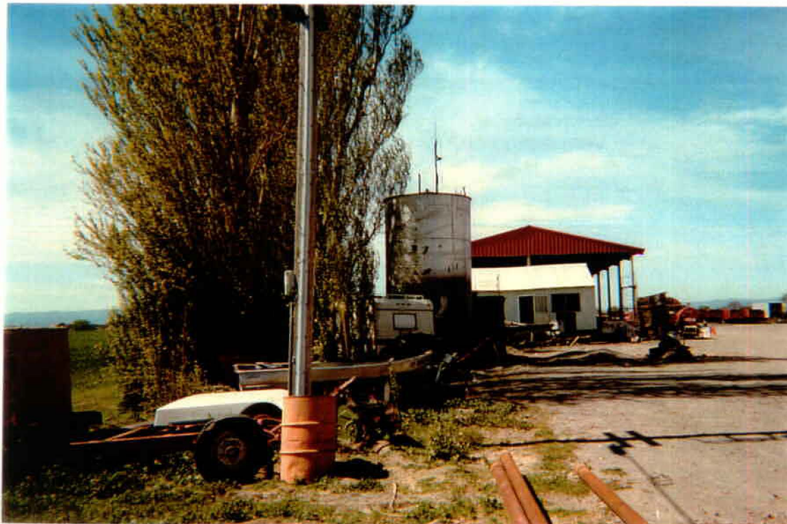
Photograph No. 10. View of 55-gallon drum (appeared to be full of spent motor oil) and diesel AST (approximately 10,000 gallon) seen in background and in center of Mistler property looking west. AST has a pump and dispenser attached to it. According to the property owner the AST is no longer being used.
