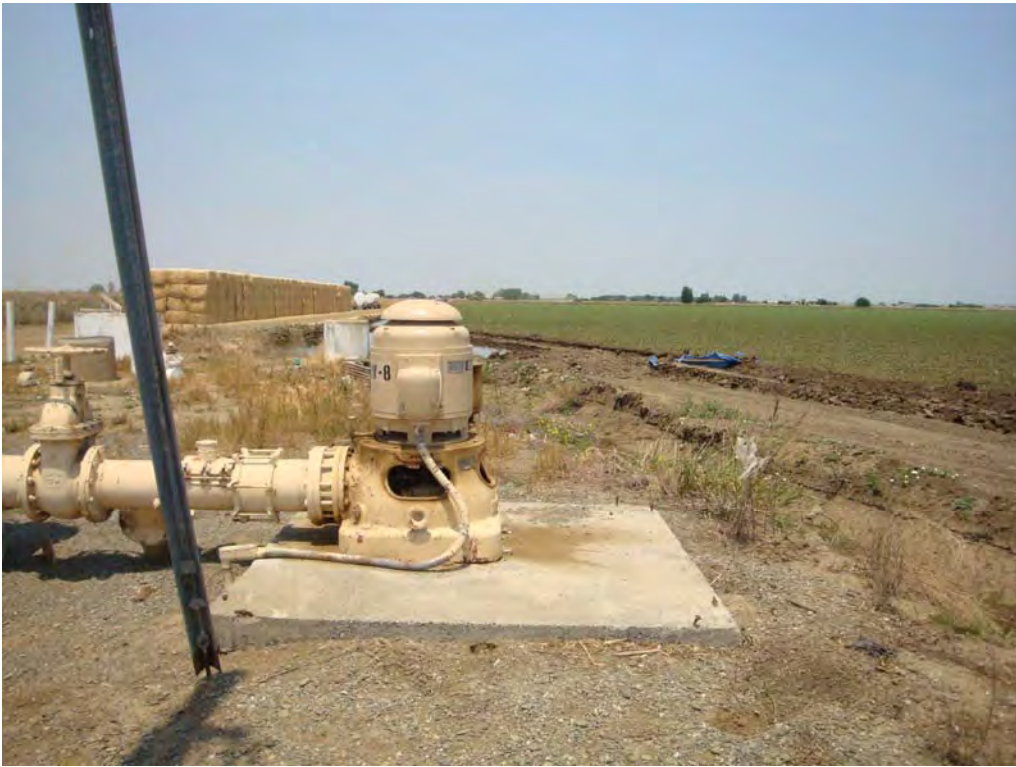
Photo 14 - Parcel 111-080-050 (H) one irrigation well, labeled DW-8.
