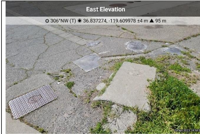
Photo 17 – Water vault and patched asphalt from previous site investigations. View northwest.
