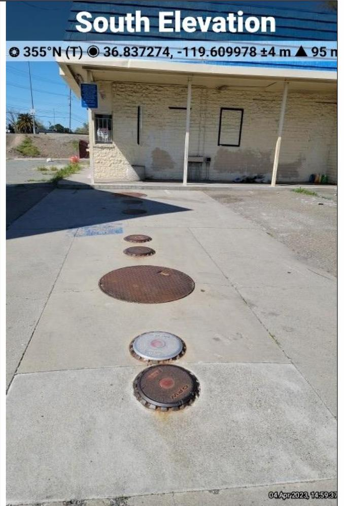
Photo 20 – Tank filling ports. View north.
