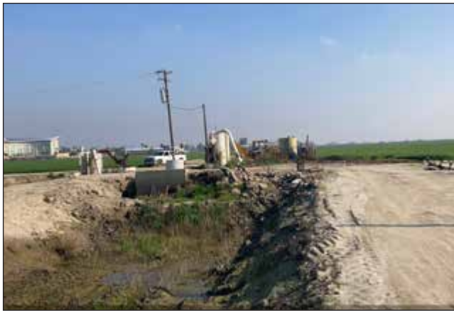
PHOTO 1: Irrigation ditch and associated infrastructure on the Property.
