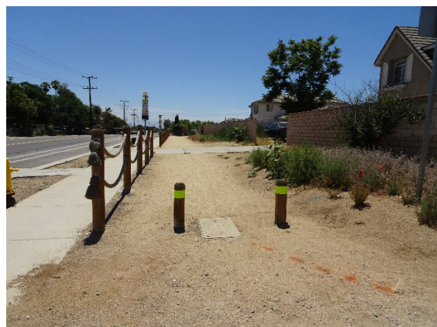
Multi-use trail along Grand Avenue.
