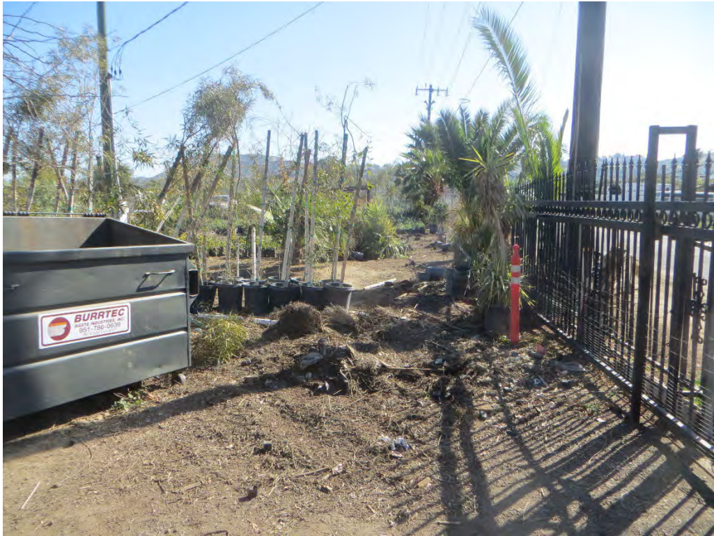
Photograph 6: From the southwest corner of the project site looking east along the southern boundary.
