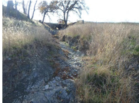
Photograph 4. ES-2 looking upstream from near IS-1. Orientation: west.
