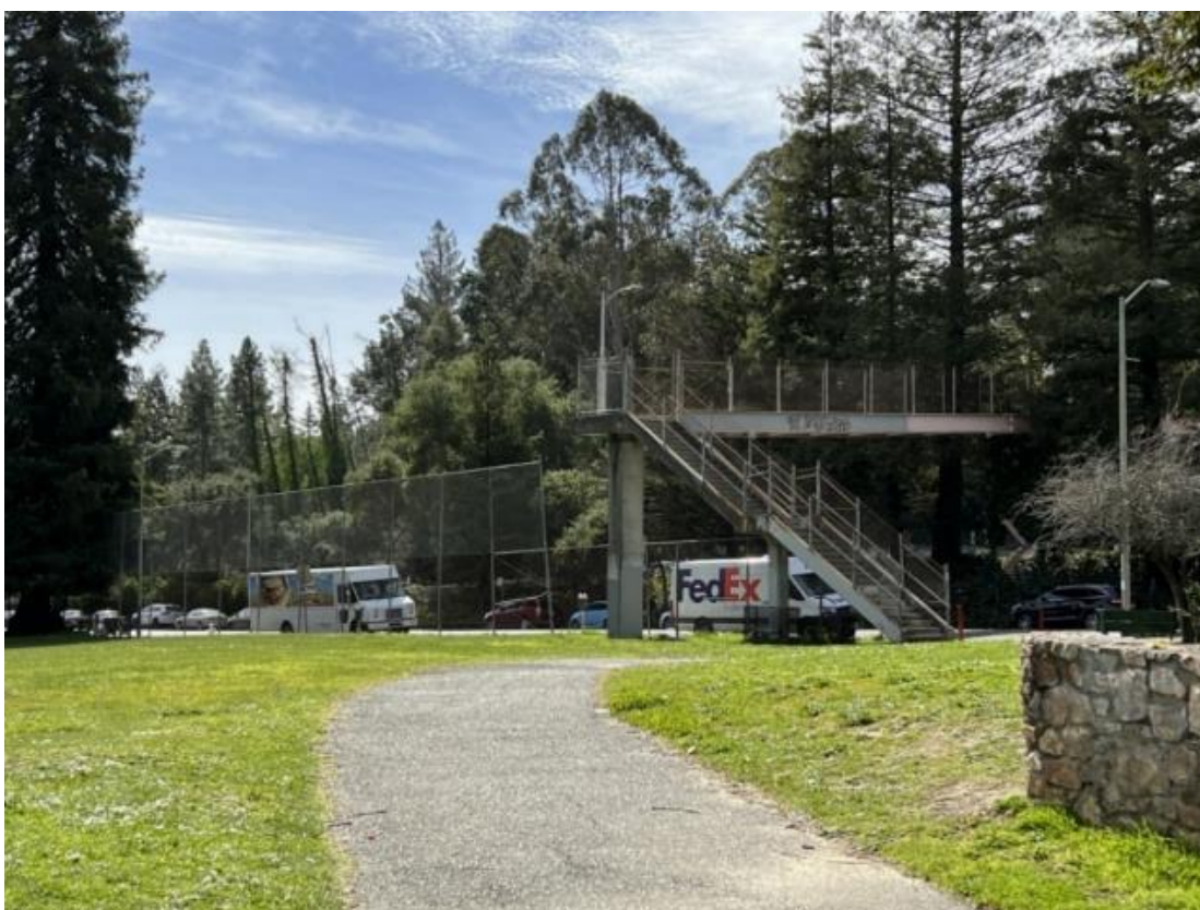
Figure 1-3. Existing Conditions at Bruns Court POC. View west from Montclair Park.
