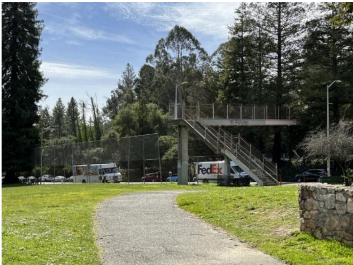
Figure 1-9. View of Existing Touchdown in Montclair Park. View west.
