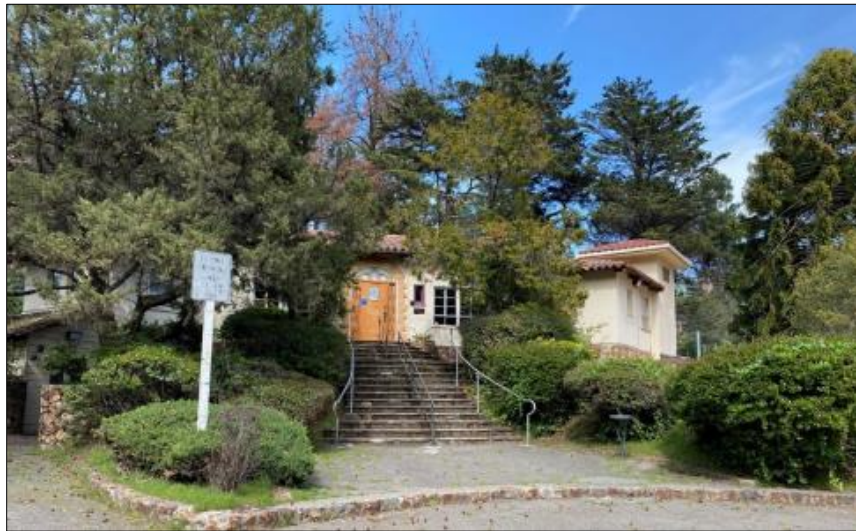
Figure 25. Montclair Park Recreation Center (I. Peña, Caltrans, December 2021)
