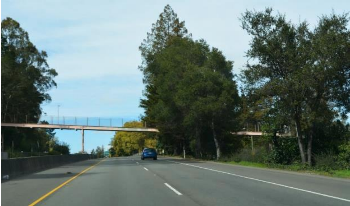
Figure 1-8. View of Existing POC from SR-13. View north.
