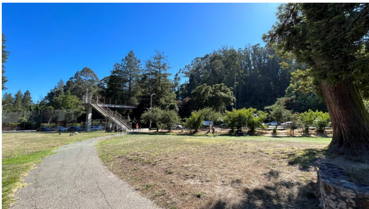
Figure 2-5. Alternative 3a/b. Existing view of pedestrian overcrossing from Montclair Park Trail. View southwest.
