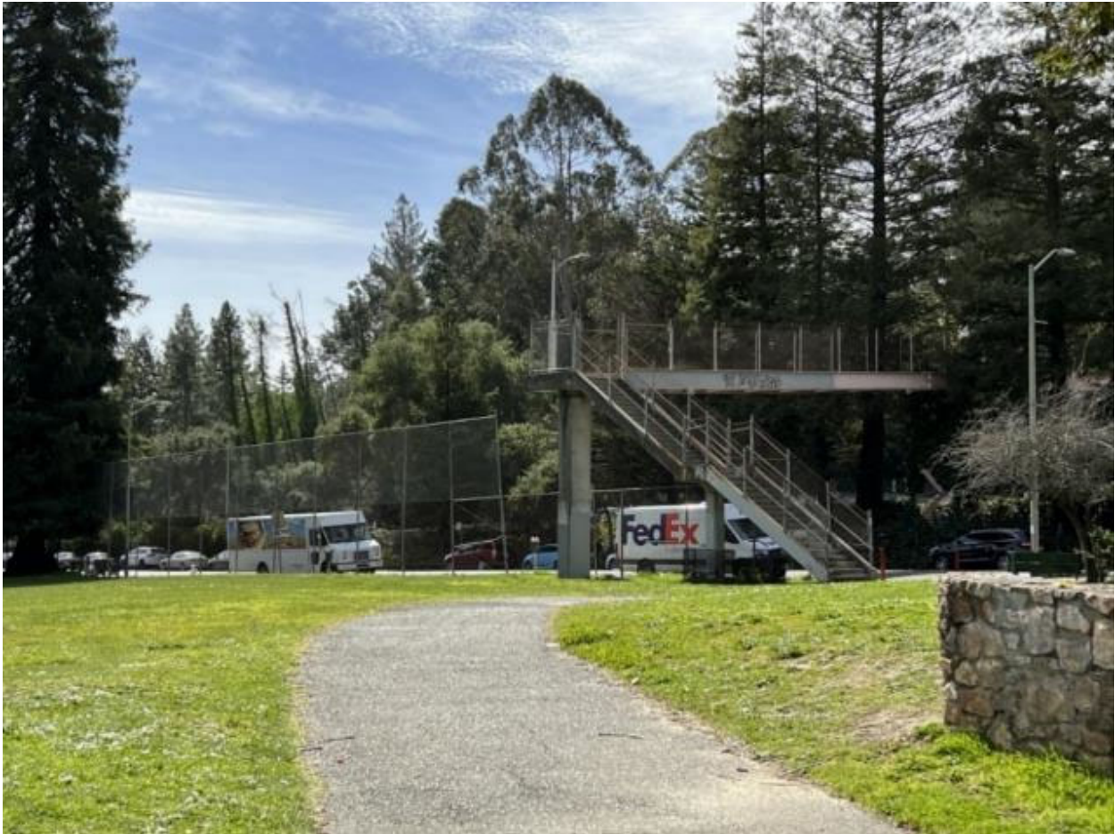
Figure 2-3. Alternative 2. Existing pedestrian overcrossing from Montclair Park Trail. View southwest.
