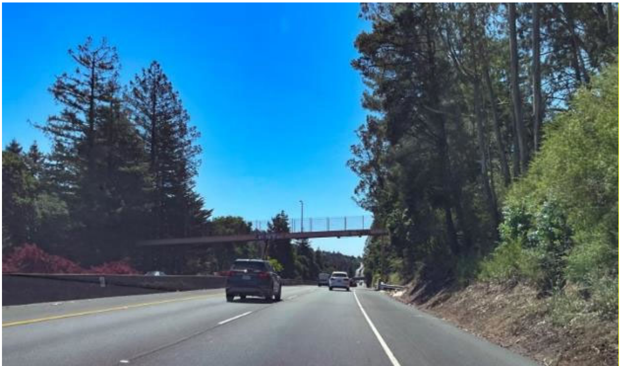
Figure 2-12. Alternative 3a/b. Existing view of pedestrian overcrossing from SR-13, southbound. View south.
