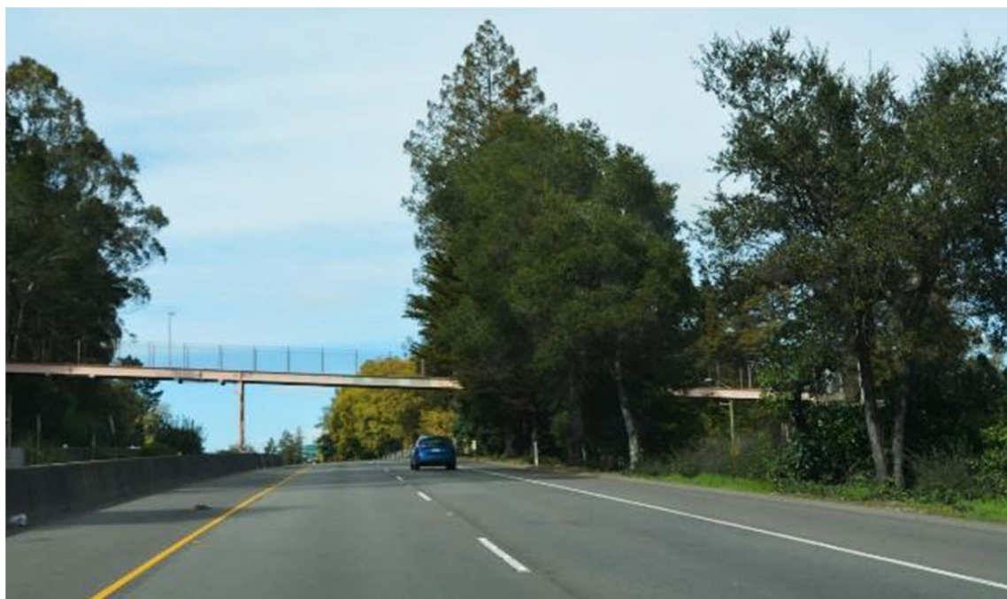
Figure 1-8. View of Existing POC from SR-13. View north.
