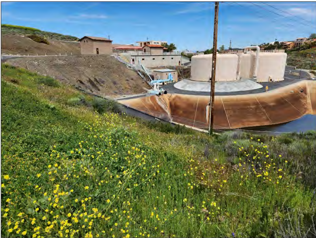
View of existing decant pond, tanks, and buildings from southern portion of site, looking north.
