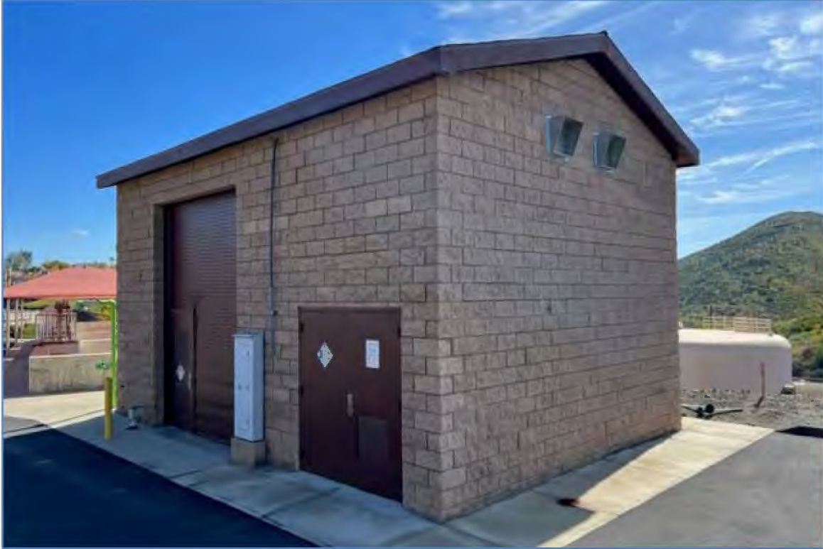
Plate 17. Chemical Feed Building 2, looking east.
