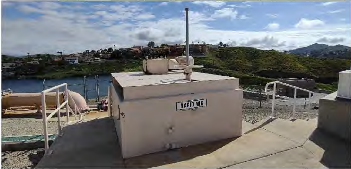
Plate 11. Rapid Mix enclosure, looking northeast.
