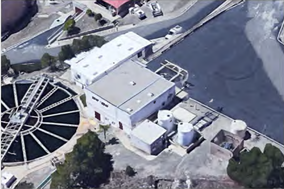
Plate 2. Aerial showing delineation of Chemical Feed Area 1 Building addition. Source: Google Earth 2023.
