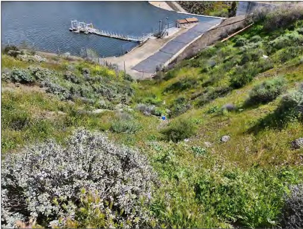
View looking north showing location of non-jurisdictional swale with dock and spillway in background. Photo taken March 27, 2023.
