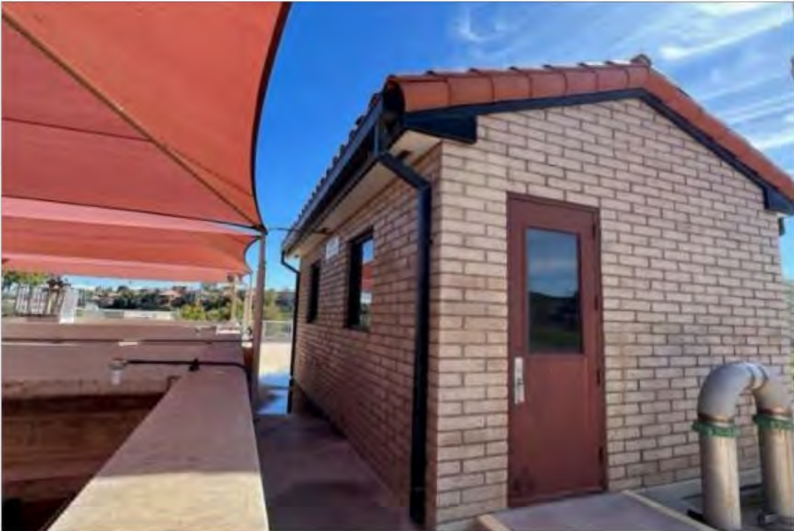
Plate 16. Containment feed structures at left, filter building at right, looking northeast.
