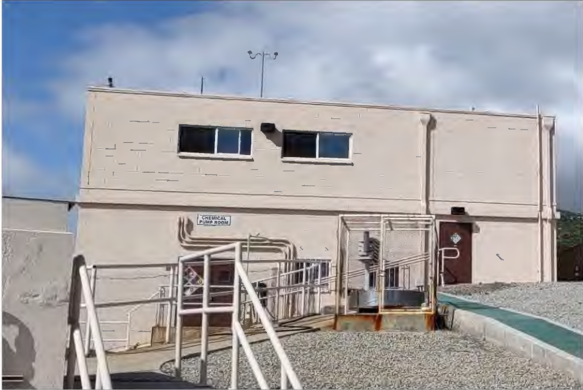
Plate 6. Chemical Feed Building 1 northeast façade showing concrete block construction, looking west.
