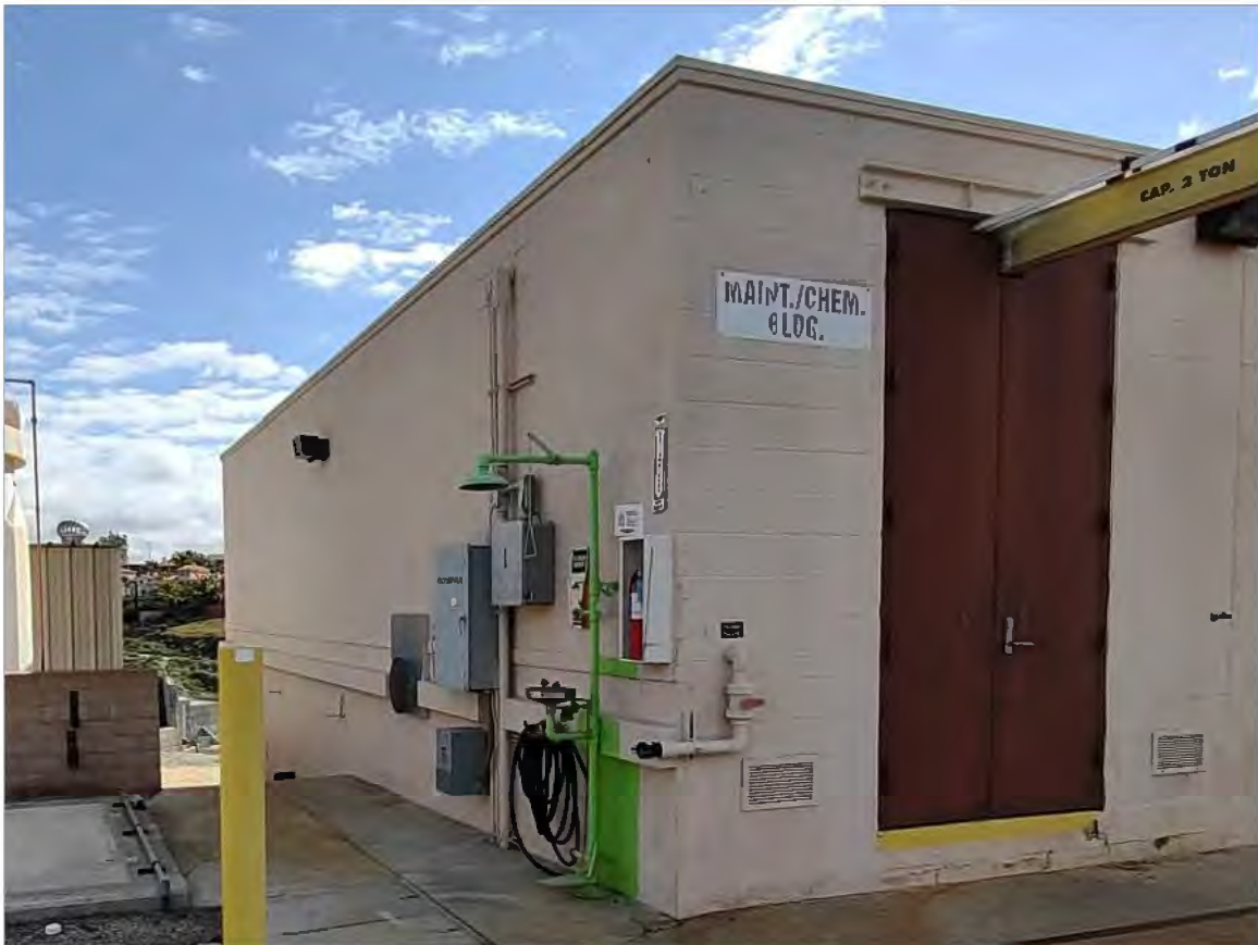
Plate 5. Chemical Feed Building 1 northwest façade, looking east.
