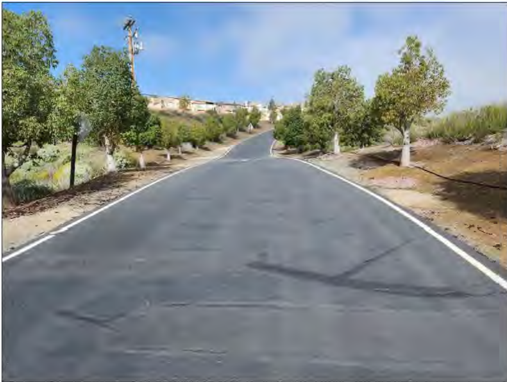
View looking northwest along entrance driveway showing ornamental trees. Photo taken March 17, 2023.
