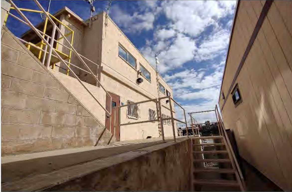
Plate 3. Chemical Feed Building 1, southeast façade, looking northeast.
