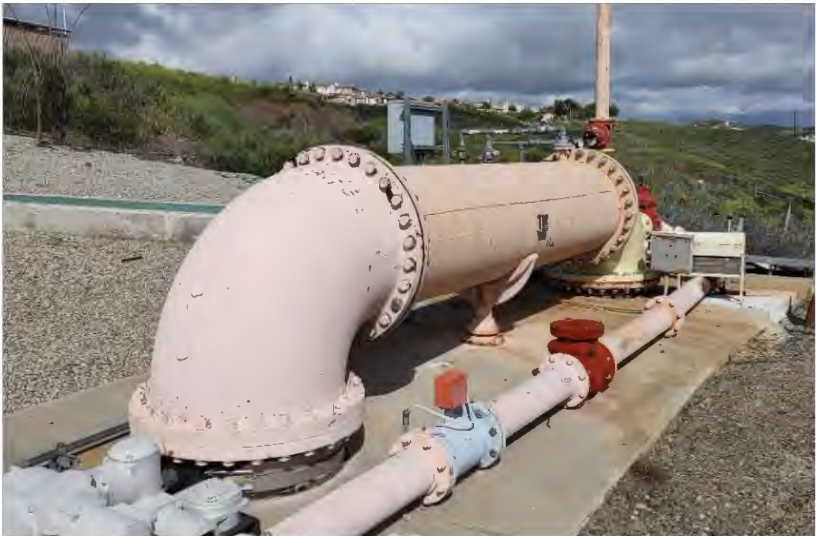
Plate 10. Static mixer (in-line), looking west.
