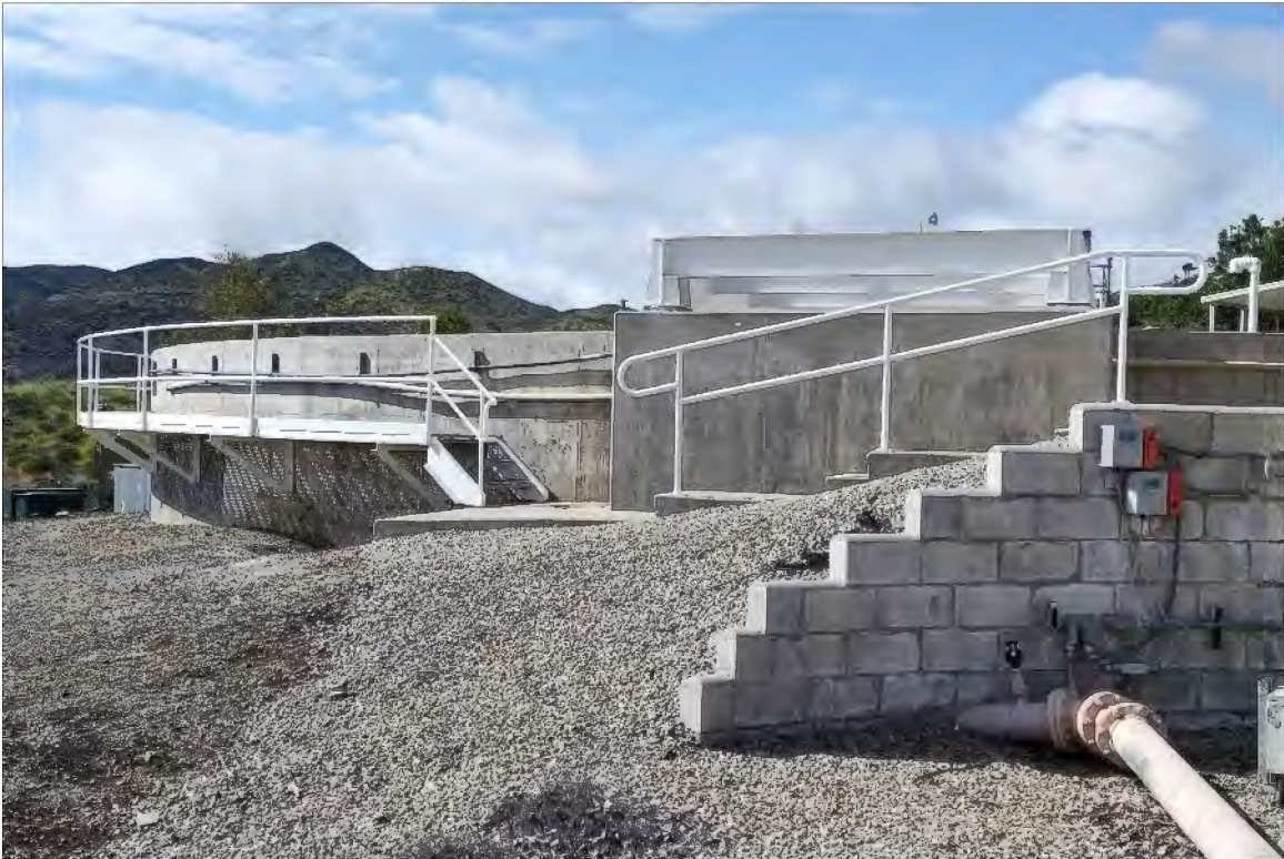
Plate 13. Exterior of concrete structure housing clarifier, looking southwest.
