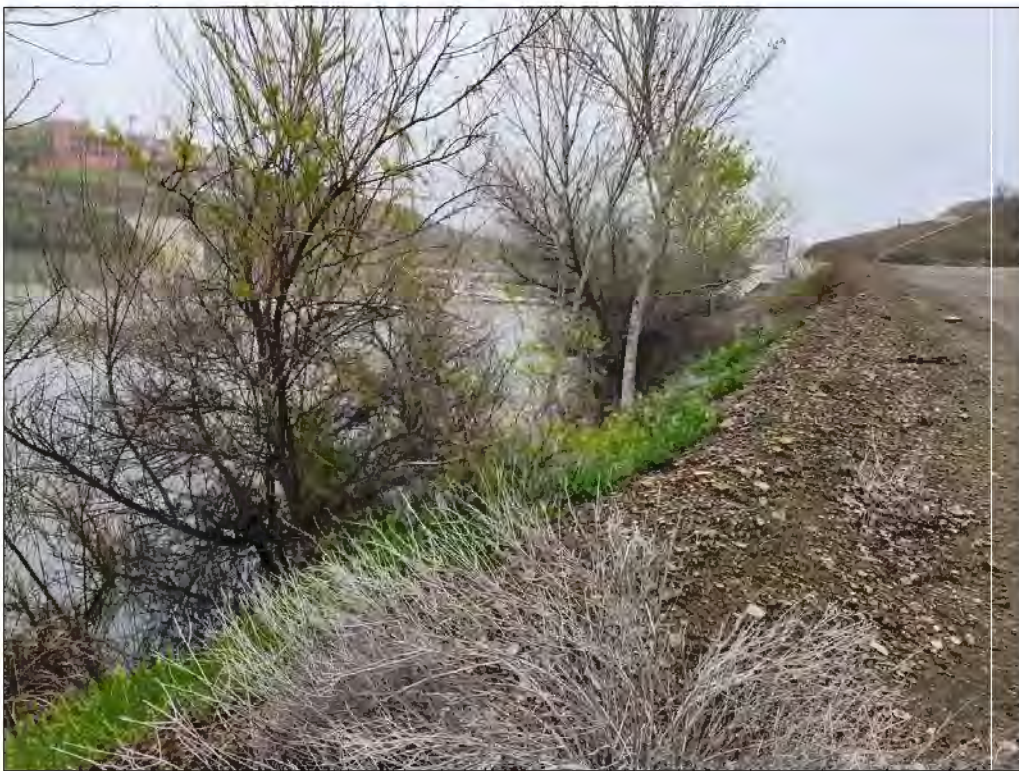
View looking north at spillway showing water level at spillway height. Photo taken May 16, 2023.
