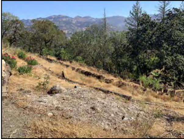
17 : Typical view of man-made retaining walls constructed with wood and old power poles.
