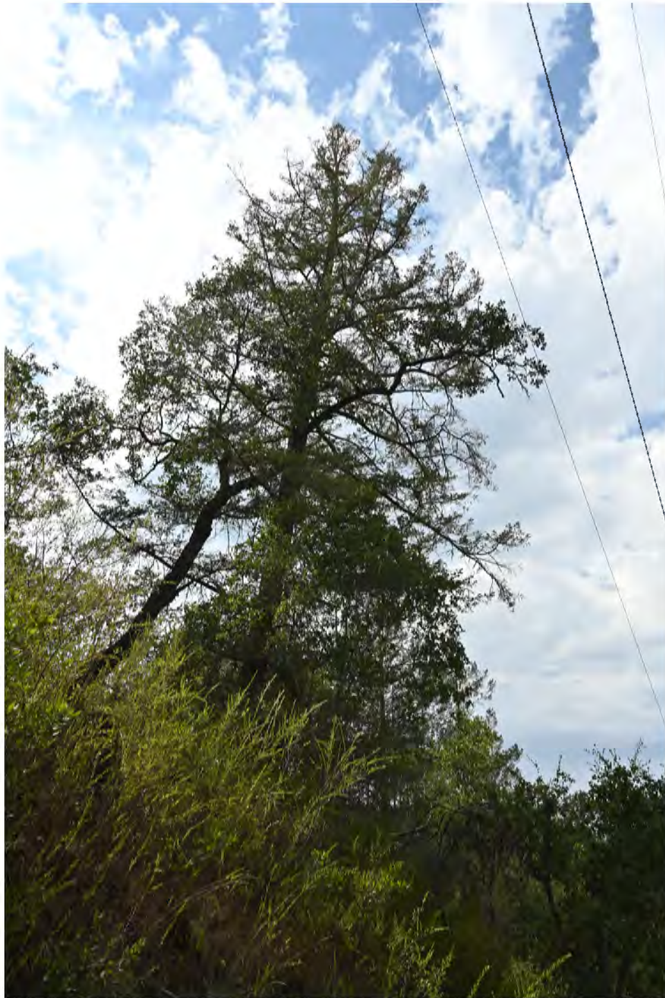
Tree #3, a Douglas fir, is in decline from boring insect attack. The tree is likely located in grading limits for road turnout.
