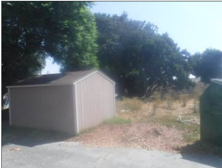
Photo 10: Smaller Storage Shed Facing East
