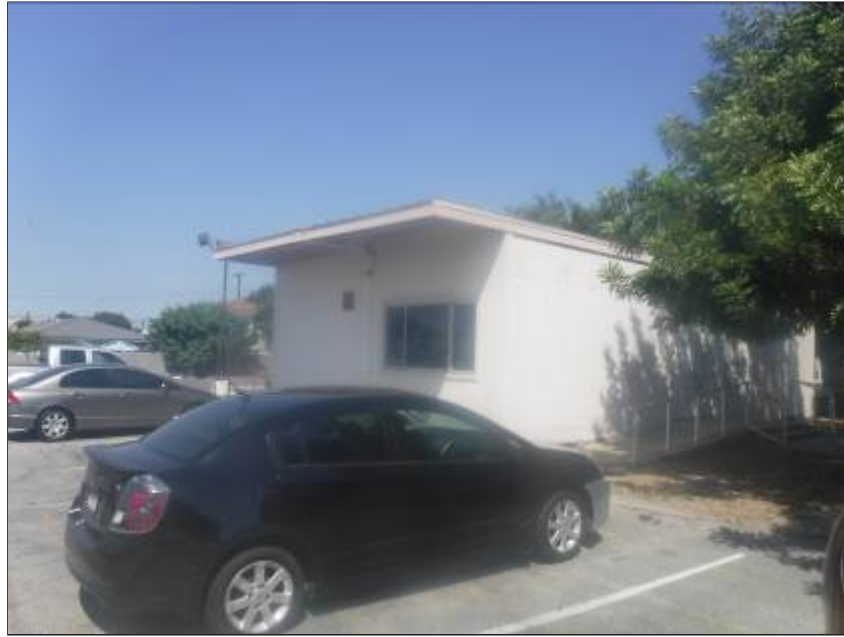
Photo 11: Classroom Bungalow on Southern portion of Site Facing Northwest
