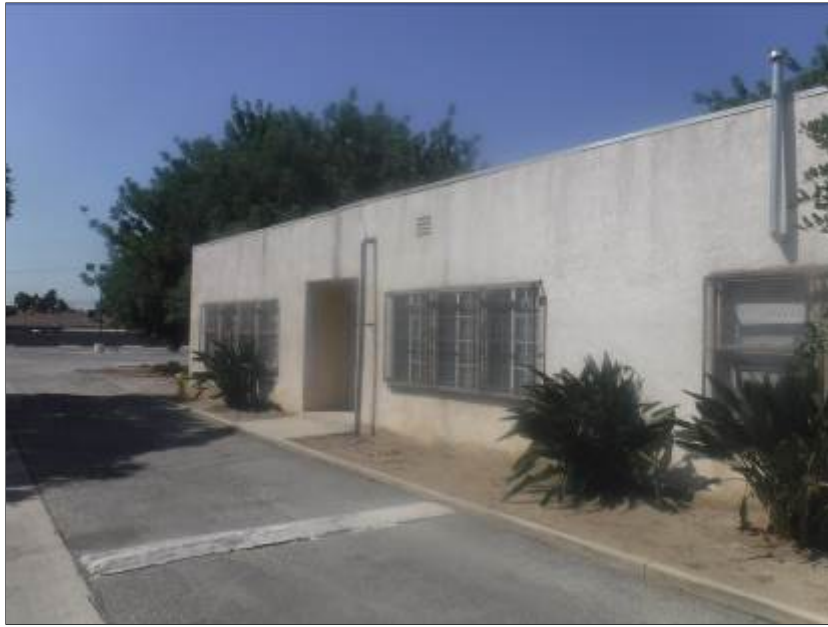
Photo 7: Classroom Building Adjoining Parking Lot Facing Southwest
