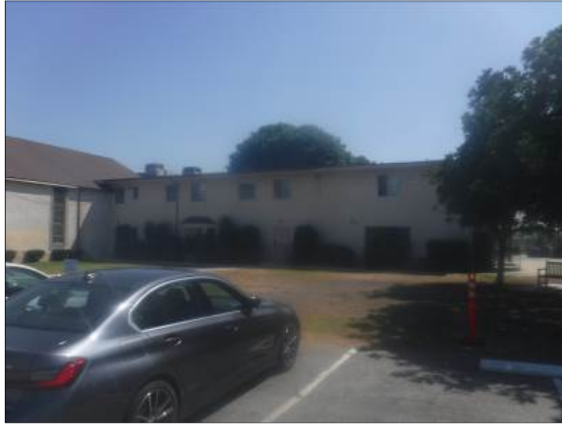
Photo 3: Church Offices connected to Chapel Facing East.
