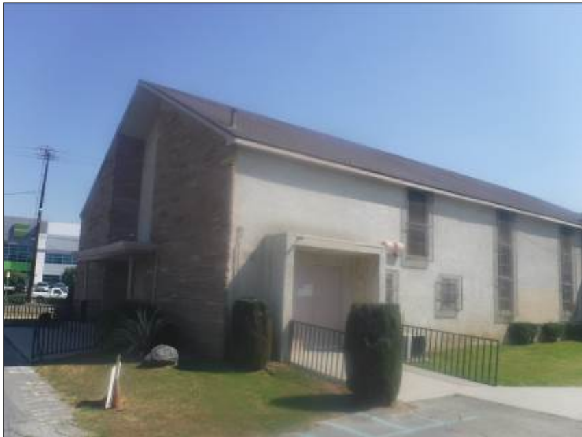
Photo 2: Chapel and Church Offices building Facing North
