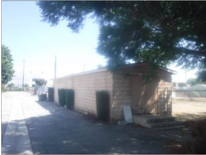
Photo 9: Storage Shed Building Facing Northeast
