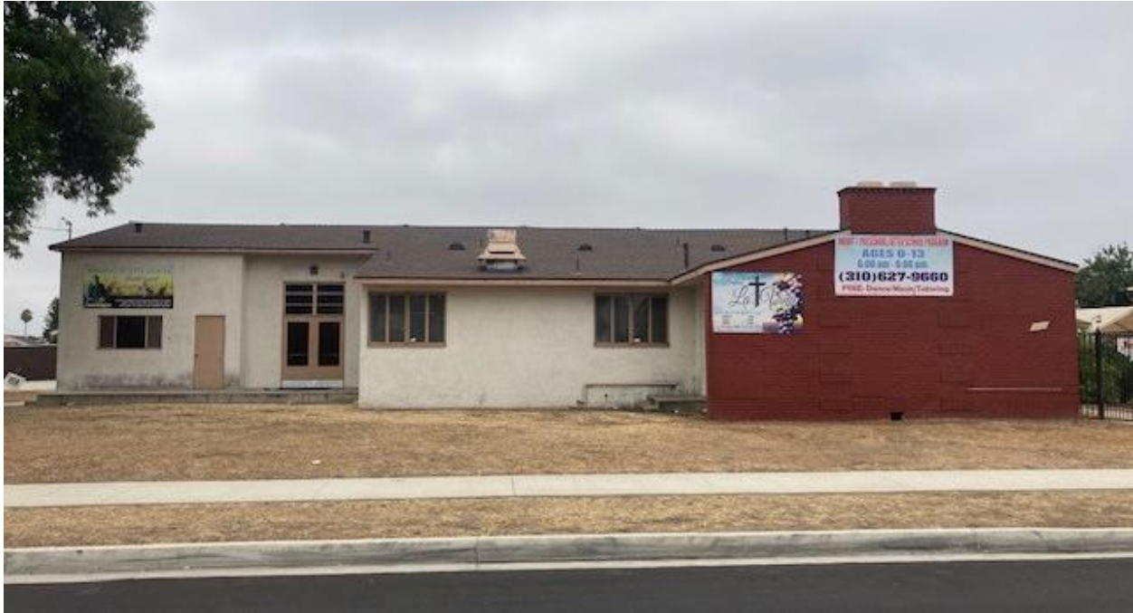
Figure 3 900 East Rosecrans North Elevation, Facing South
