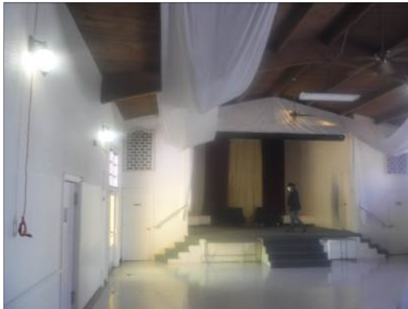
Photo 4: Interior of Fellowship Hall Building Facing East
