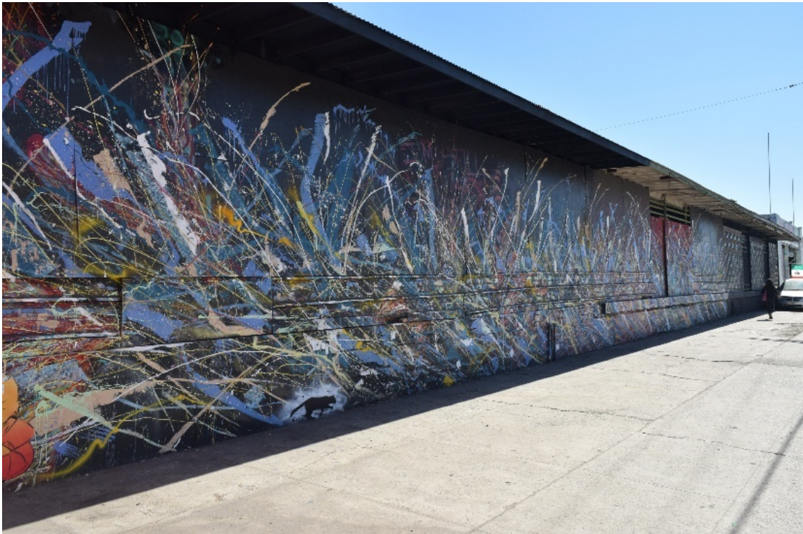
Figure 5-16. 422-430 South Alameda Street, West Elevation
