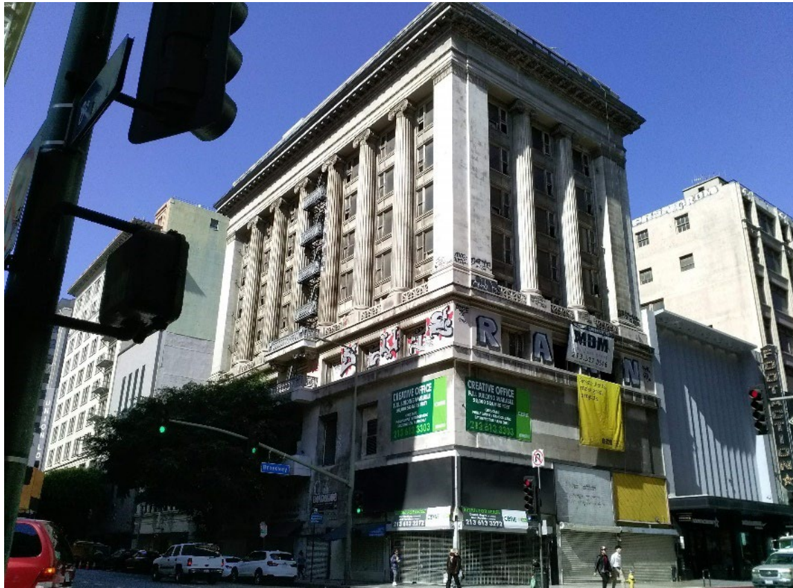
Figure 5-27. Merritt Building, South and East Elevations
