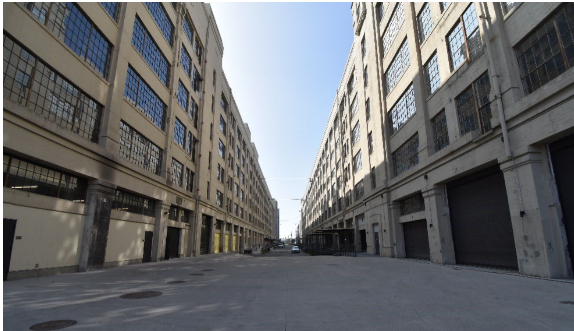
Figure 5-7. Los Angeles Union Terminal District and Buildings; Taken from the Property's Interior, North-Facing
