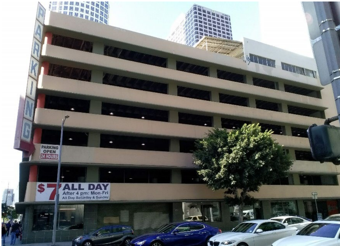
Figure 5-47. General Petroleum Corporation Parking Garage, South and East Elevations
