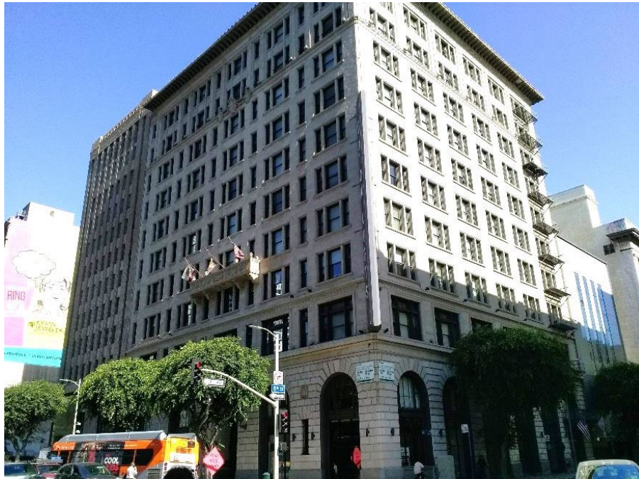
Figure 5-32. Union Bank and Trust Company Building, Primary (South and West) Elevations
