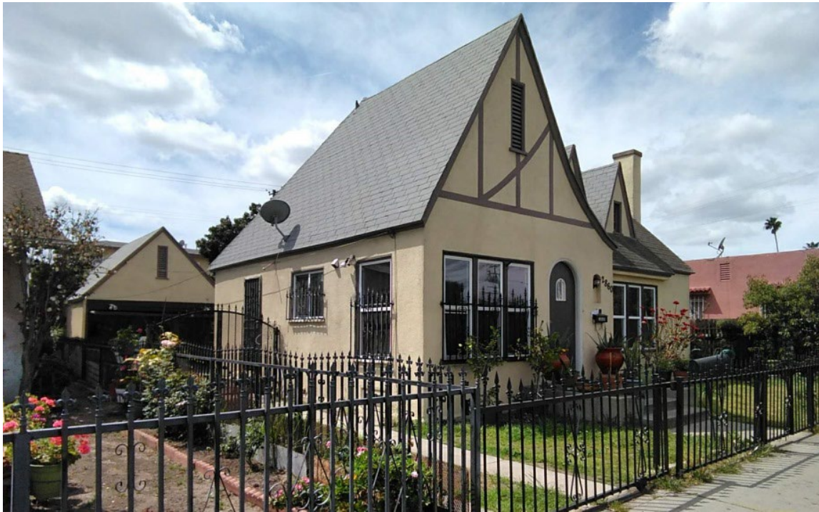
Figure 5-84. 2860 Randolph Street Primary (North) and East Elevations
