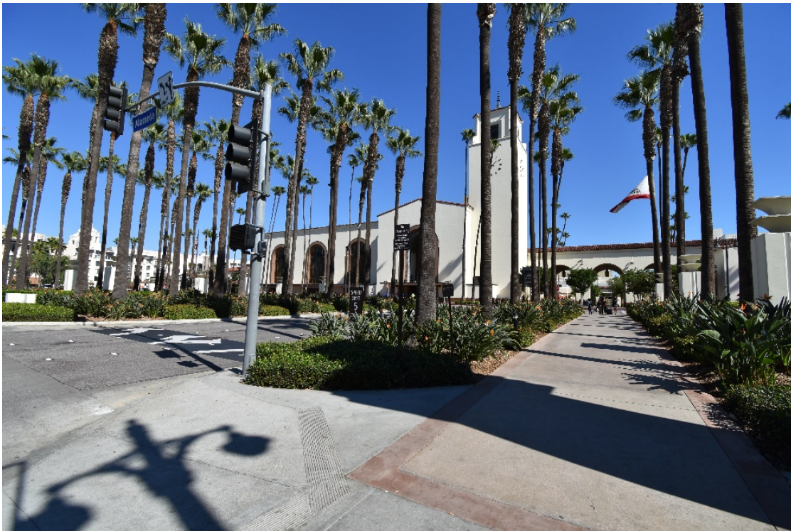
Figure 5-1. Los Angeles Union Station, West Elevation of Terminal Building
