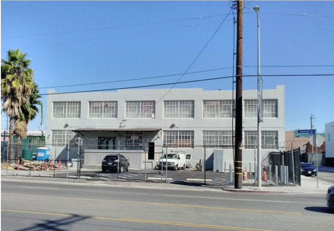
Figure 5-19. 542 South Alameda Street, Primary (West) Elevation
