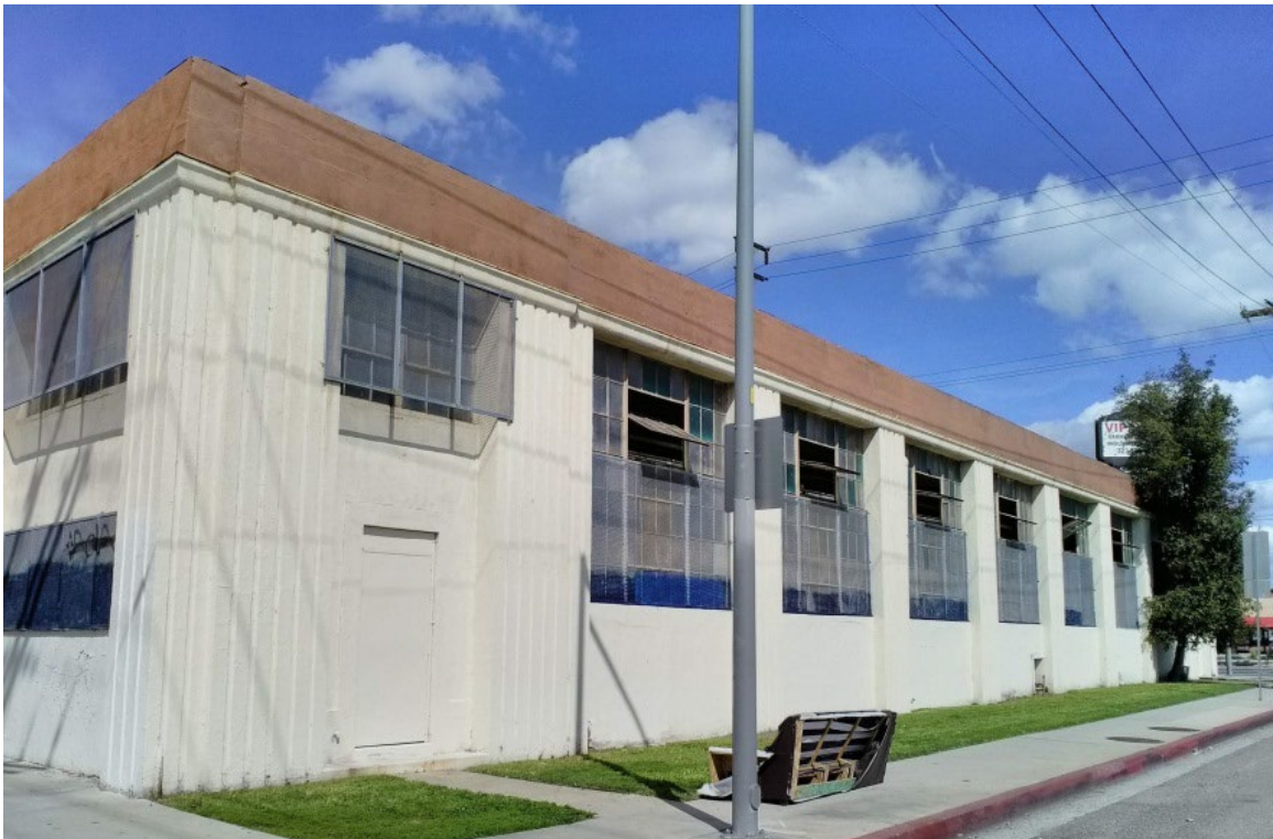
Figure 5-82. 6101 Santa Fe Avenue
