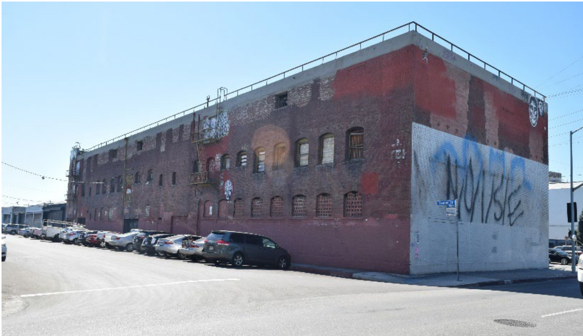
Figure 5-15. 400 South Alameda Street, North and East Elevations
