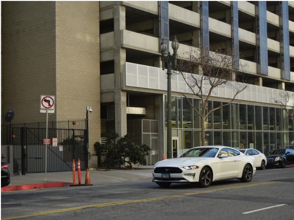
Figure 5-55. South Hope Street Streetlights, East side of Hope Street, South-Facing
