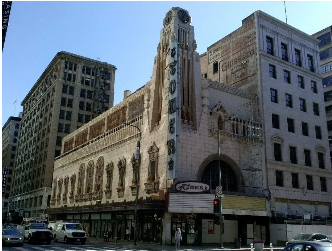
Figure 5-29. 800 South Broadway, North and West (Primary) Elevations
