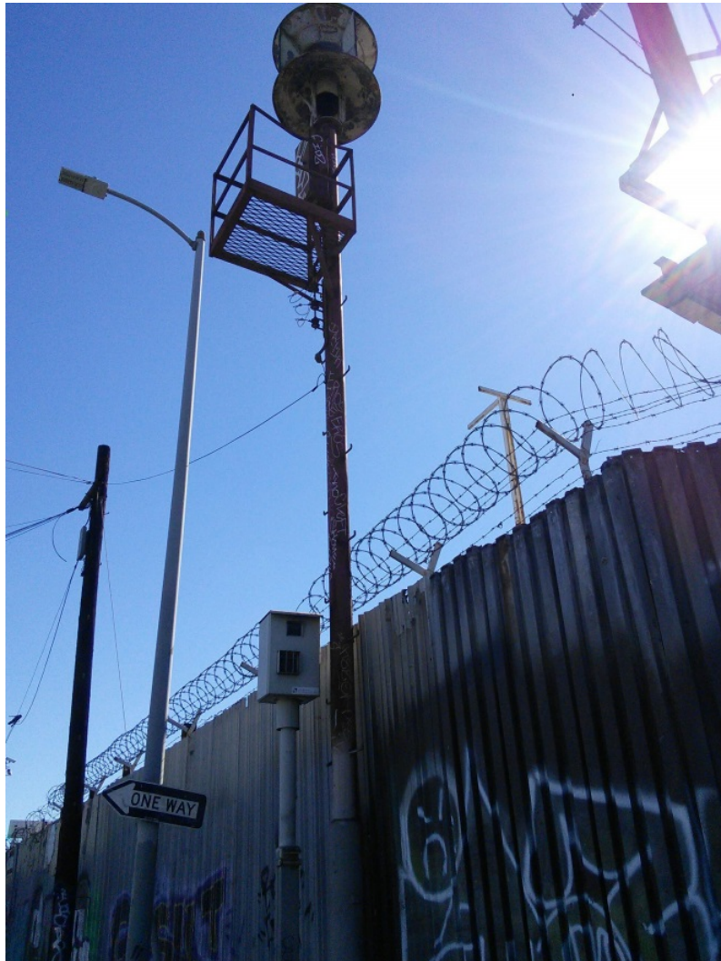
Figure 5-57. Air Raid Siren No. 70, South-Facing
