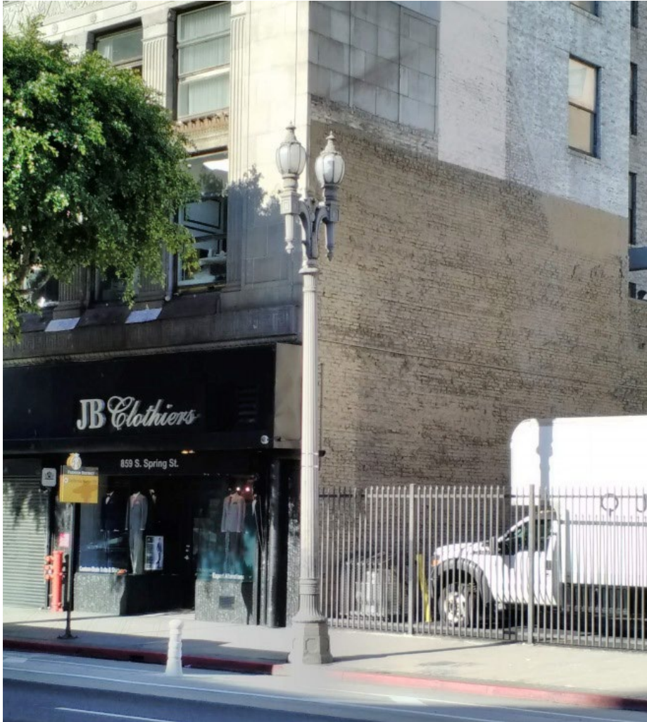
Figure 5-56. South Main Street Streetlights; West side of Main Street, Southwest-Facing
