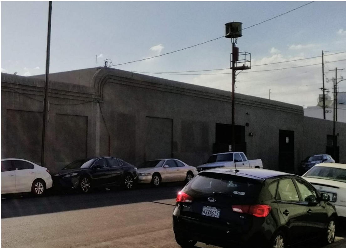
Figure 5-53. Air Raid Siren No. 65, View from the North
