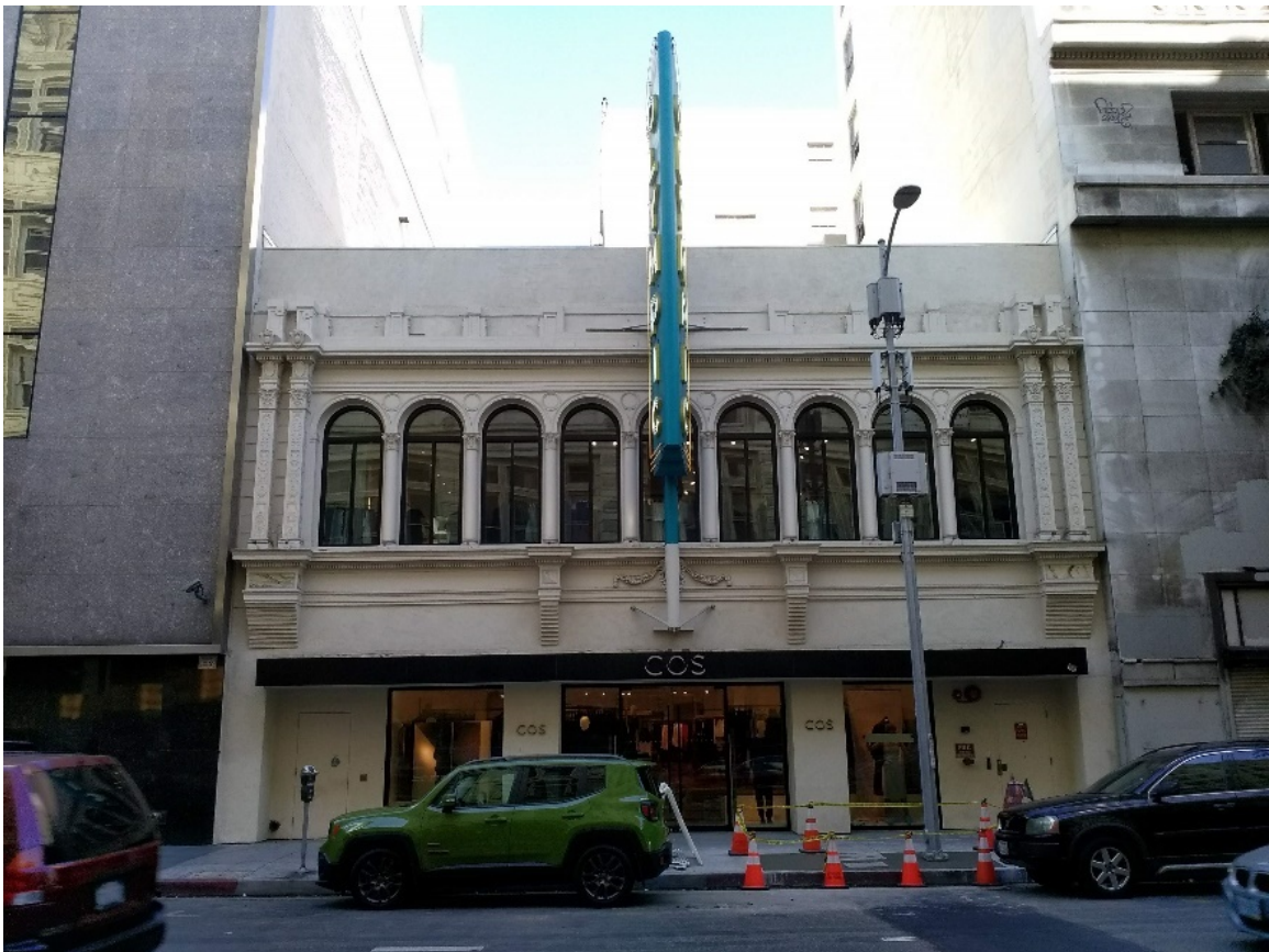
Figure 5-48. The Olympic Theater, Primary (South) Elevation
