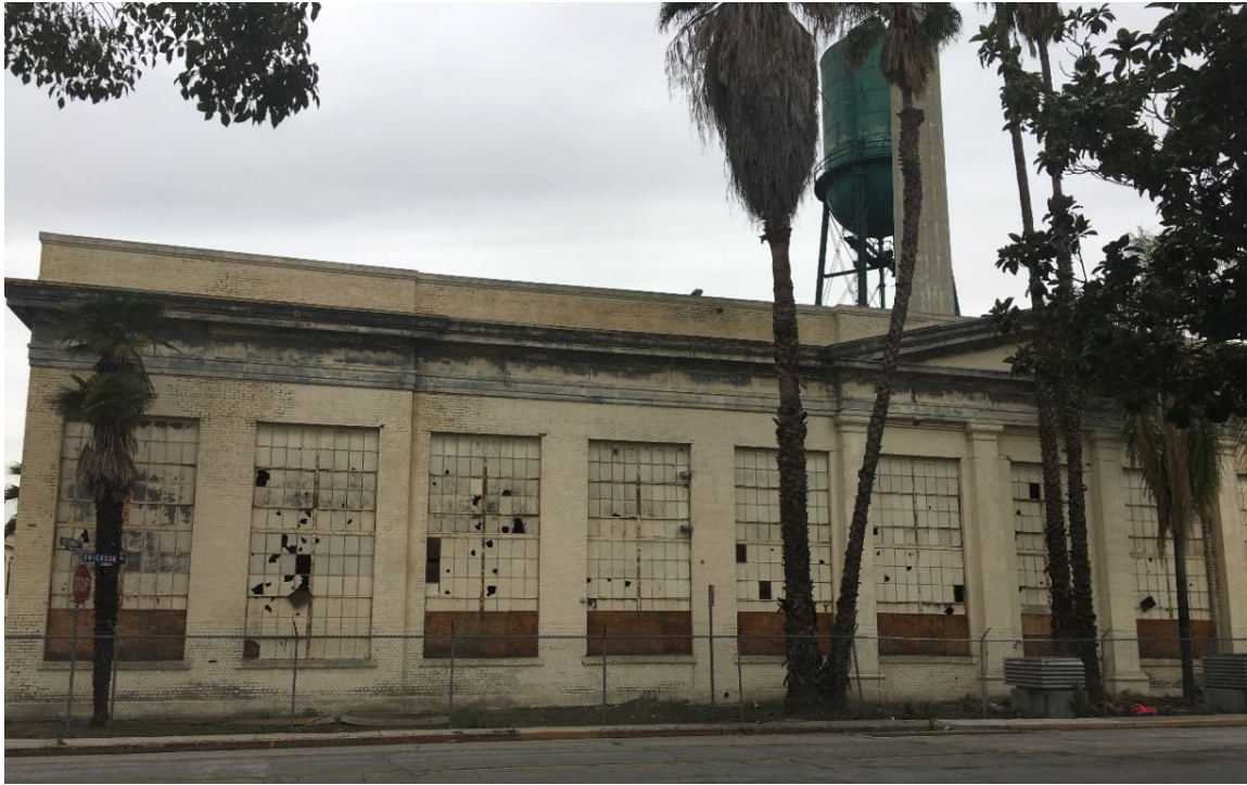
Figure 5-69. Rancho Los Amigos Medical Center Historic District; Taken from Interior of Property, Northwest-Facing
