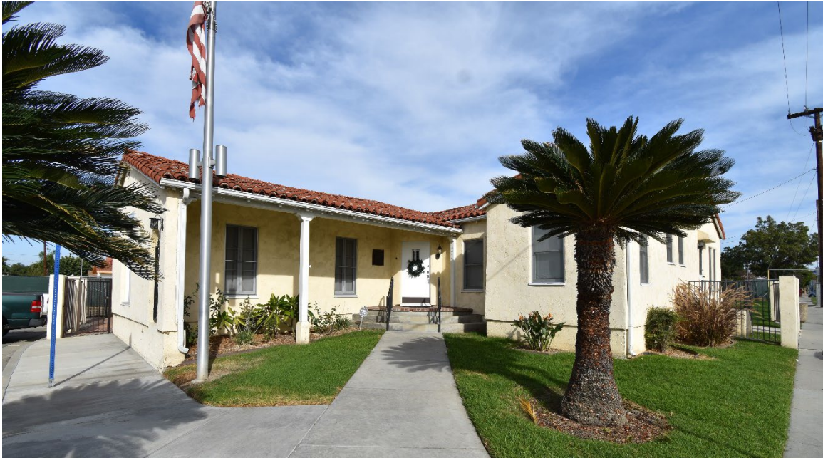
Figure 5-87. Primary Building at 81644 Albutis Avenue; South and West Elevation
