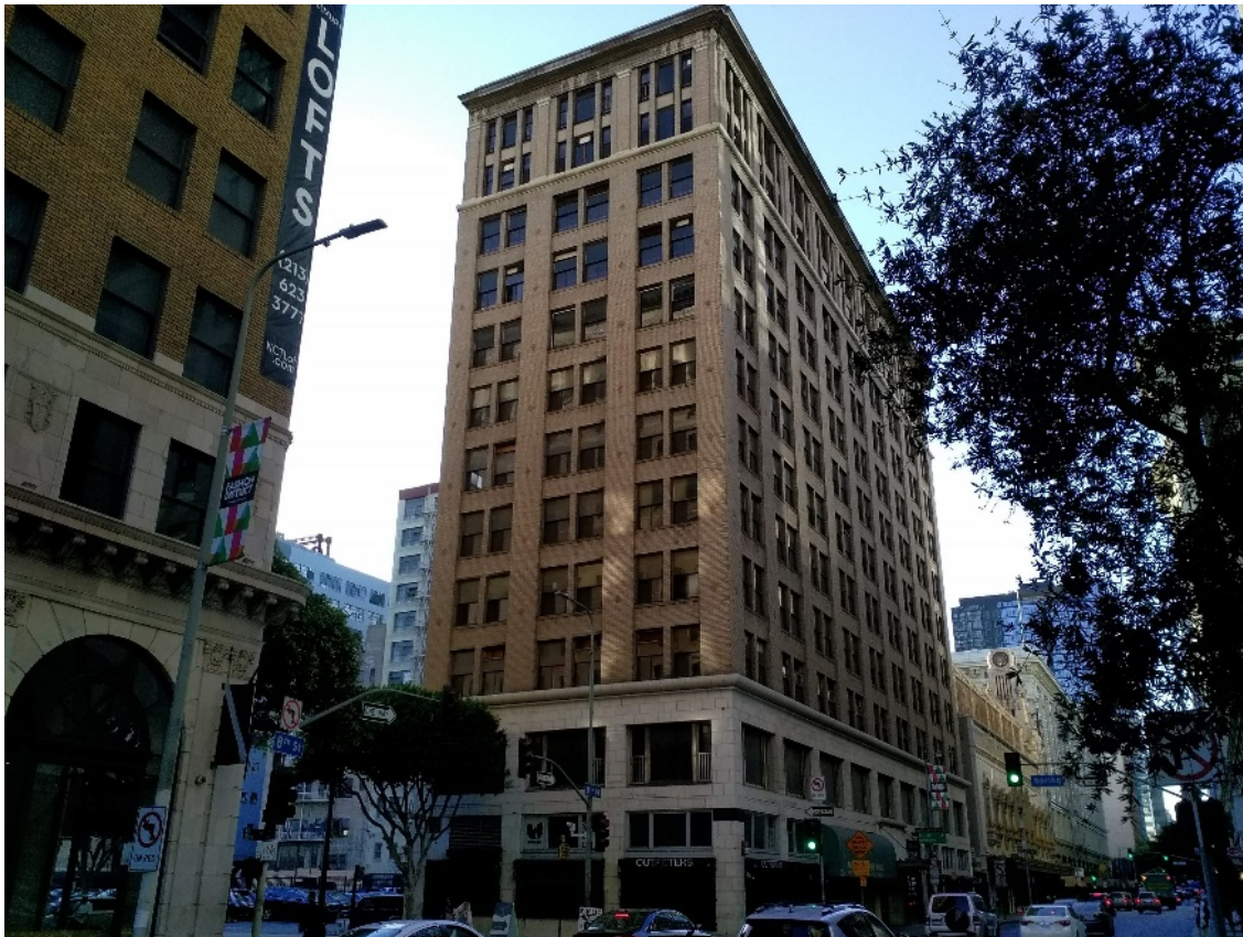
Figure 5-45. 801 South Spring Street, Primary (North and East) Elevations
