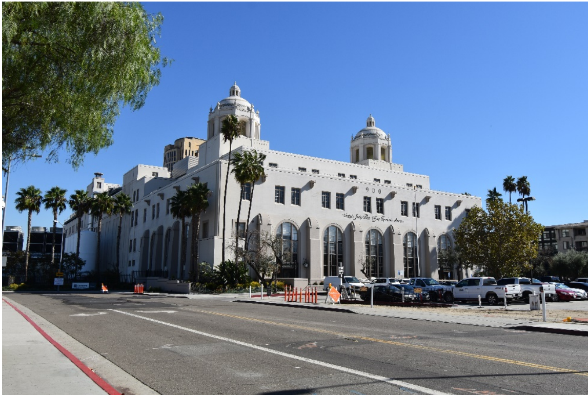
Figure 5-6. Los Angeles Terminal Annex Post Office, South and West Elevations
