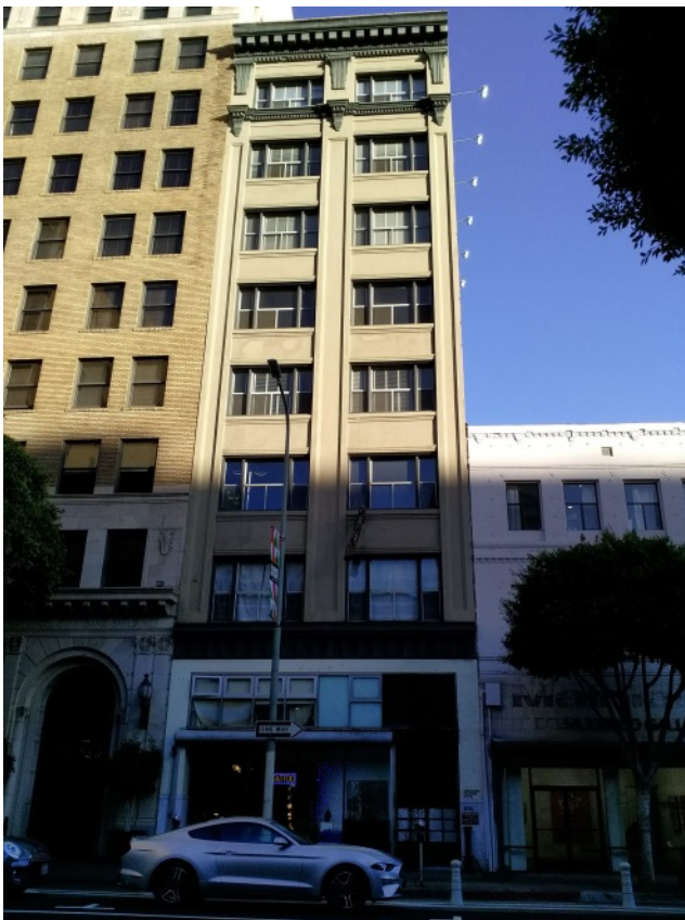
Figure 5-37. Gans Brothers Building, East Elevation
