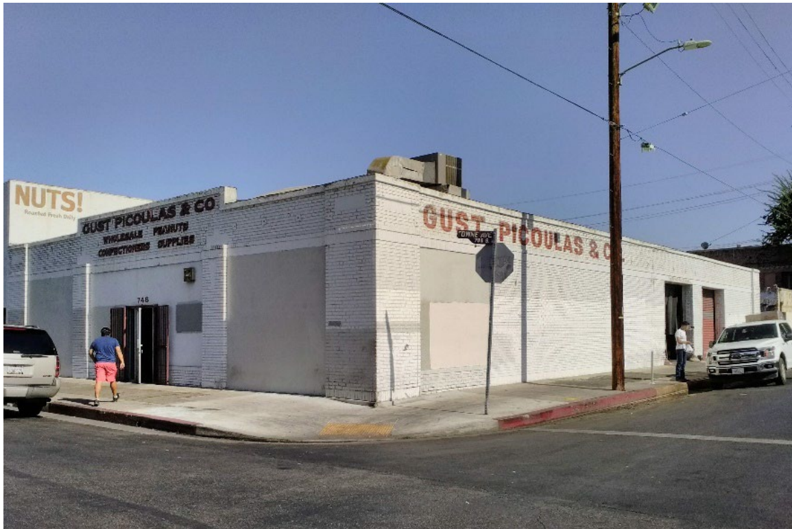
Figure 5-54. 740-746 Towne Avenue; Southern Building, Primary (West) and South Elevations
