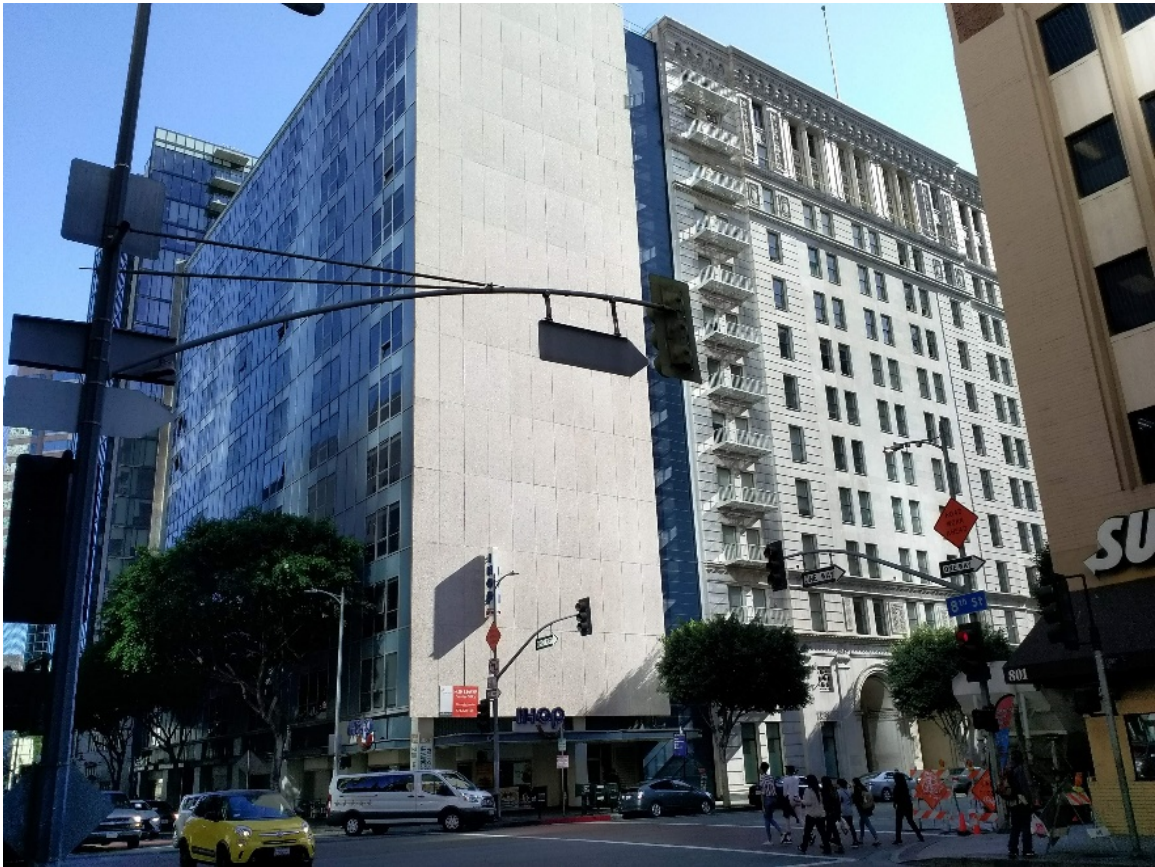
Figure 5-36. SoCal. Gas Complex, View from the North
