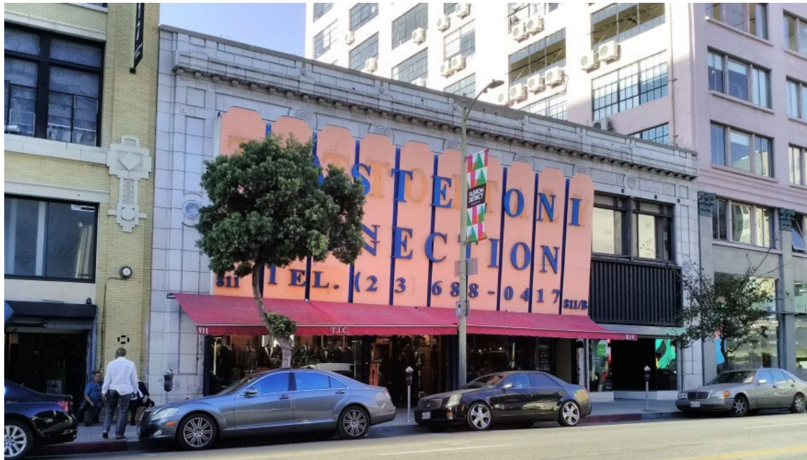
Figure 5-44. 809 South Los Angeles Street, East Elevation
