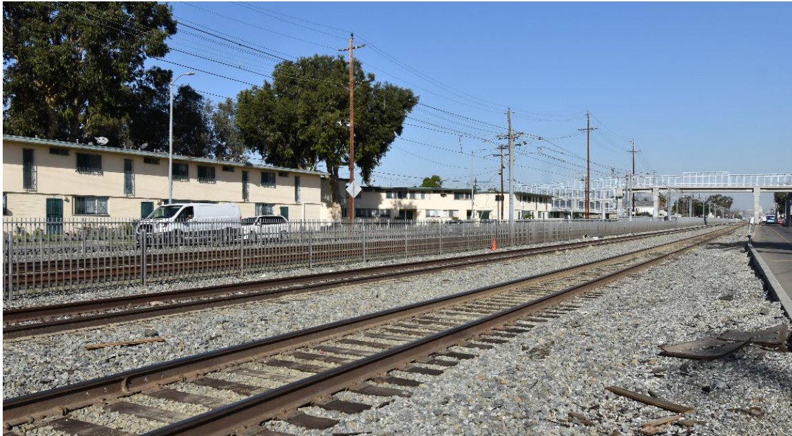
Figure 5-61. Pueblo Del Rio Public Housing Complex Historic District in Relationship to Existing Rail ROW; Existing 53rd Street Pedestrian Bridge in Background at Right; Southwest-Facing
