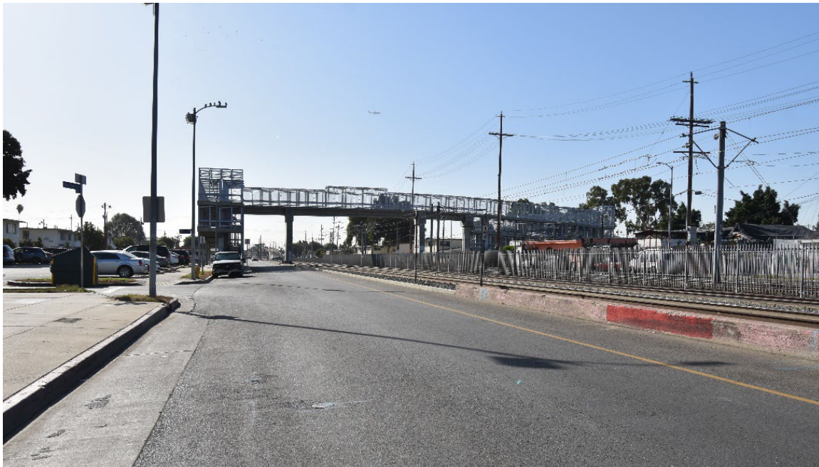
Figure 5-62. Existing 53rd Street Pedestrian Bridge Northeast-Facing
