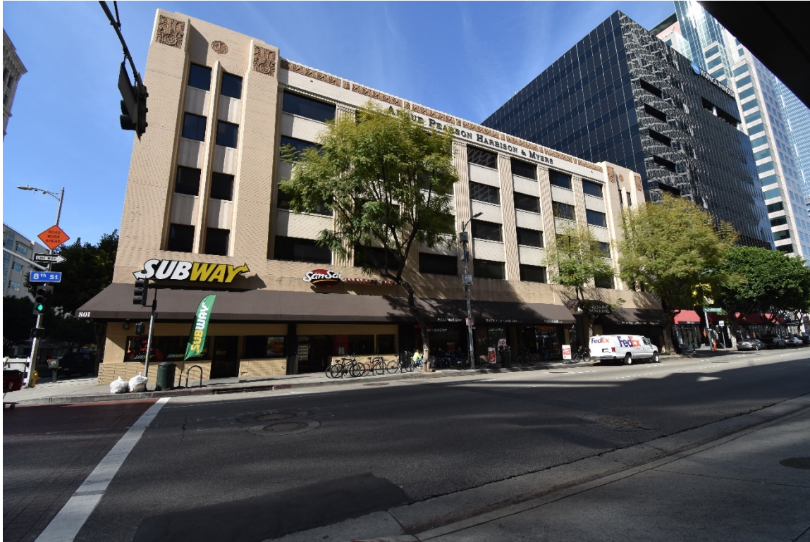
Figure 5-41. 801 South Flower Street, North Elevation
