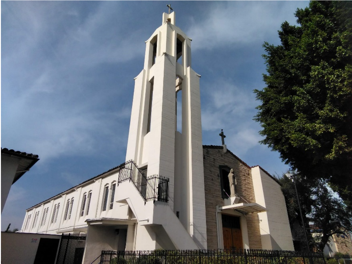
Figure 5-79. Our Lady of the Rosary Church Building, Primary (East) and South Elevations
