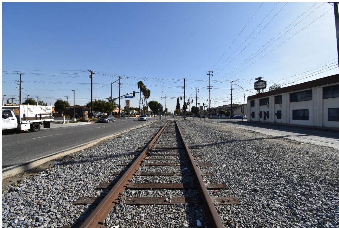
Figure 5-83. View of 6101 Santa Fe Avenue and its Current Surroundings and Relationship to the ROW
