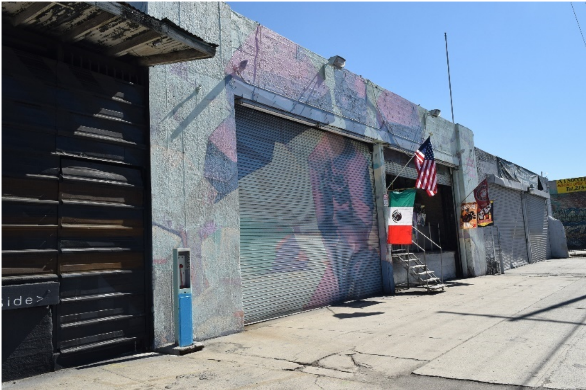
Figure 5-17. 436 South Alameda Street, West Elevation
