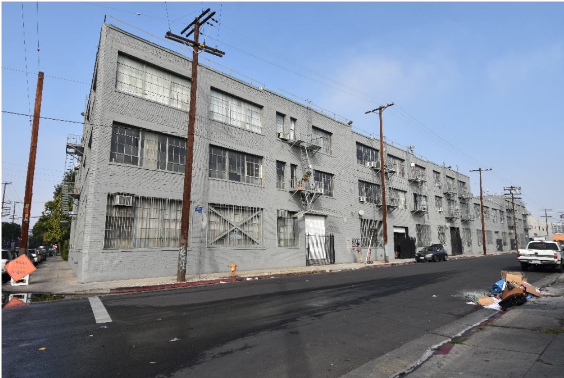
Figure 5-21. 1250 Long Beach Avenue, East Elevation
