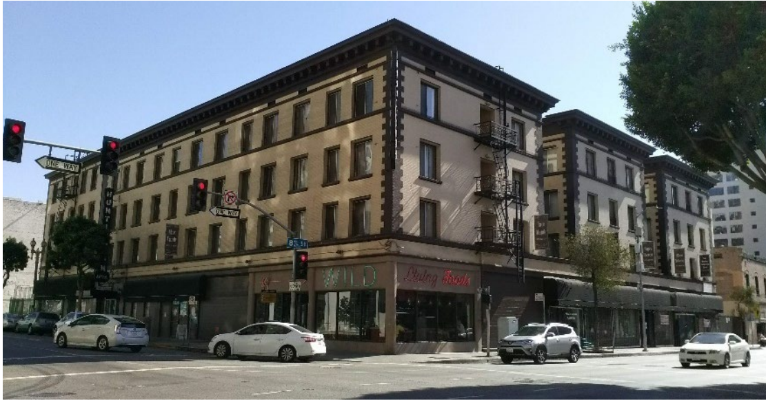
Figure 5-42. 752 South Main Street, South and West Elevations
