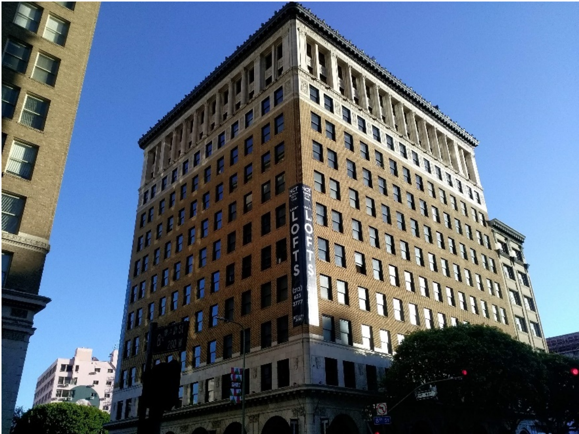
Figure 5-46. National City Bank Building, Primary (North and West) Elevations
