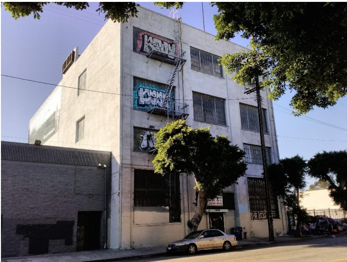
Figure 5-9. 1608 East 15th Street, North Elevation
