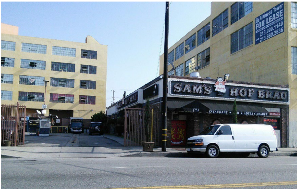
Figure 5-24. 1731 East Olympic Boulevard, Primary Elevation
