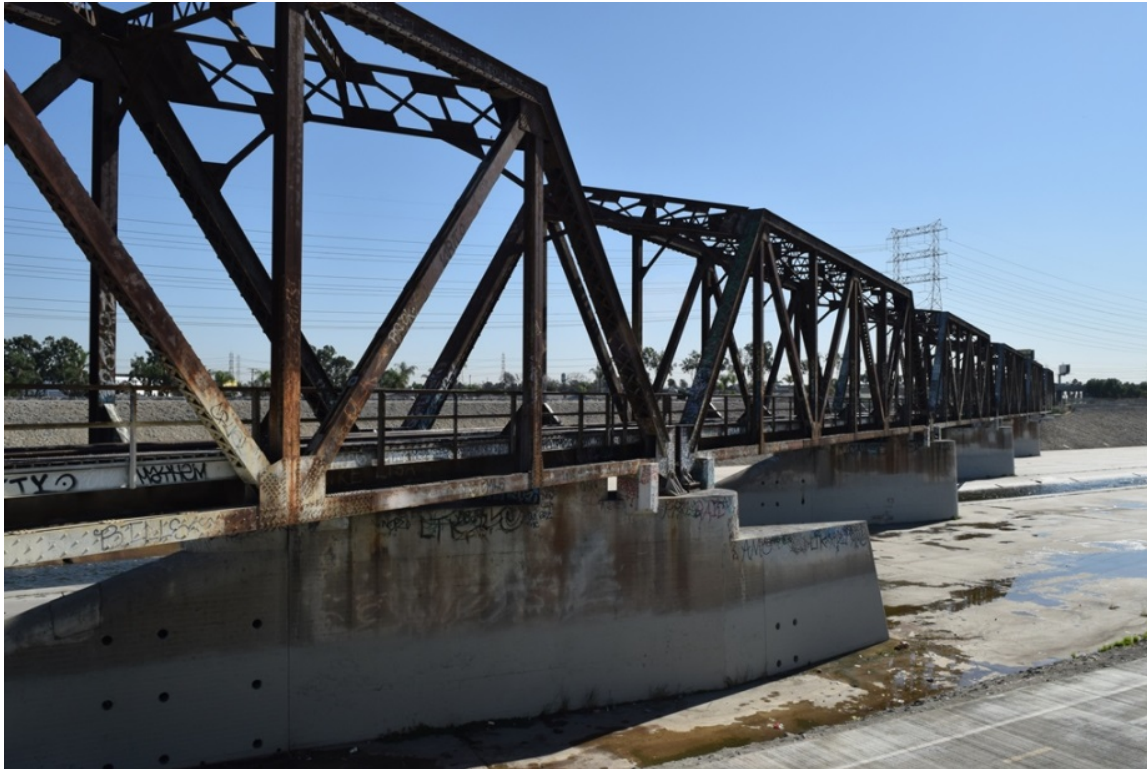
Figure 5-78. Union Pacific Los Angeles River Bridge Taken from the North Side of the Rio Hondo, South-Facing
