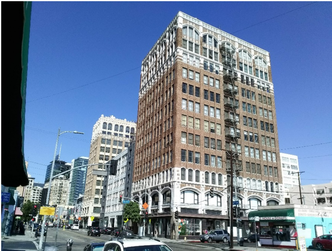
Figure 5-35. Textile Center Building, South and East Elevations
