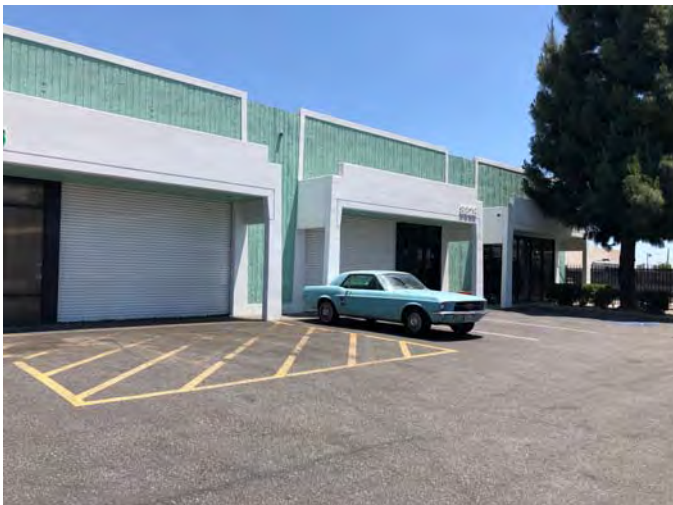
Figure 4. View of Building 2, West Elevation
