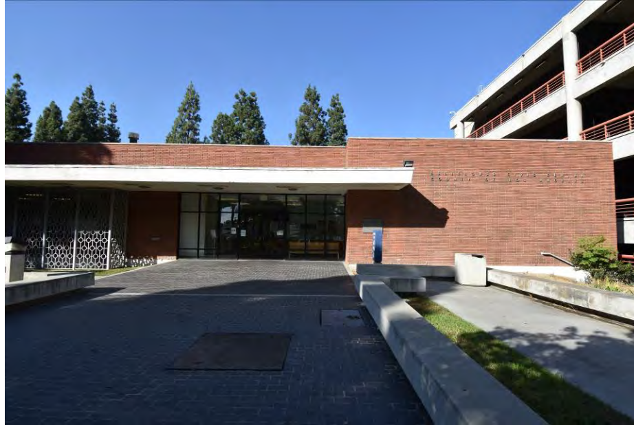
Primary Elevation of Heath Center Building; north-facing
