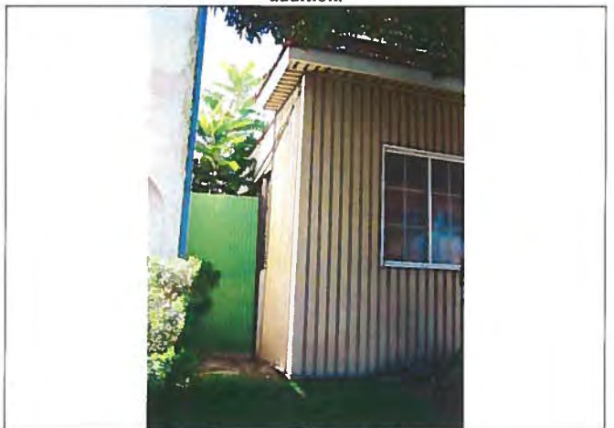
View looking southeast at the north elevation.
