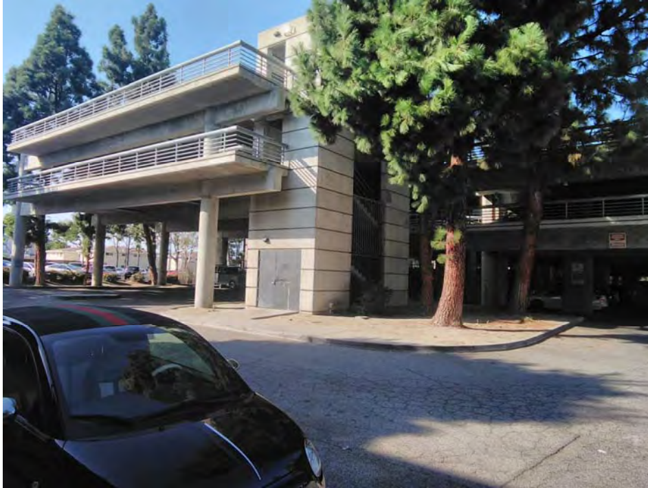
Parking Structure, view to the northwest
