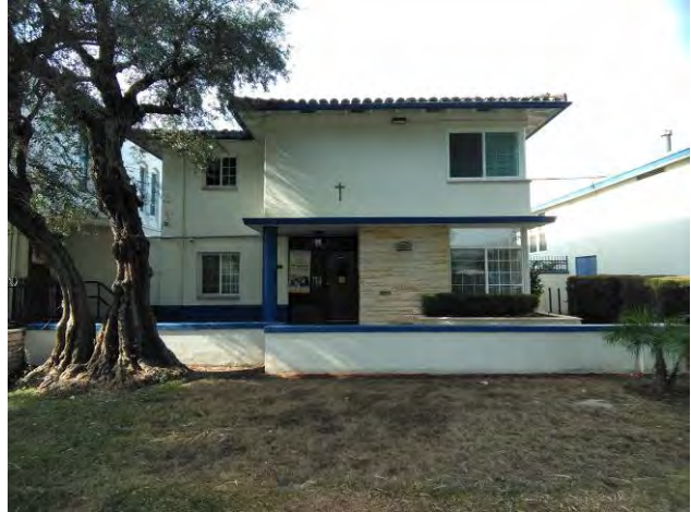
Rectory building, eastern façade, view west.
