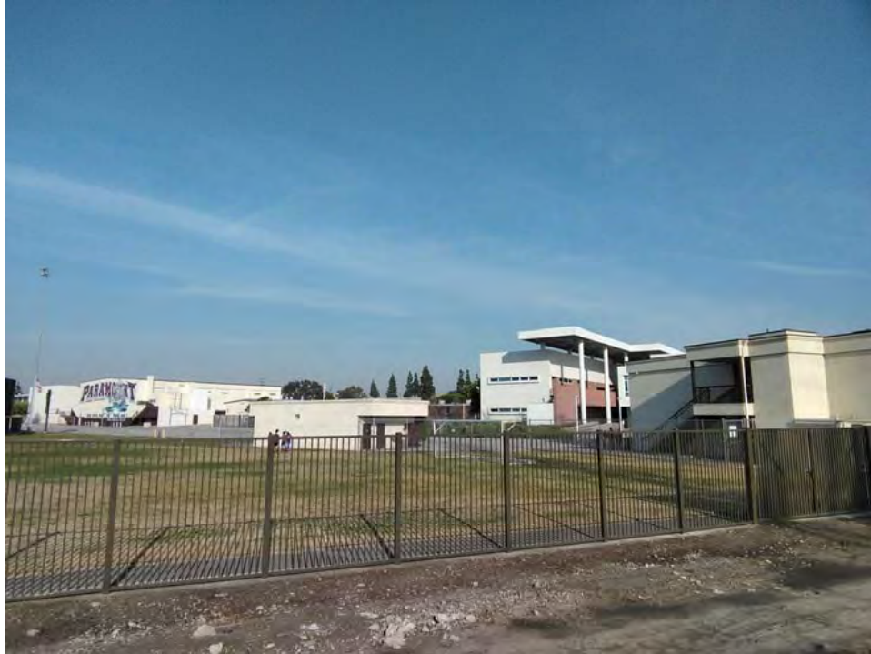
Photograph 2. Overview of south end of PHS West Campus: (left to right): Gymnasium, restroom, Medical Health and Science Building, classroom building. Camera facing northeast.
