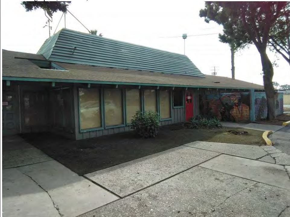
Photograph 2. Building 2, north elevation, camera facing southwest.
