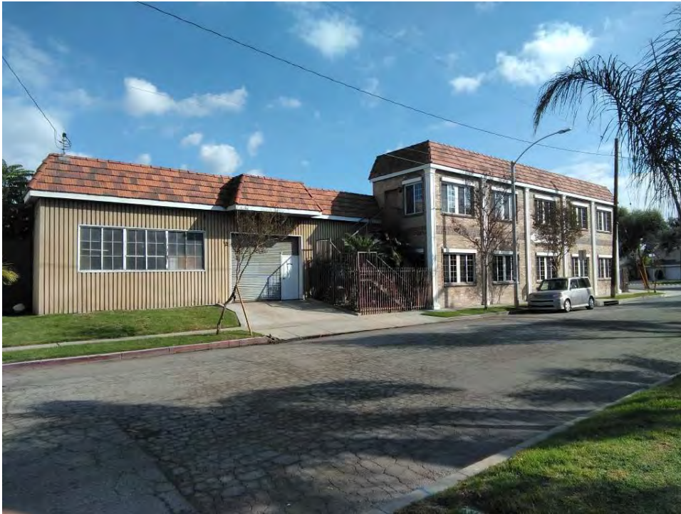
12508 Center Street, west elevation. Camera facing southeast.
