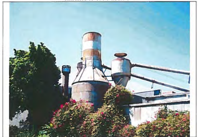
View looking southwest at 1957 sawdust collector (center) and circa 1970s incinerator (left).
