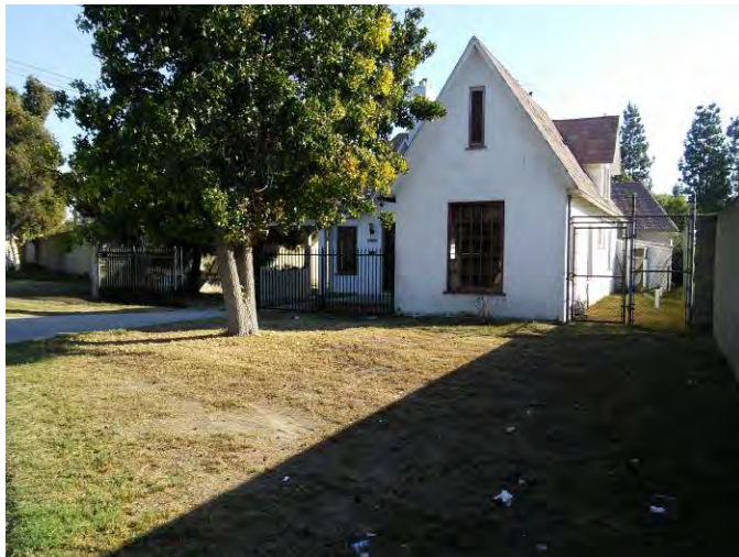
Northern façade, view to the south.
