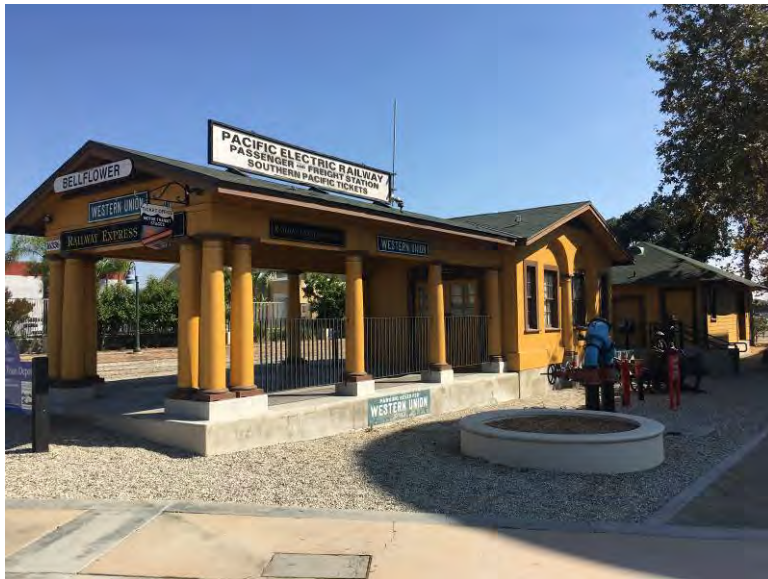
Bellflower Railroad Depot west and south elevations, view to the northeast.
