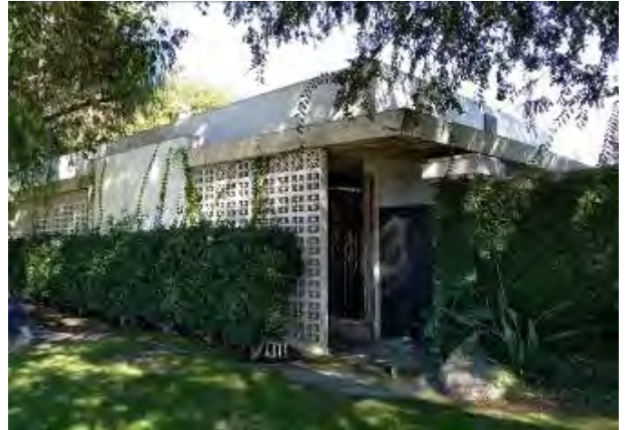
Southwest corner of building at 14632 Downey Ave, view to NE.
