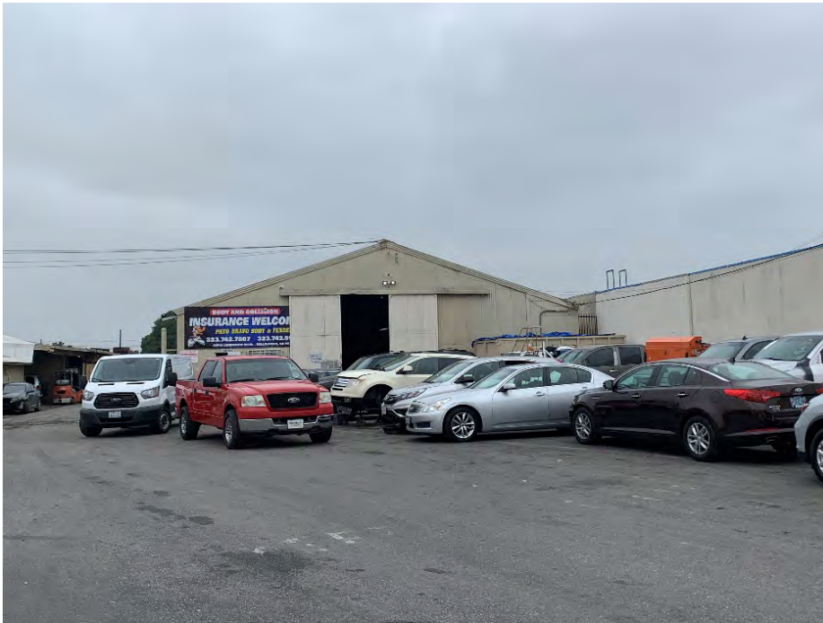
West Façade of Southern-most Building on Property
