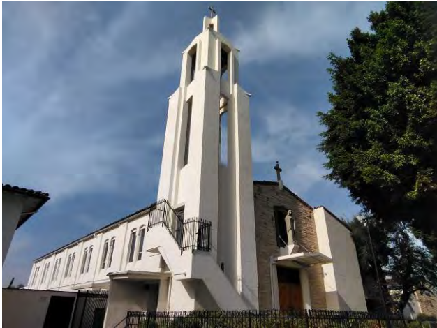
Church, eastern façade, view northwest.
