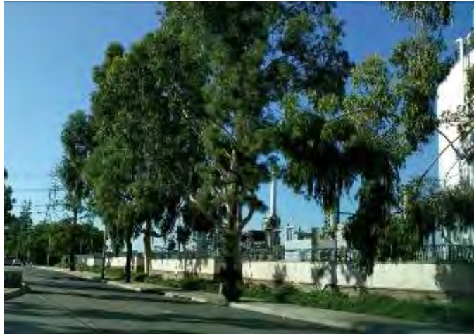
View of refinery from Somerset Blvd., view to the NW.
