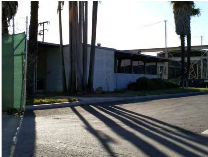
Office building, north elevation, view to the southwest, 11/14/2018.
