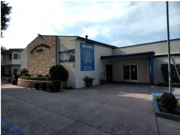
School building at NE corner of property, view southwest.
