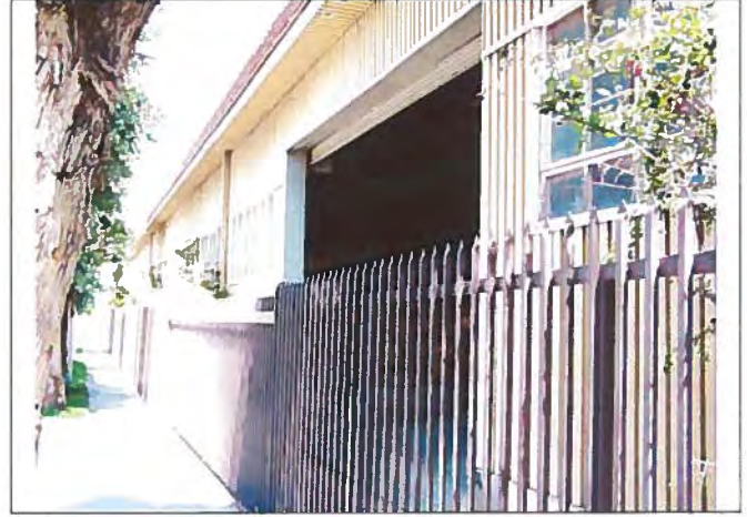
View looking northwest at the south facing entrance to the 1946 elevation addition.
