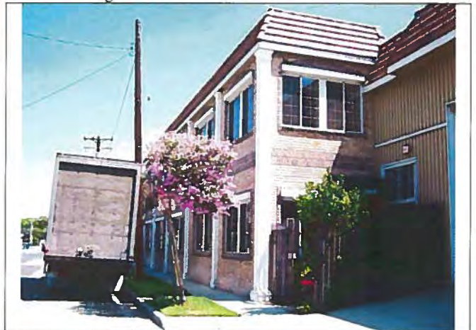
View looking northeast at the west elevation of 1991 office addition.
