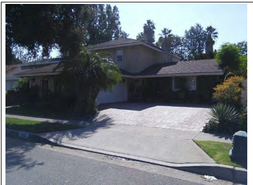
P5b. Description of Photo: Northeastern façade, view to the south, Nov. 2018.
