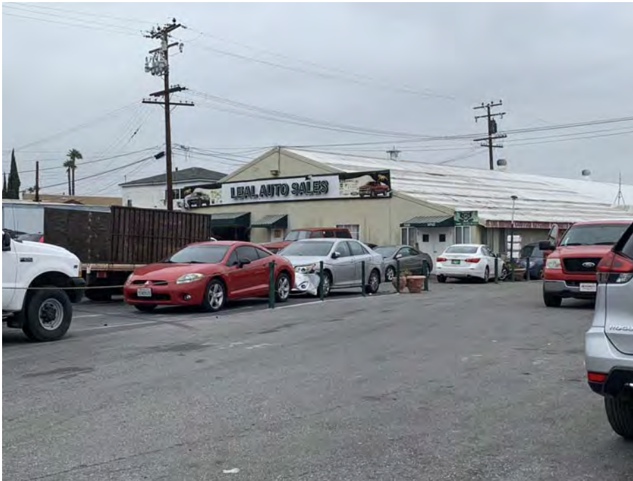
West and south elevations of Northern-most Building on Property
