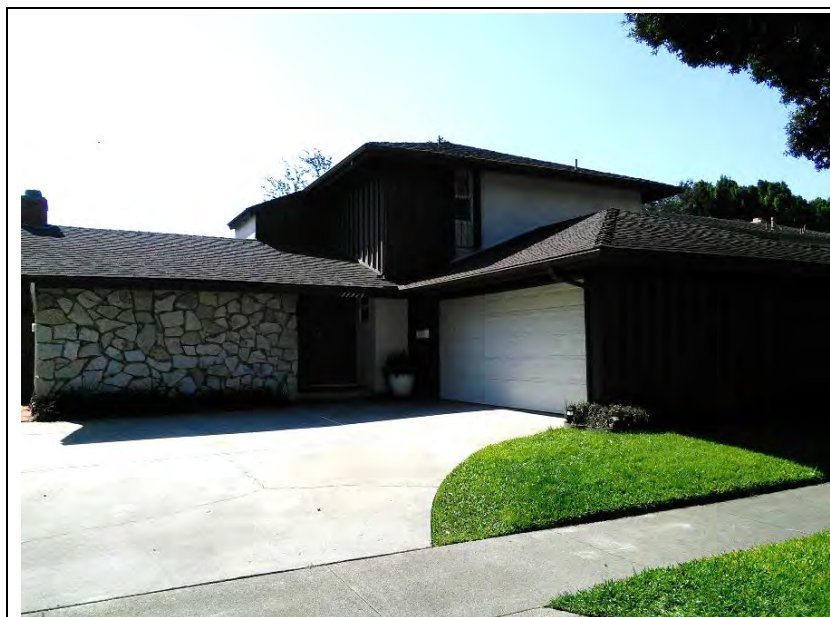
P5b. Description of Photo: Northeastern façade, view to the south.
