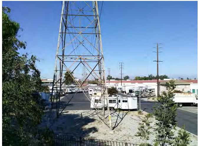
RV storage and SCE equipment on APN 7034-001-803, view north
