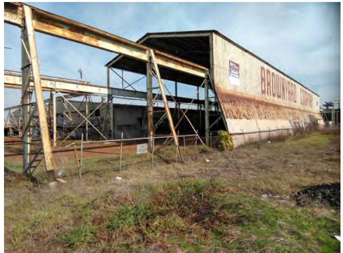
Large shed at southern edge of property, view to northeast, 1/16/2018.
