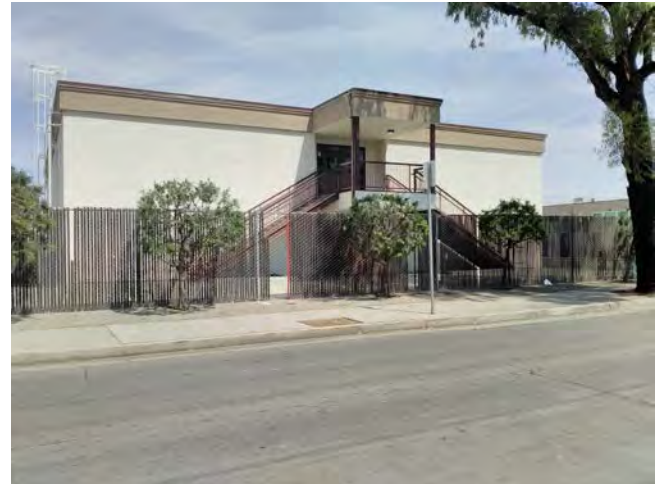
Paramount Park High School West Auditorium Building (Building #15), South Elevation; North-facing
