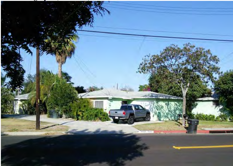
Photograph 2. Overview of cottages on Flora Vista Street. Camera facing north.
