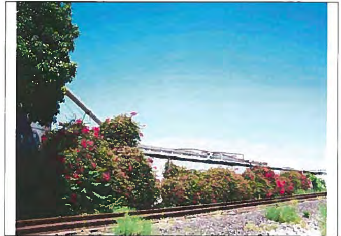
View looking northwest at the east elevation of the 1932 addition.
