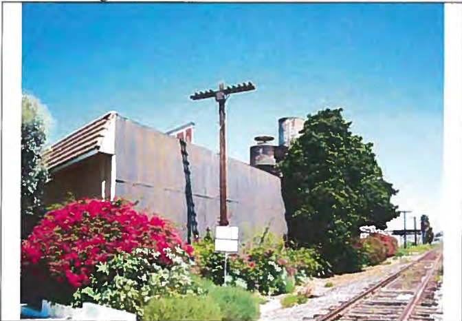
View looking northwest at the east elevation.
