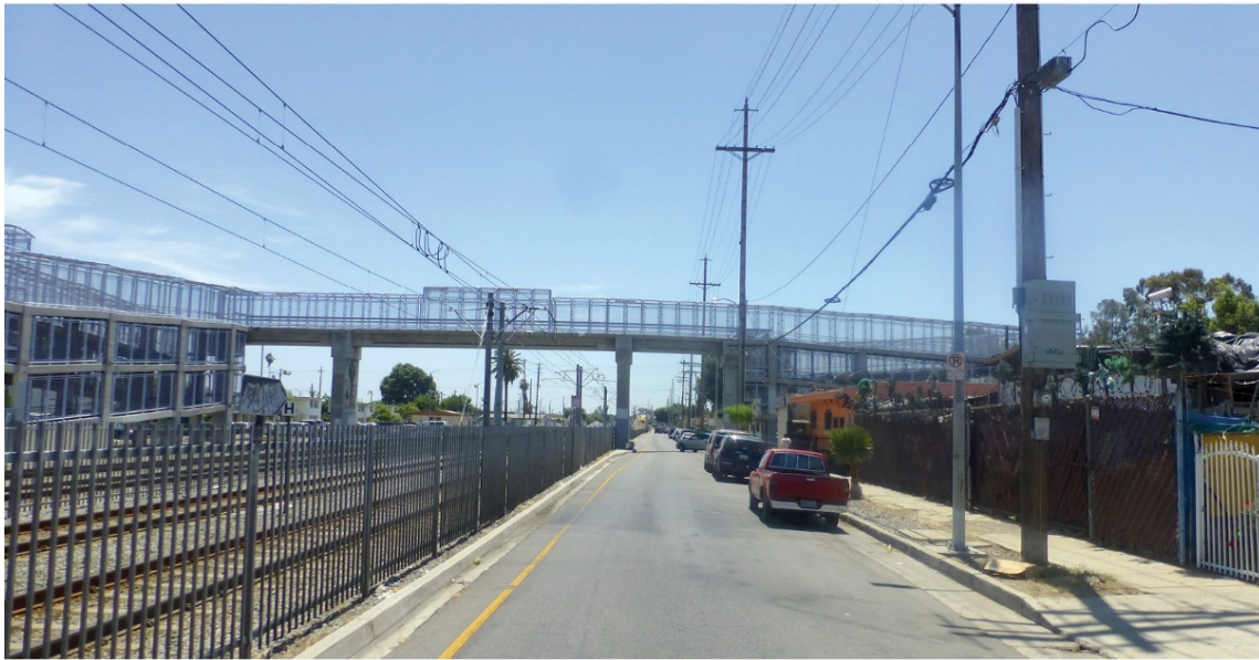
Existing Long Beach Avenue at 53rd Street Pedestrian Bridge
