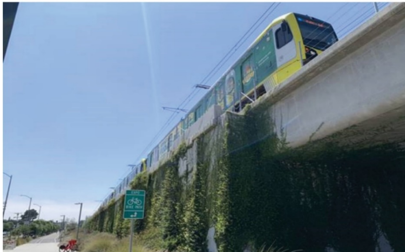
Aerial Guideway Transition to At-Grade Level over Retaining Wall on the Metro E Line
