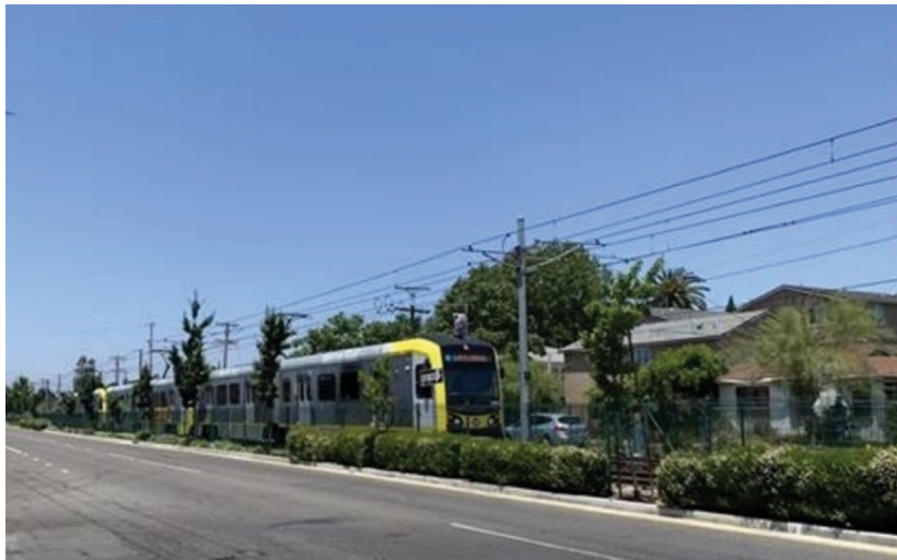
At-Grade LRT Guideway on the Metro E Line
