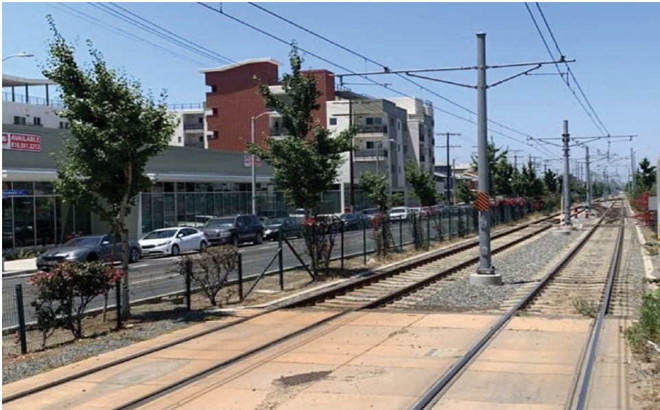
Figure 1-6. Example of Overhead Catenary System
