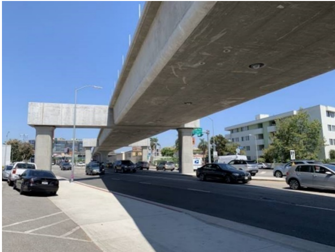
Figure 1-4. Example of Aerial Structure Straddle Bent (Metro E [Expo] Line)
