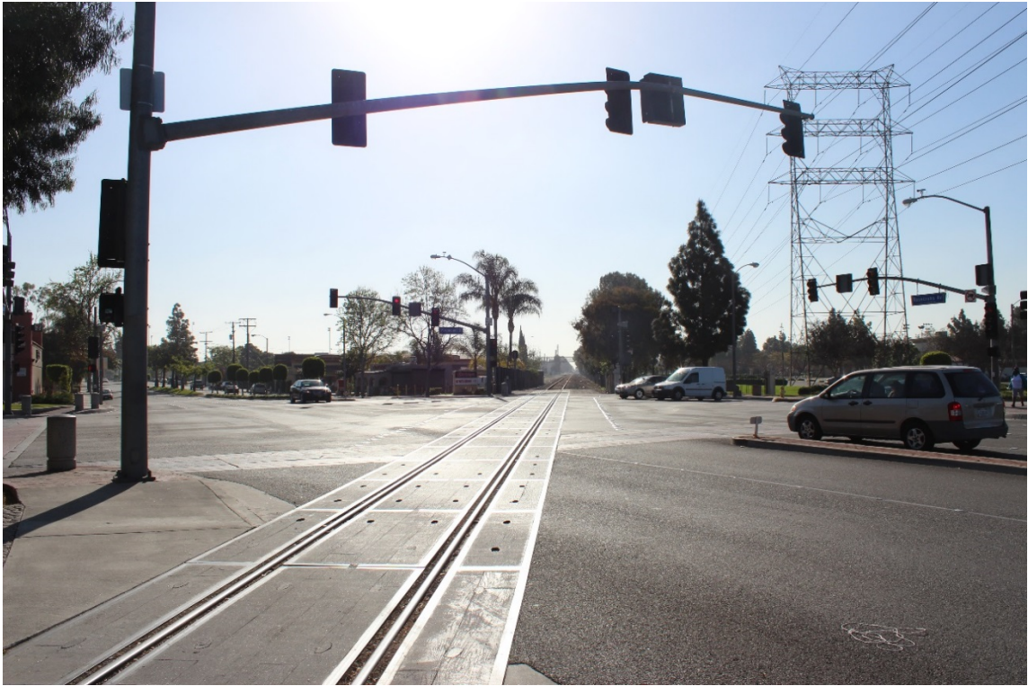
Figure 1-2. Existing Paramount Boulevard and Rosecrans Avenue At-Grade Train Crossing
