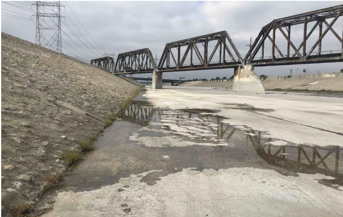
Photograph 3. Los Angeles River, facing south.
