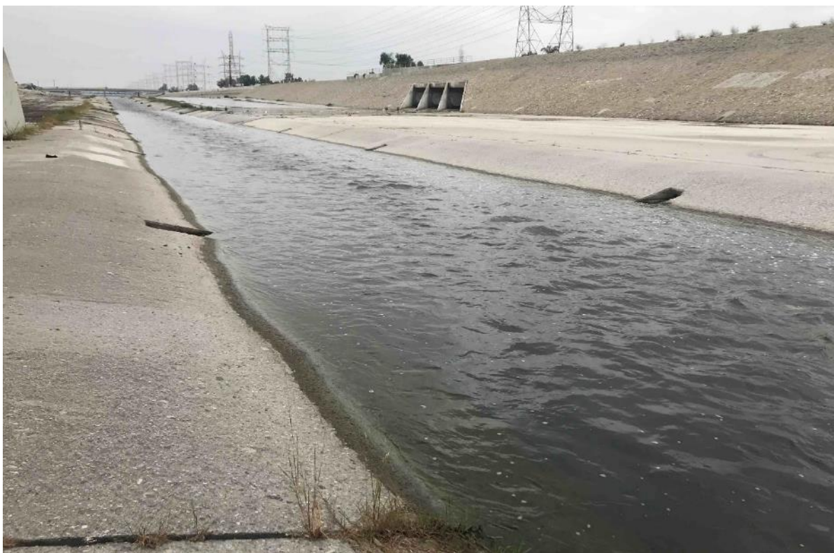
Photograph 4. Low flow channel within Los Angeles River, facing northeast.
