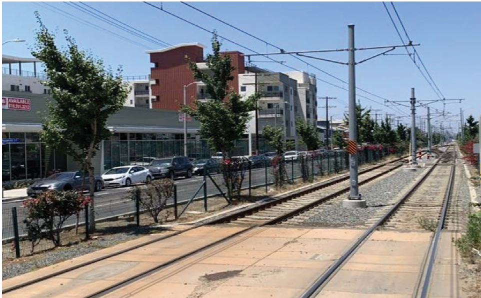
Figure 1-5. Example of Overhead Catenary System
