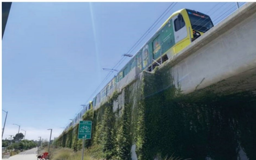
Aerial Guideway Transition to At-Grade Level over Retaining Wall on the Metro E Line
