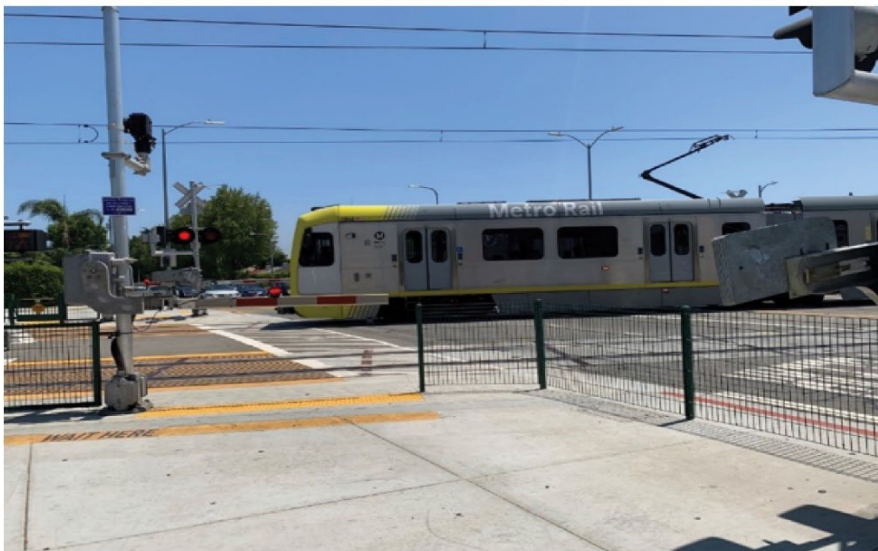
Pedestrian Gate Crossing Equipment on the Metro E Line
