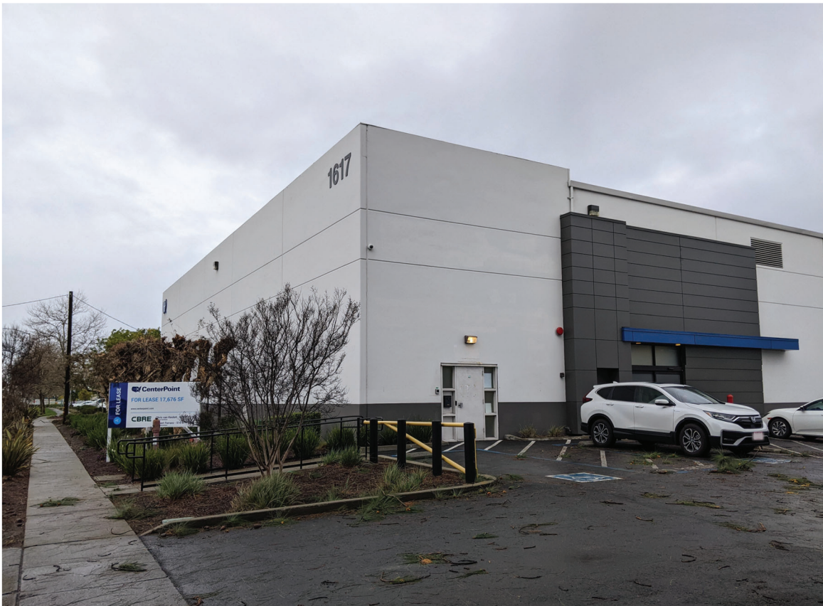
Photo 4: Existing industrial buildings at 1617 Industrial Parkway West.
