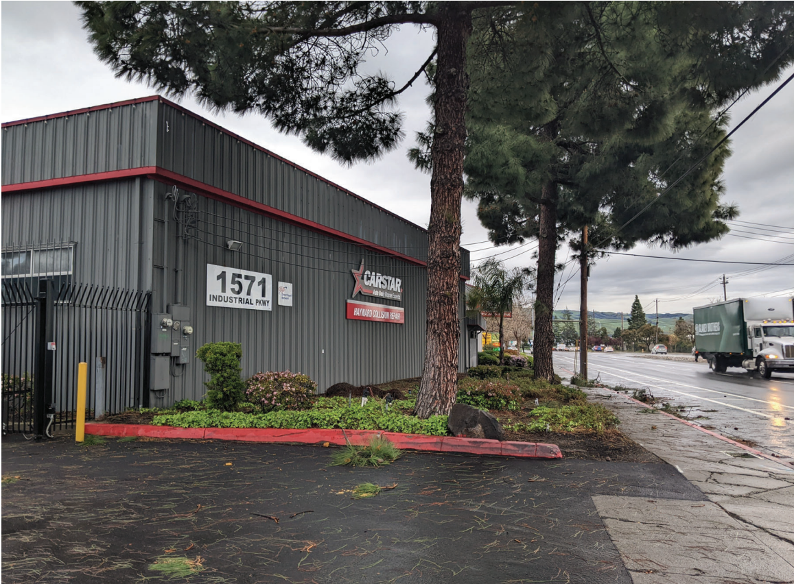
Photo 3: Existing industrial buildings at 1571 Industrial Parkway West.
