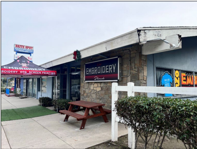
Primary elevation, west end, view east.
