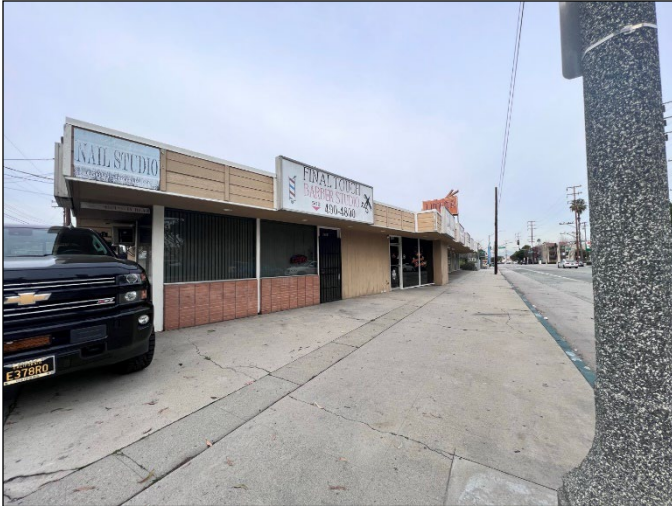
South end of primary elevation, view northwest.
