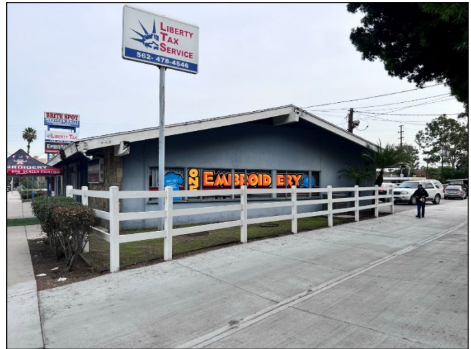
West elevation, view east.
