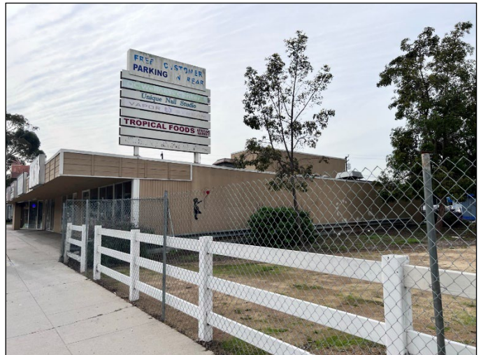
North elevation, view southwest.
