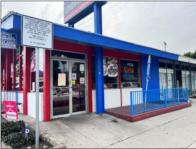
Primary elevation, east end, view south.
