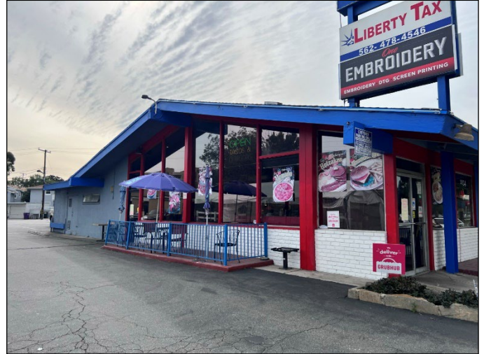
East elevation, view southeast.
