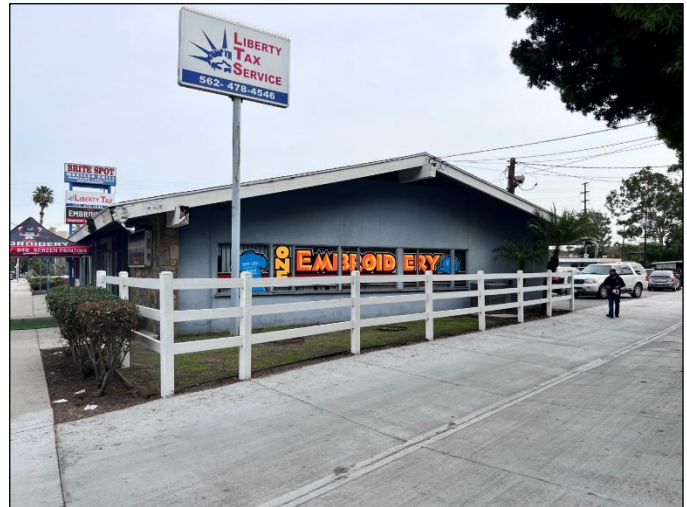
West elevation, view east.
