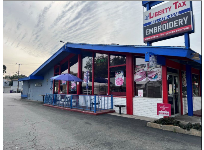
East elevation, view southeast.
