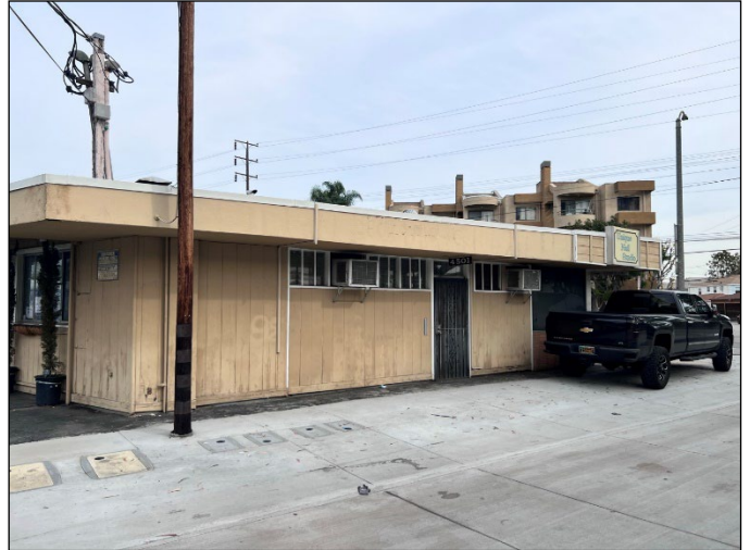
South elevation, view northeast.
