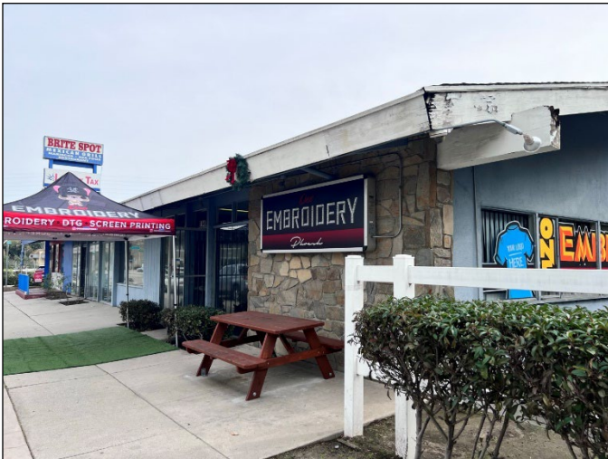
Primary elevation, west end, view east.
