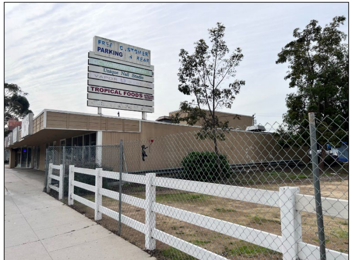
North elevation, view southwest.
