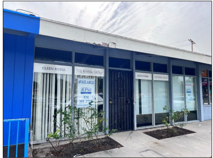
Primary elevation, center unit, view south.
