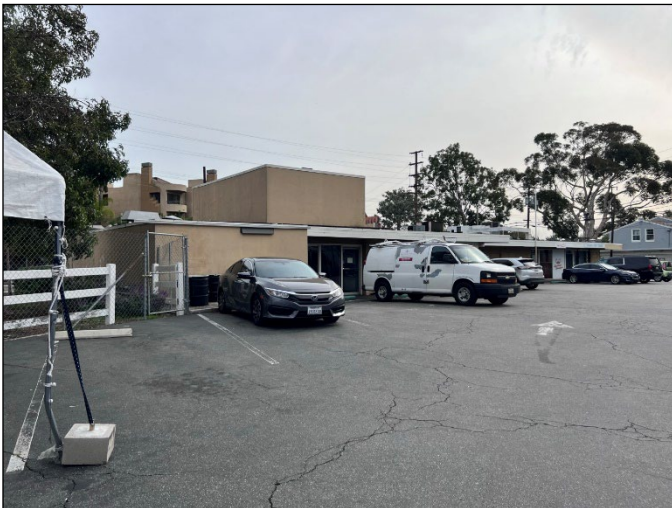
West elevation, view southeast.
