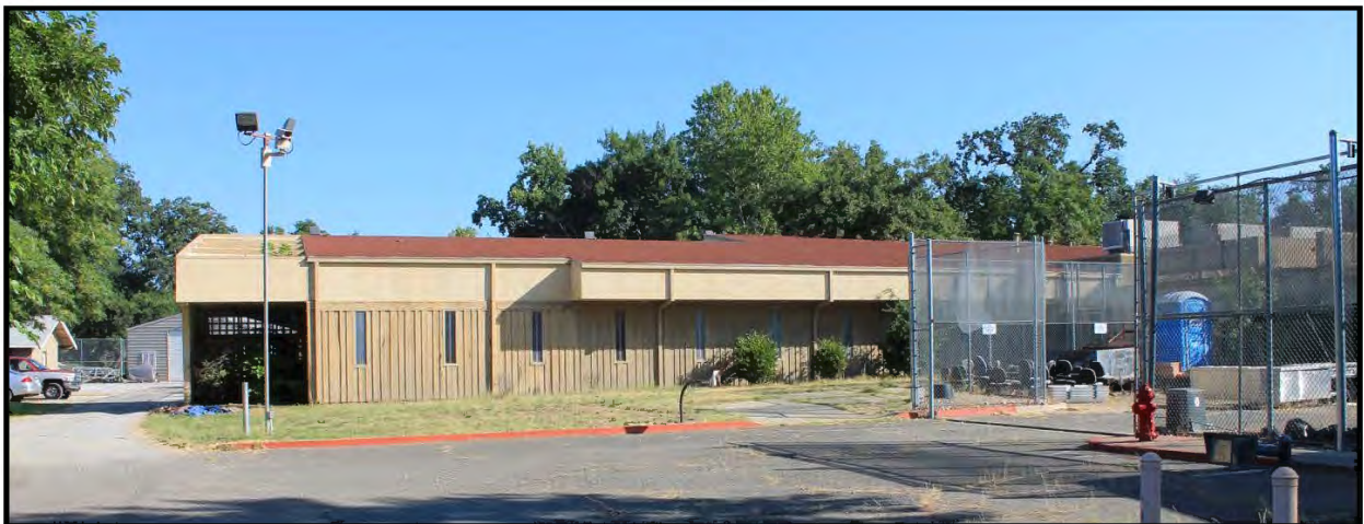
South elevation of the 1992 addition to Old SCJJC. View looking north.
