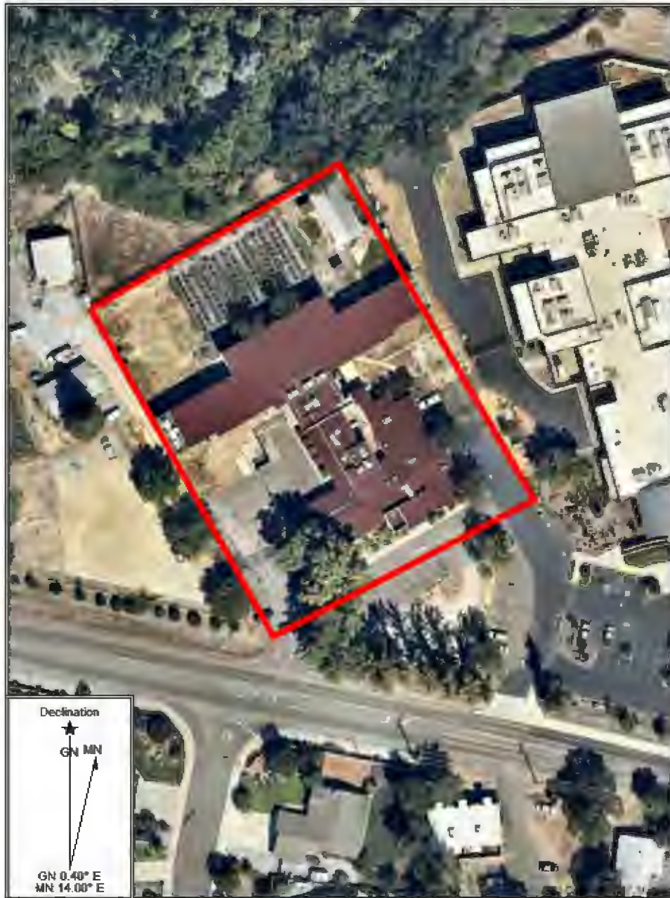
SCALE 1:1200 0 100 200 Feet Figure 2-3: Aerial Photograph Old Juvenile Justice Center 2680 Radio Lane, Redding Shasta County, CA
