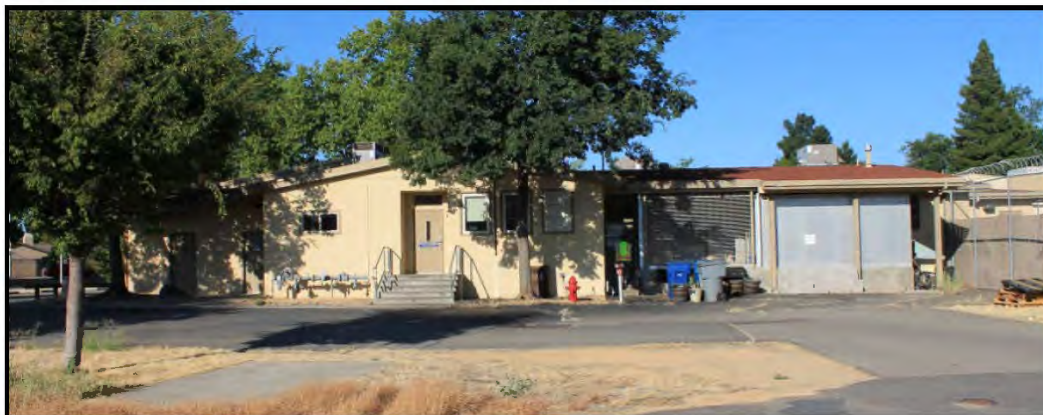
East elevation of Old SCJJC. View looking west.
