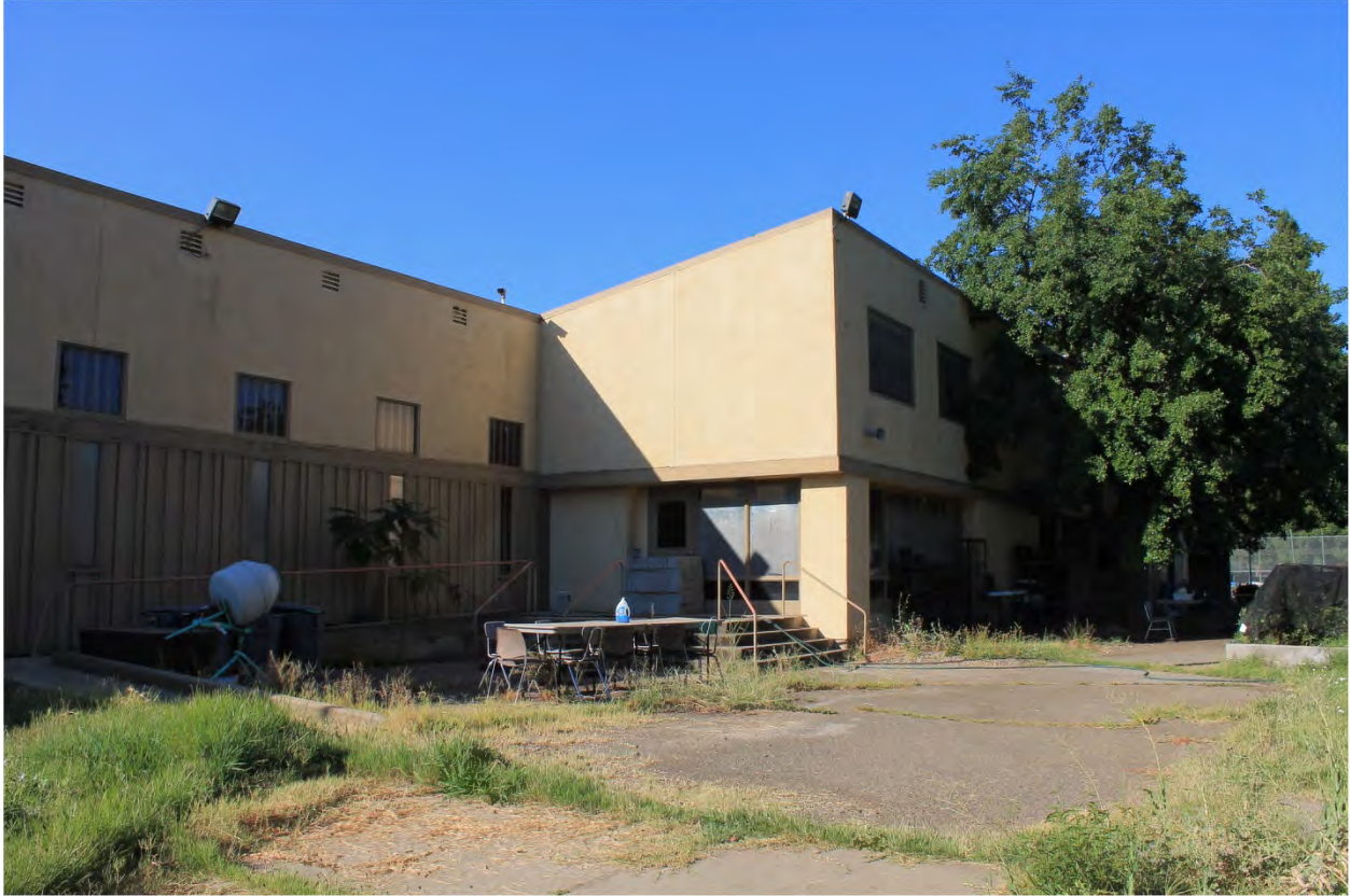
Figure 12: North elevation of the 1990 wing of the Old SCJJC. The individual bunkrooms span to the east and west from the large day room of the wing (projecting room with canted roof slope). View looking southwest.
