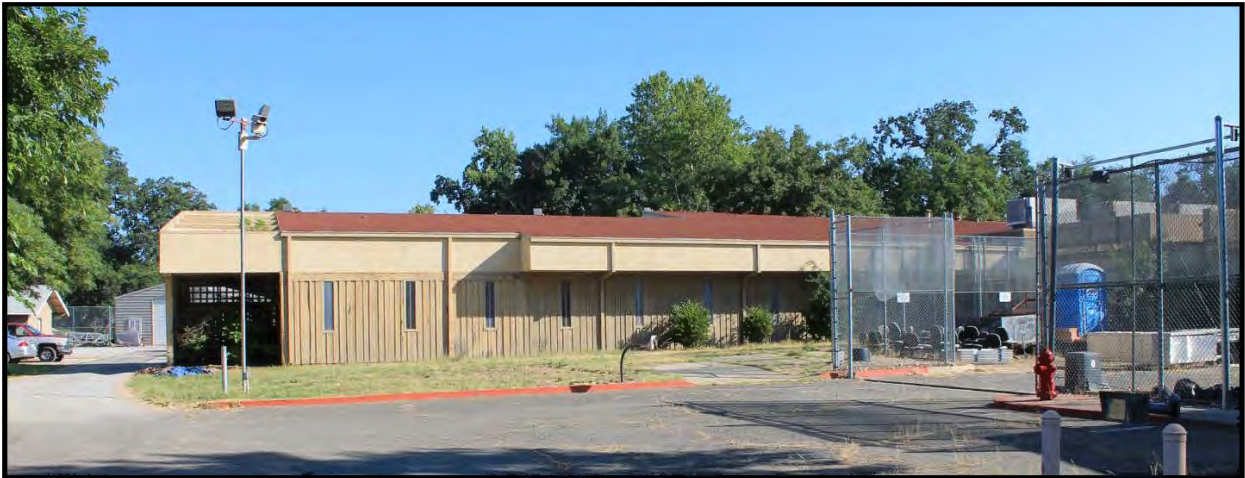
Figure 11: South elevation of the 1990 addition to Old SCJJC. View looking north.
