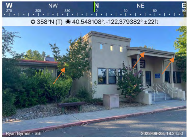
Photo 6. Photo of the main entrance to the Old Juvenile Justice Center. Orange arrows indicate potential bat entry and exit locations within the building's soffit. No bats or signs of bat use was observed during the surveys.
