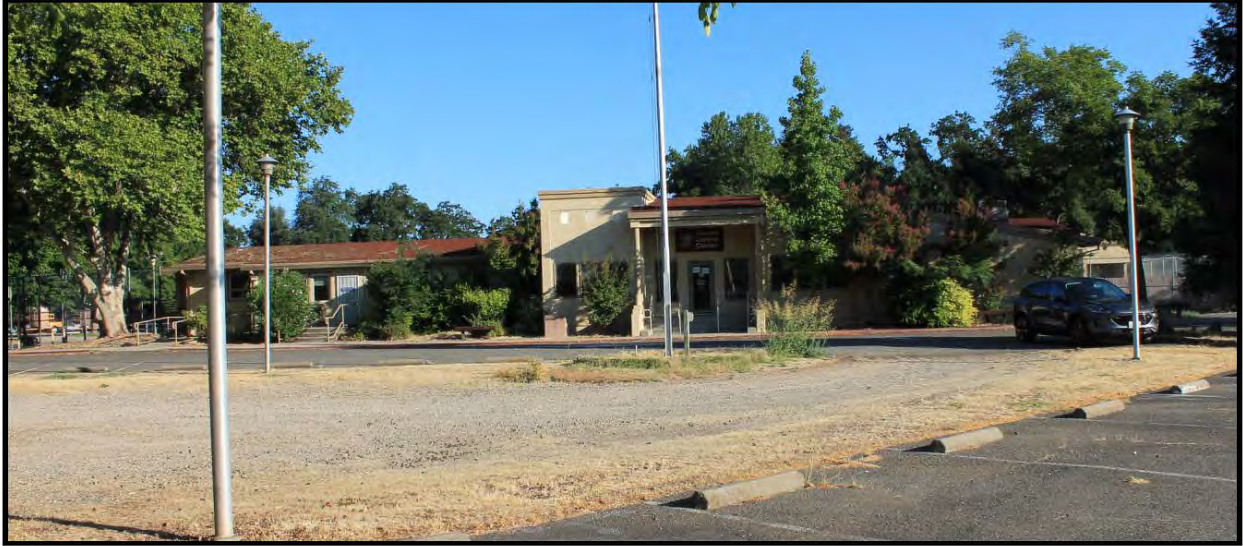
Figure 8: Front (south) elevation of OLD SCJJC. View looking north.
