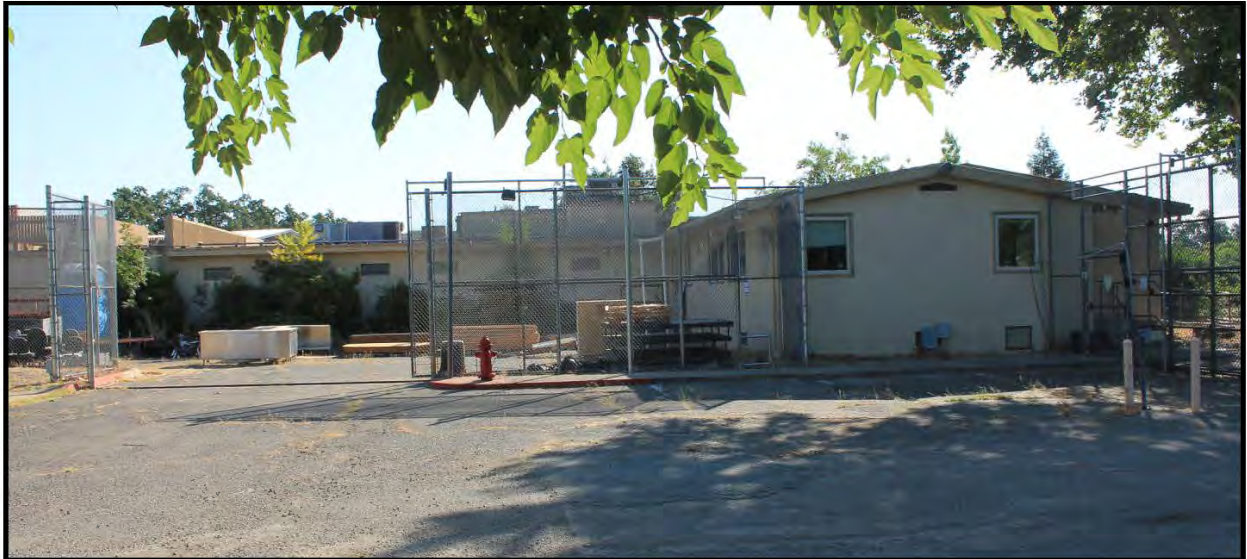
West elevation of the original main block, with the west elevation of the security wing on the left. View looking east.
