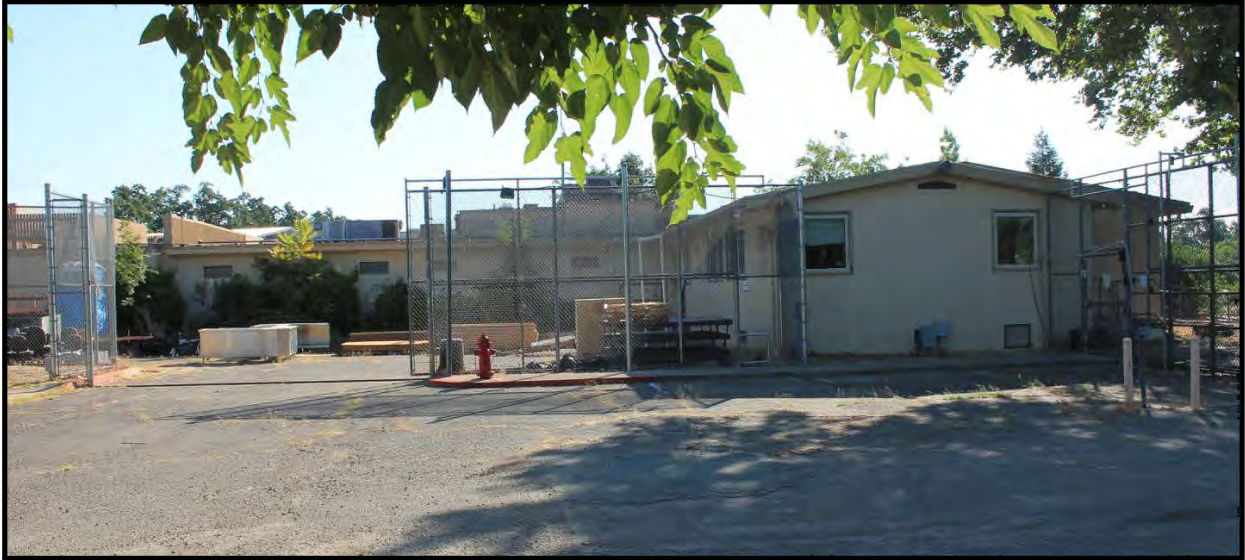
Figure 10: West elevation of the original main block, with the west elevation of the security wing on the left. View looking east.
