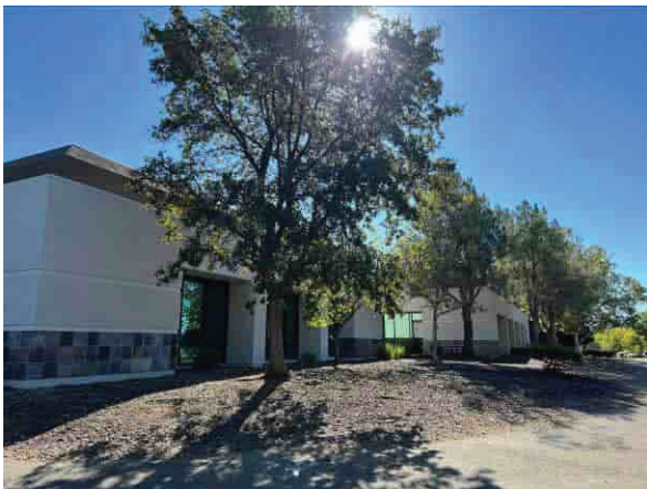
Photo #11 View of northeastern adjoining property.
