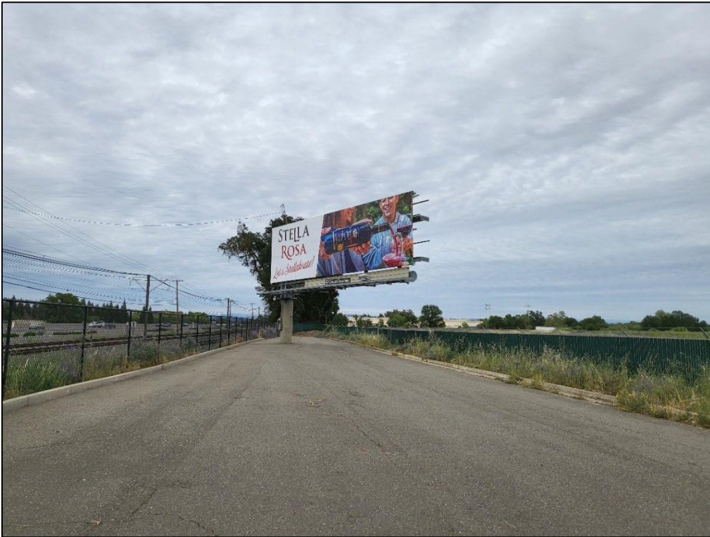
Photo 3. Overview of existing billboard that is proposed for removal, facing east
