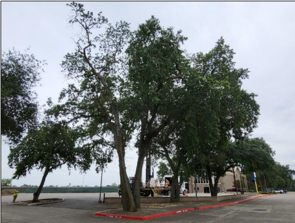
Photo 8. Overview of continued access to west side of parcel near existing building
