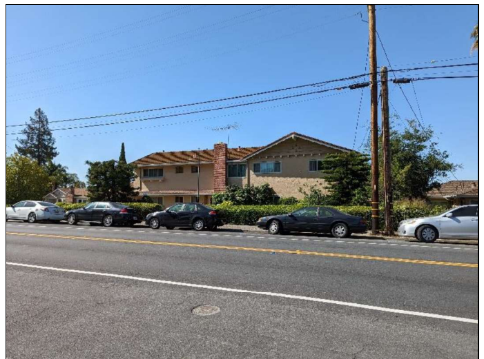
24. View of the west adjacent property at 133 Kirk Avenue
