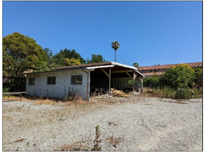
14. View of the open-air shed from the southeast
