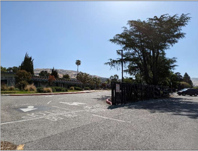
19. View of the north adjacent property
