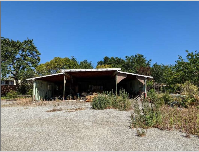
13. View of the open-air shed from the east
