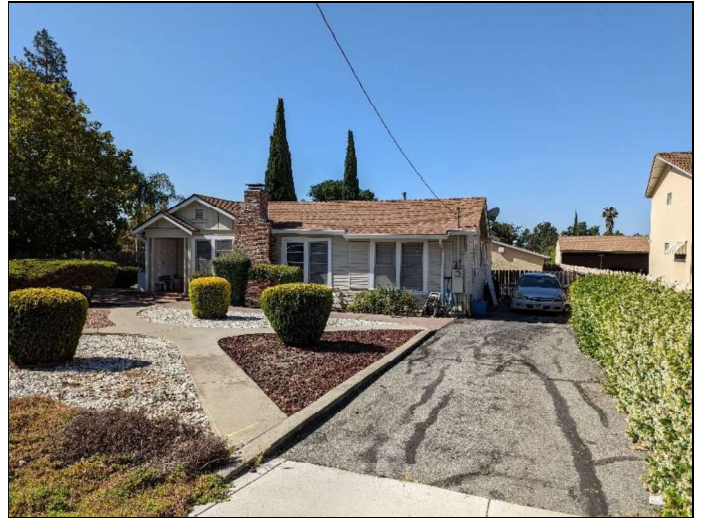
2. View of the subject property building from the northwest
