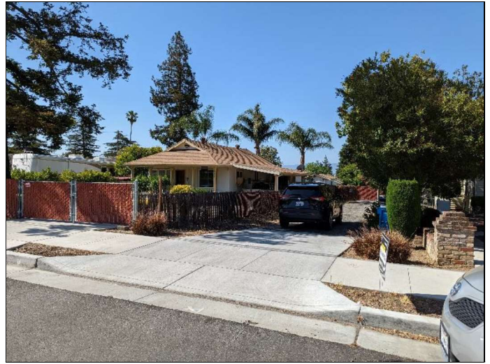
20. View of the east adjacent property at 117 Kirk Avenue
