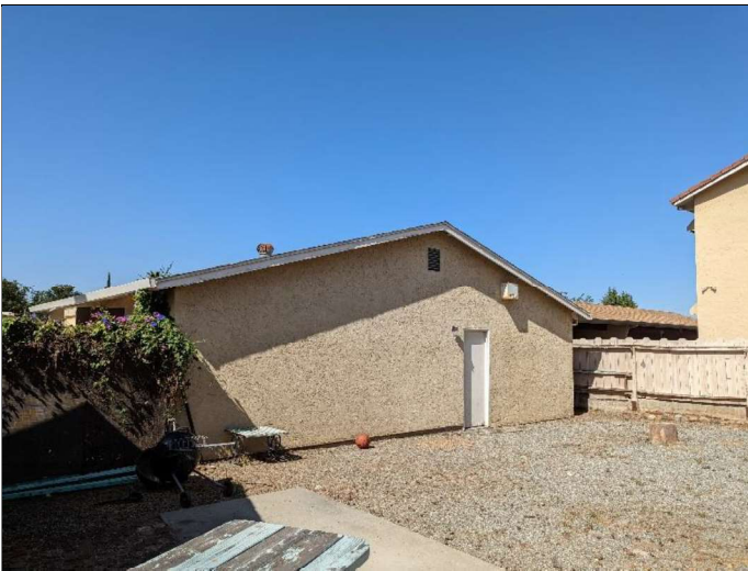
9. View of the detached garage from the north
