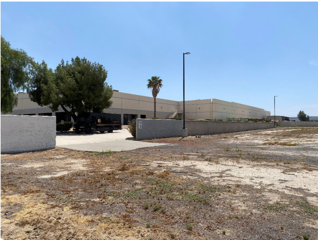
G-2. Entrance to Parcel 13 (06/03/2022).
