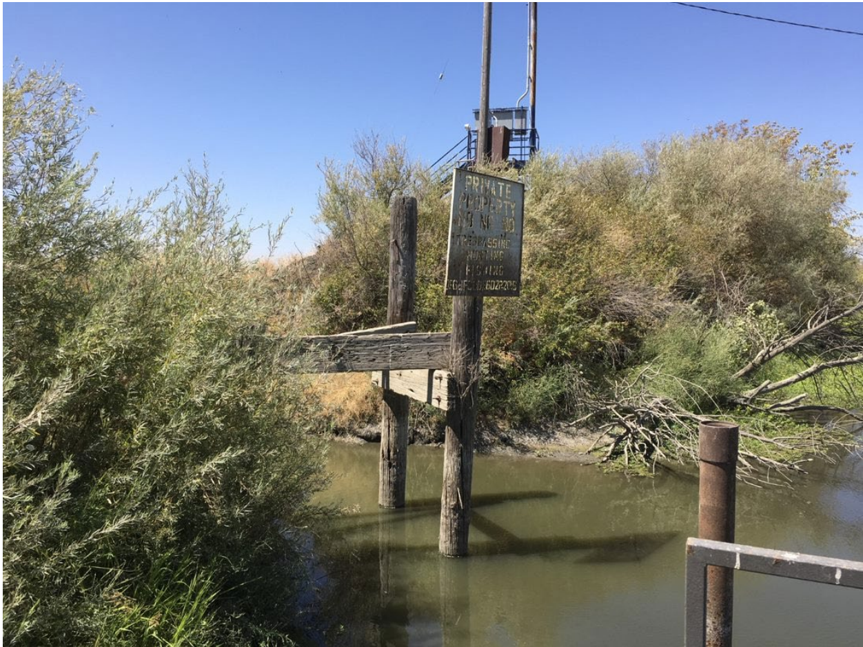
Photograph 3. Site of proposed concrete headwall fish barrier . (June 2022)
