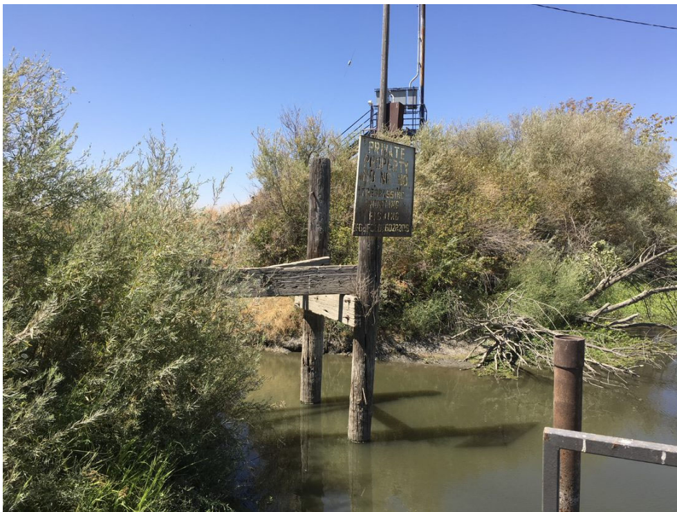
Photograph 2. Site of proposed concrete headwall fish barrier. (June 2022)
