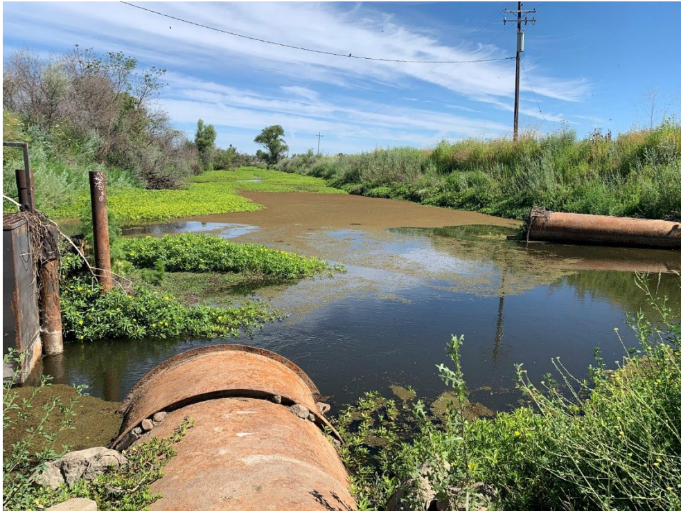
Photograph 1. Tule Canal looking north. Left side of photo is the site of proposed concrete headwall fish barrier. (June 2022)
