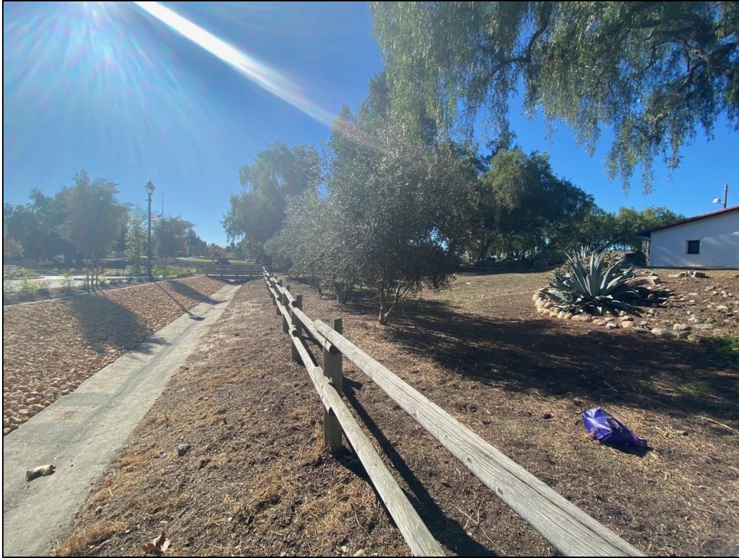
Figure 8. Drainage canal at rear of NRHP listed Blas Aguilar Adobe (right), facing southwest
