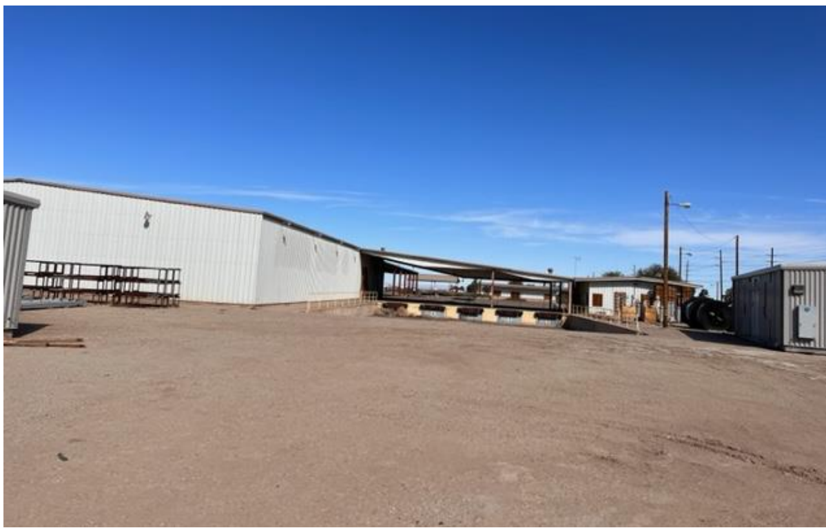
Photo 5: View north from Villa Avenue towards Bonanza Building and surrounding structures located at the northwest corner of Dogwood Road and Villa Avenue to be demolished to accommodate construction of the 9-acre, three cell evaporation pond.
