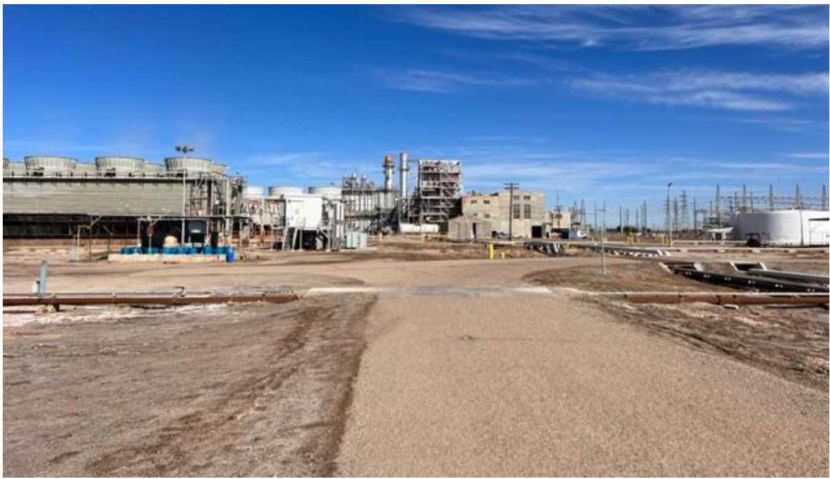
Photo 4: View north along internal access road/pipeline alignment.
