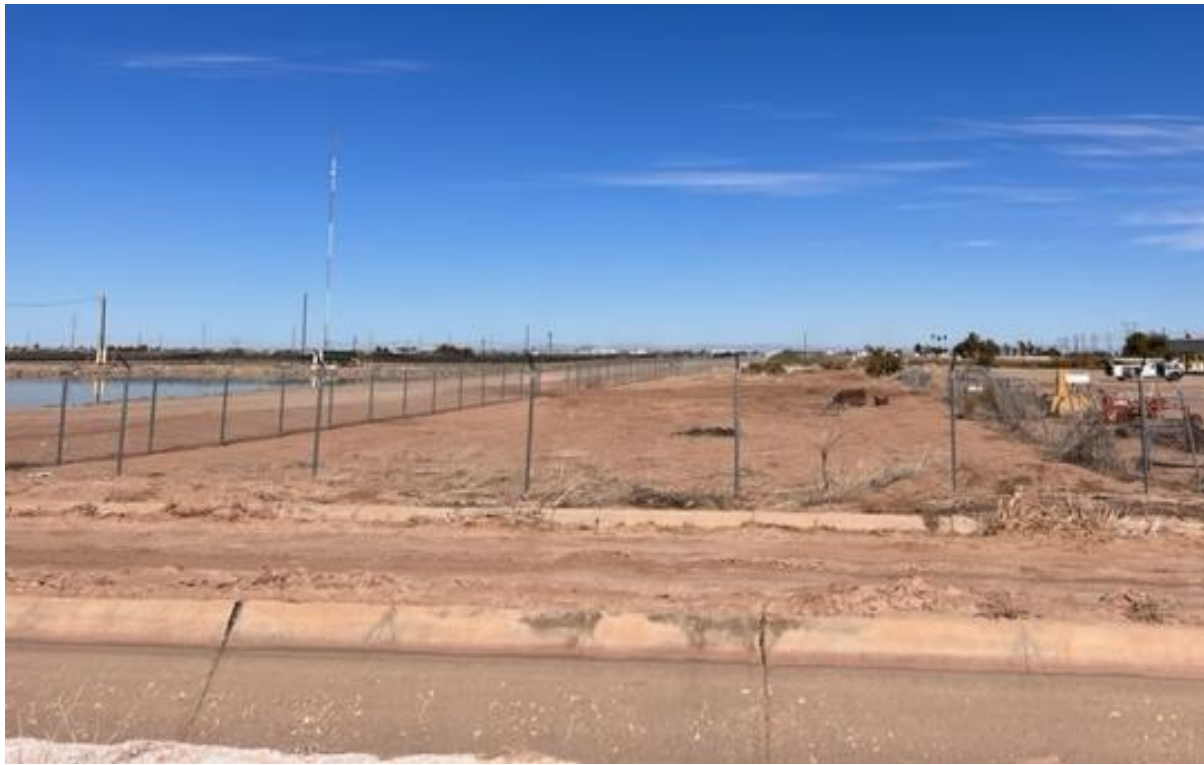
Photo 9: View north from Villa Avenue towards location of 9-acre, three cell evaporation area. Bonanza Building and associated structures to be demolished are to the east.
