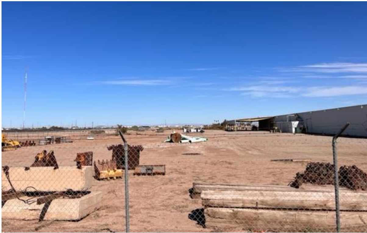
Photo 7: View north from Villa Avenue towards 9-acre, three cell evaporation pond area. Building at right will be demolished.
