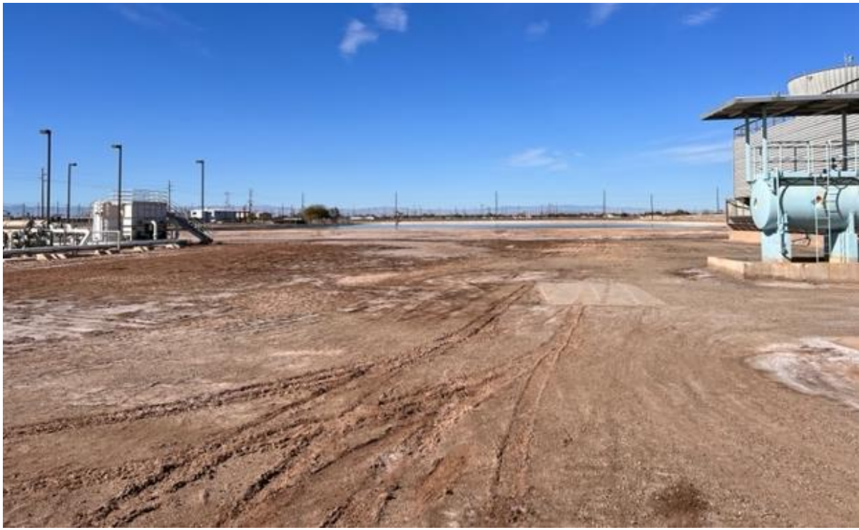
Photo 3: View west from Dogwood Road towards location of proposed treatment equipment.
