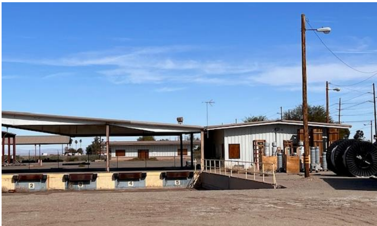
Photo 6: View north from Villa Avenue towards Bonanza Building View and surrounding structures, located at the northwest corner of Dogwood Road and Villa Avenue to be demolished to accommodate construction of the 9-acre, three cell evaporation pond.
