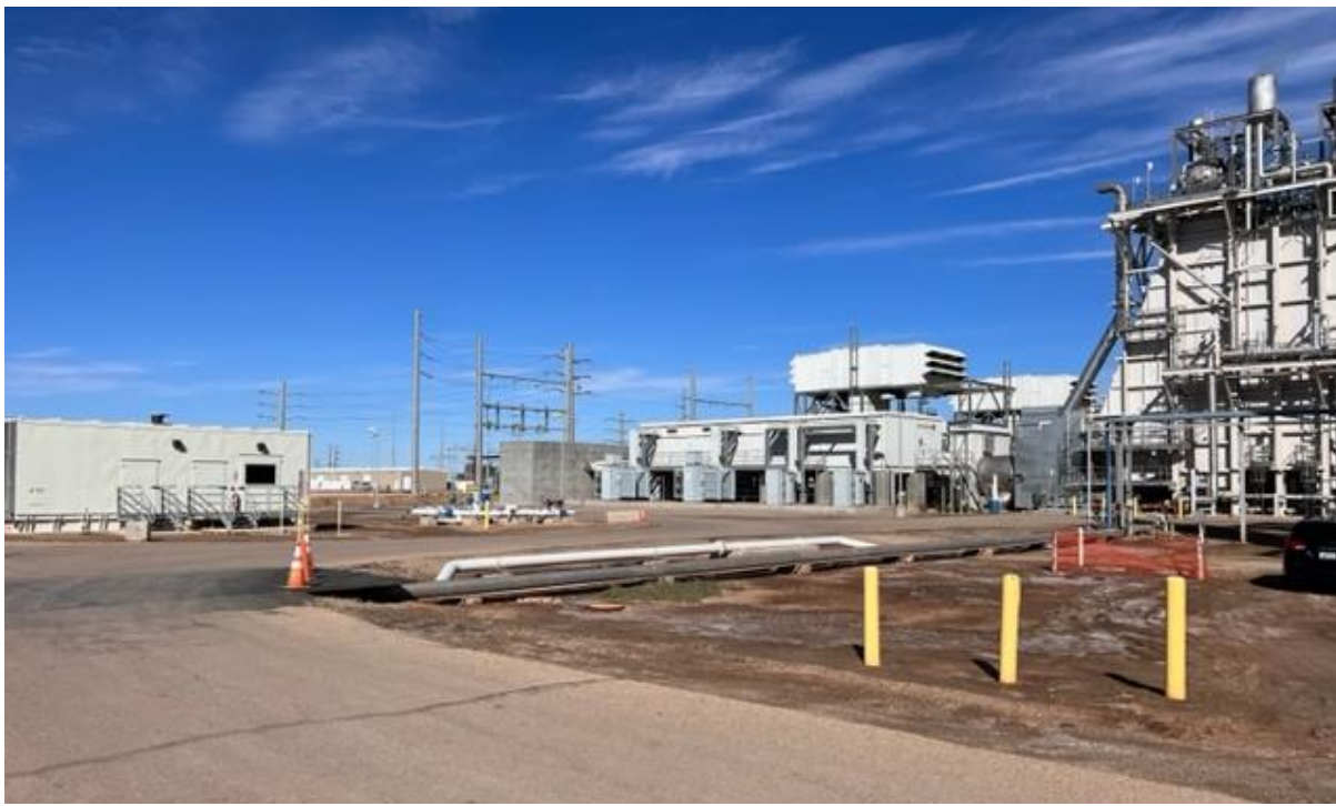
Photo 1: View southeast from internal roadway. Pipeline alignment would extend from building at right of photo.
