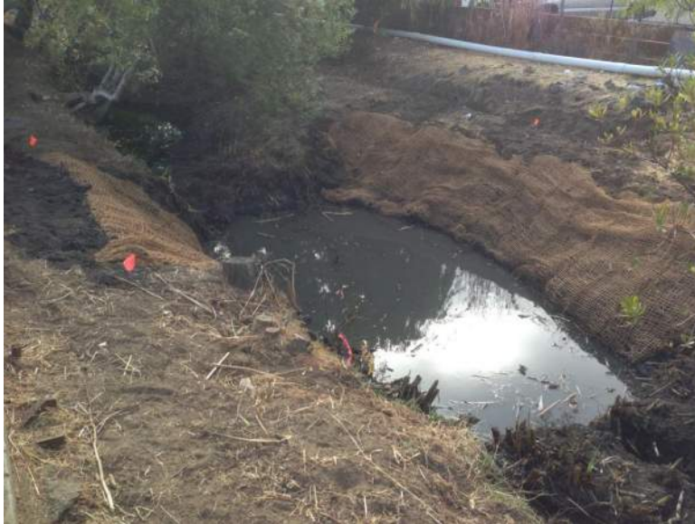
7. New excavated pool located between two protected scour pools.
