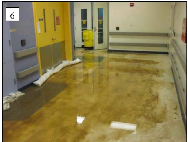
Figure 3. Photographs of siltation inside and outside of the structure located at 120 and 150 Industrial Road
