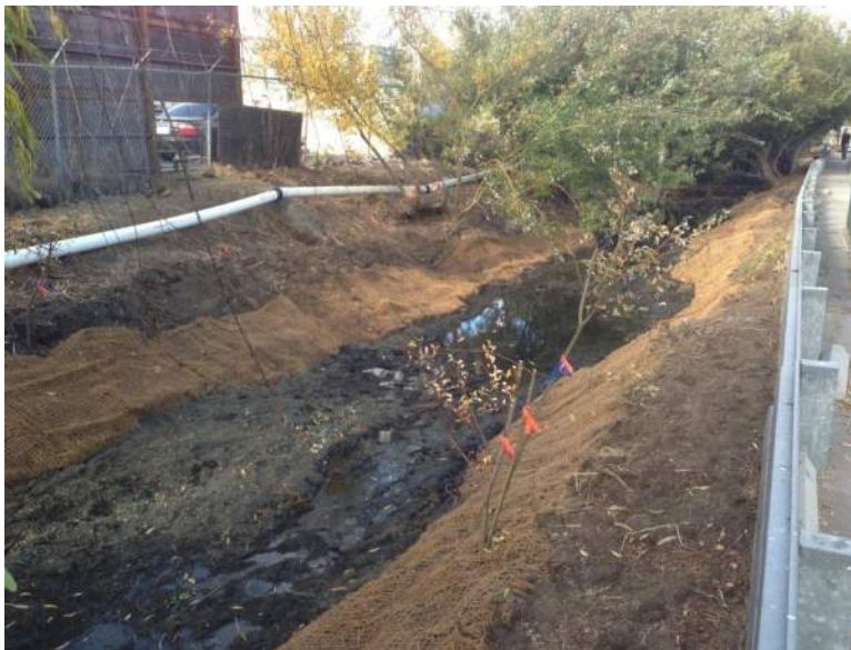
6. Mid reach of Project Area showing Coir netting and placement of pin flags to mark container planting locations. Green willow stakes can be seen in the foreground and on left bank.
