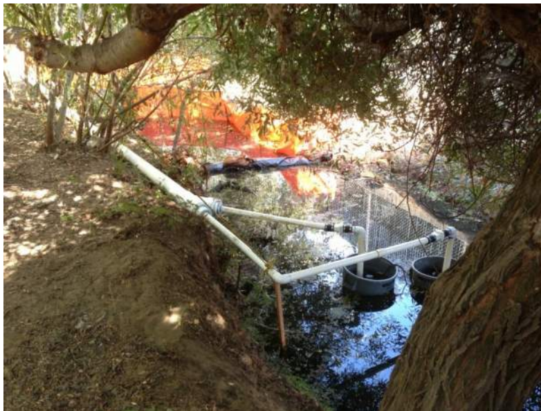
2. Photograph shows upstream coffer dam and by-pass pump configuration.
