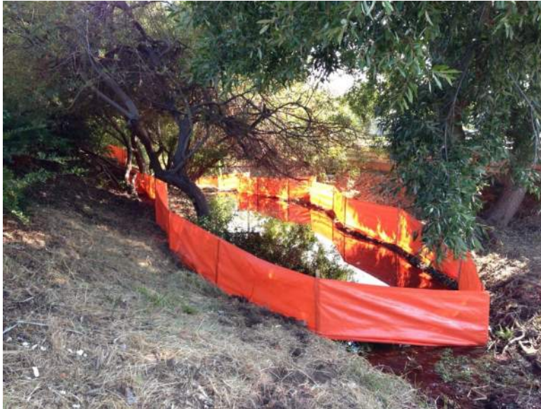
1. Representative photograph of ESA/silt fencing around one of the protected/avoided scour pool features within the Project Area.
