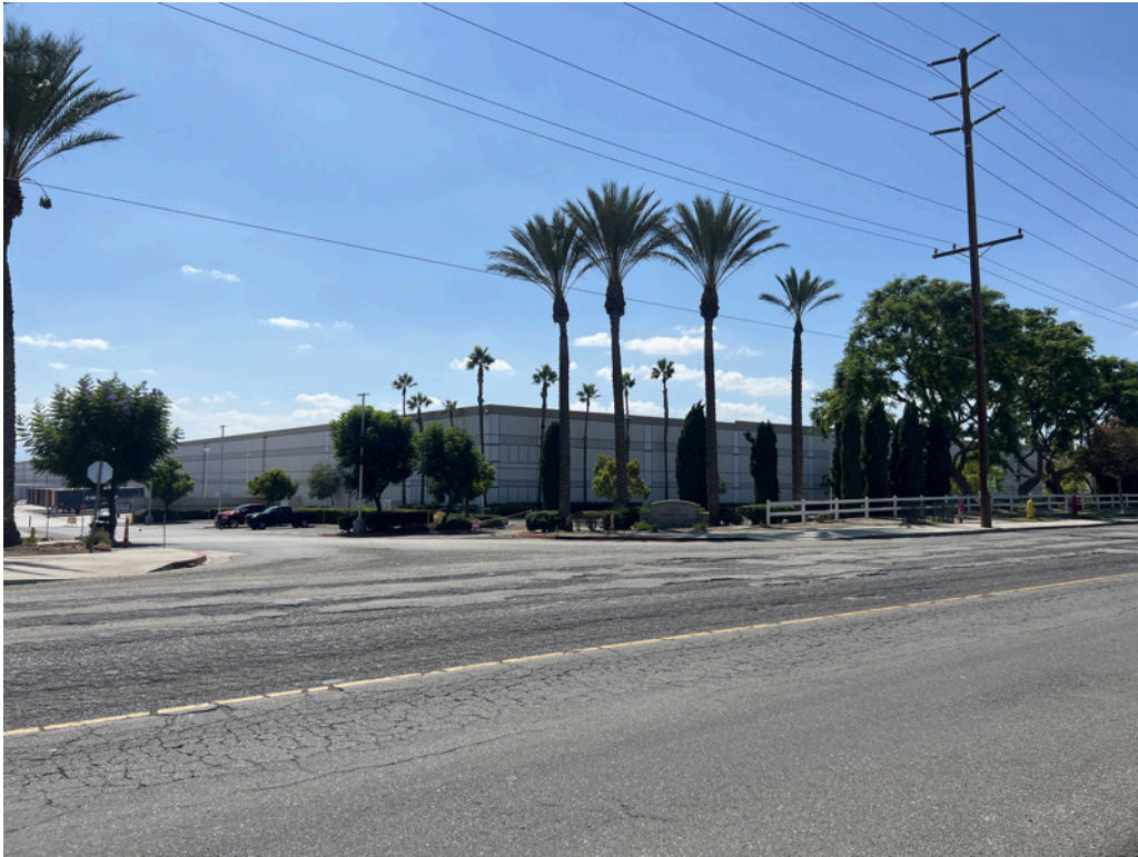
15. South adjoining property (Damco)
