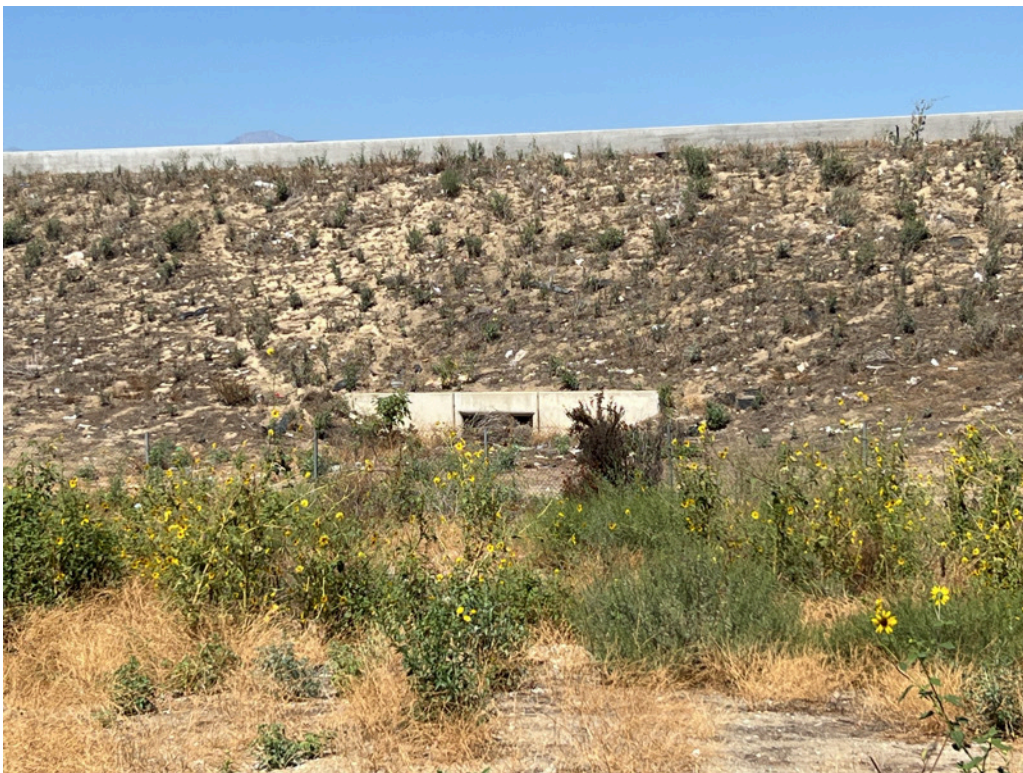
12. Underpass of Pomona Freeway north of subject property
