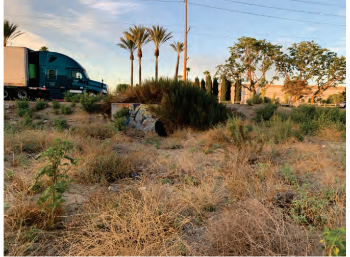
6. View facing south of culvert at Riverside Avenue. Photograph taken August 12, 2022.
