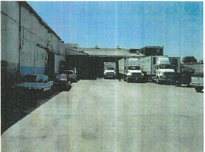
VIEW OF DOCK AREA
