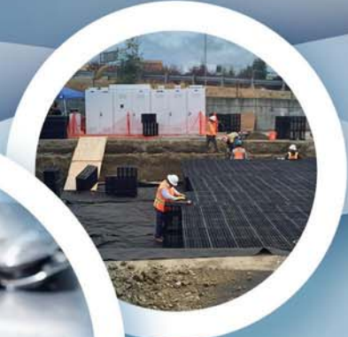
Installing retention chambers for well flushing at Gish Station
