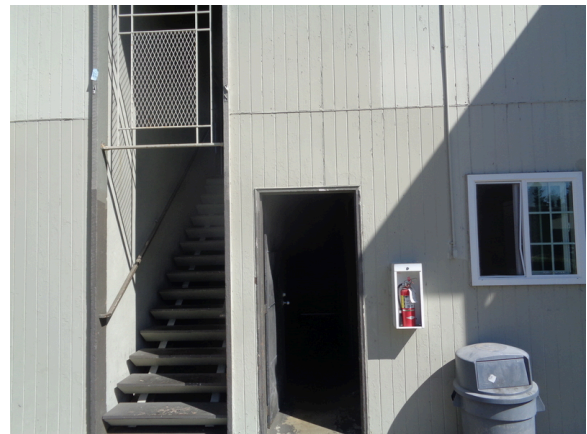
24. Staircase and access to parking
