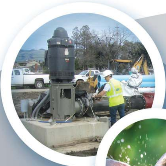
Connecting the last piece of piping for well operation at McLaughlin Station
