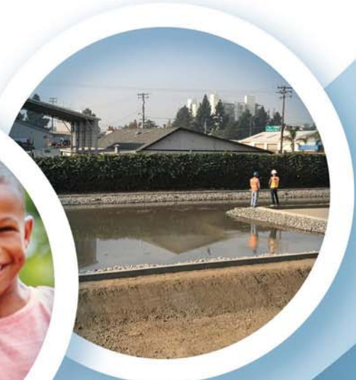
Gish station's system for retention of well flushing water
