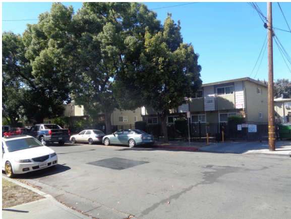
27. North adjacent property - 1319 Tripp Avenue
