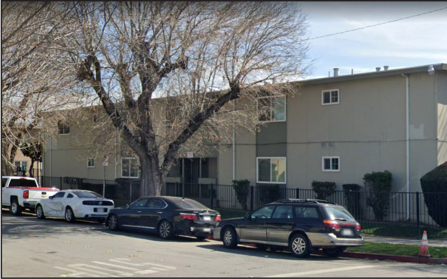
Photo #5: East facing view of apartments from N. 26th Ave. Source: Google - March 2021
