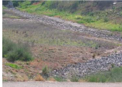
Figure 3: Gravel filled low-flow trench
