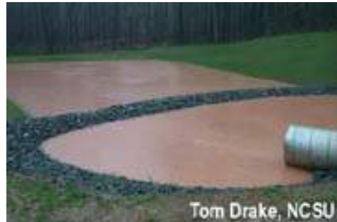
Figure 2: Forebay filled with storm water
