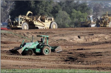
Figure 7-11: Construction graders, Inland Empire
