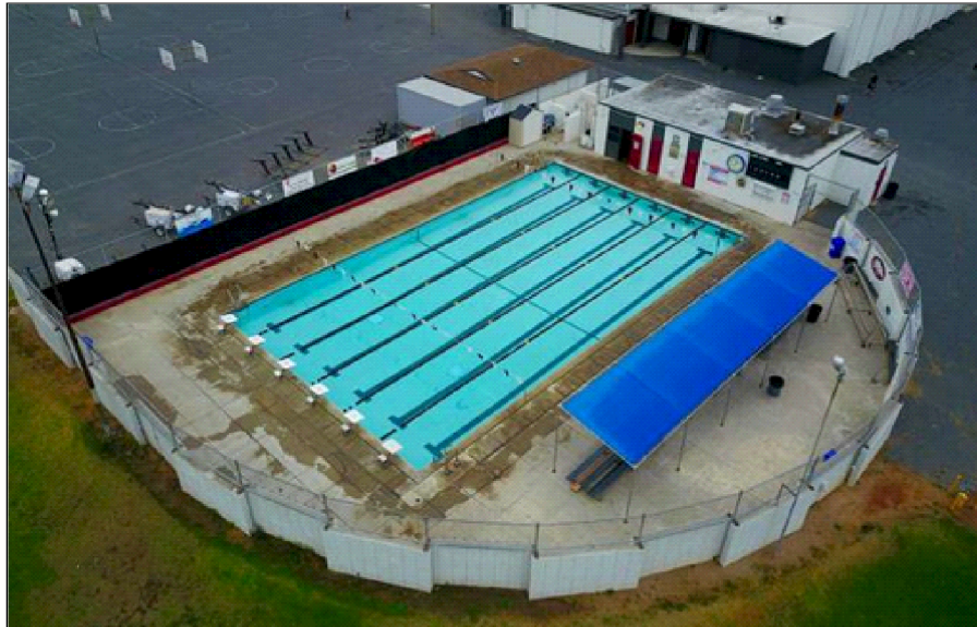
Aerial view of the existing aquatics facility with the pool, pool deck, pool house, and storage shed.
