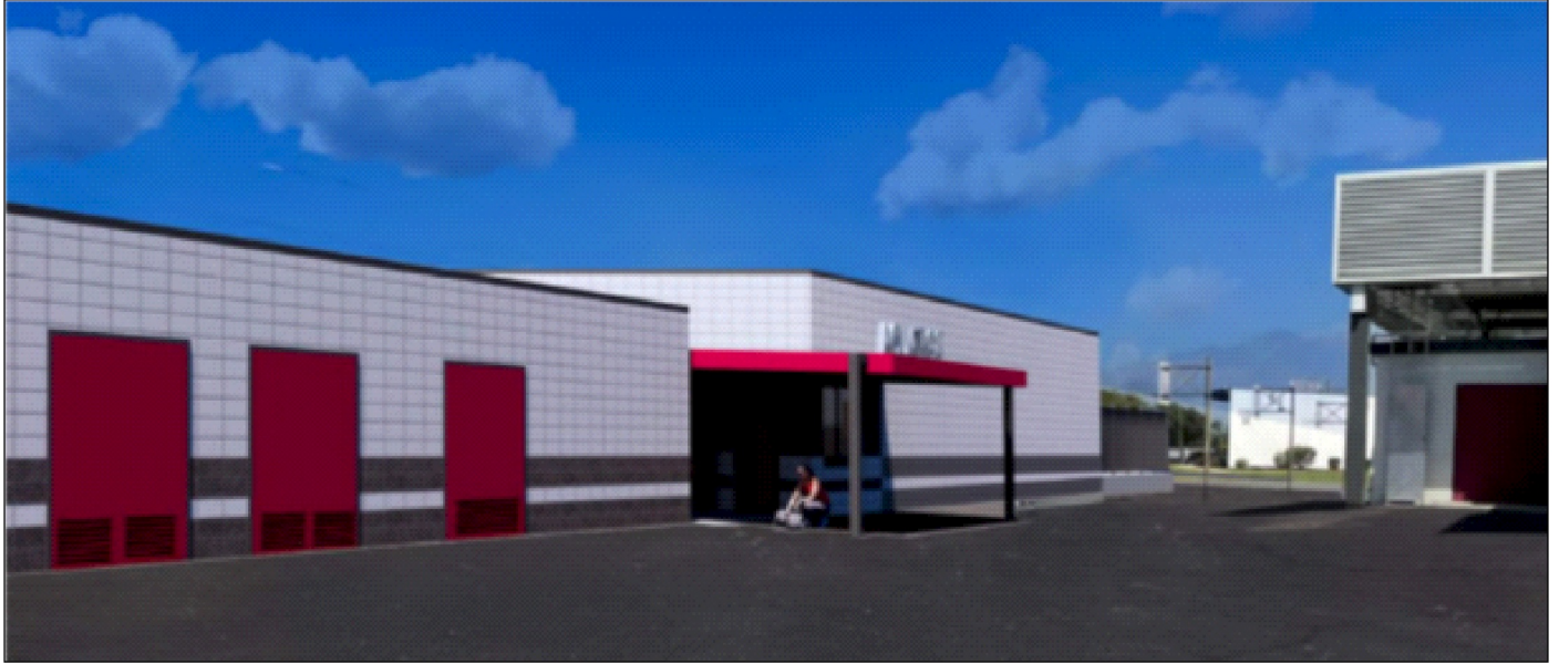
View of the east side of the proposed aquatic building from southeast of the Project site. The three red doors would provide access into the pool equipment room.
