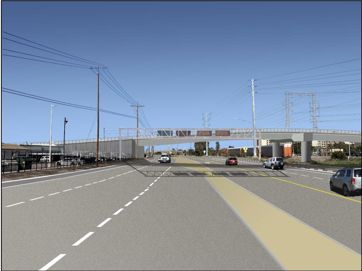
Figure 2-9: Key View 2 Proposed Condition – Build Alternative (Vesta Street Bridge Option 1, Cast in Place Box Girder with Outrigger Bent) (Northwest View)
