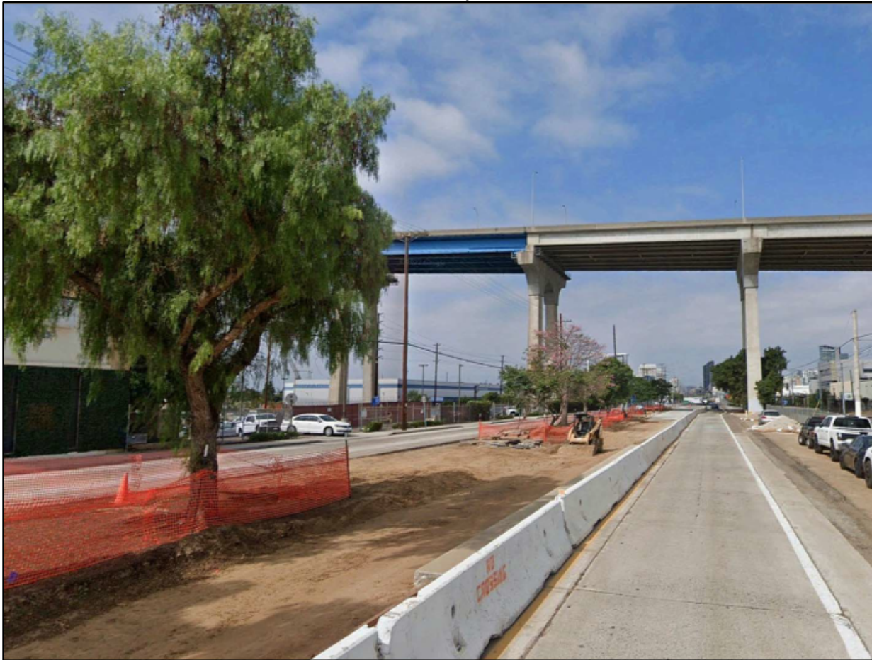
Figure 2-13: Key View 4 Existing Condition – No Build Alternative (Northwest View)
