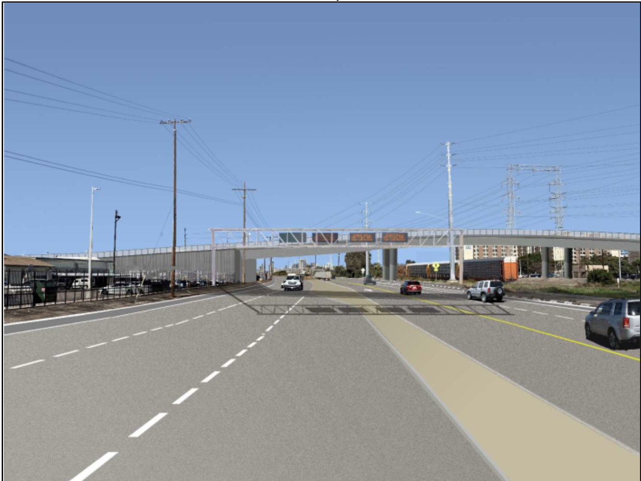
Figure 2-10: Key View 2 Proposed Condition – Build Alternative (Vesta Street Bridge Option 2, Precast Wide-Flange Girder Structure with Columns) (Northwest View)
