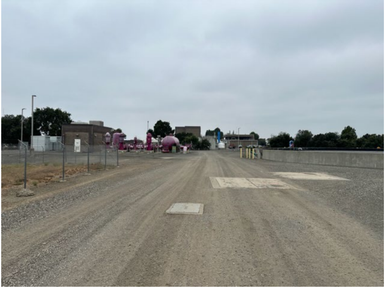
Photo 2: View of the Project Site Looking West
