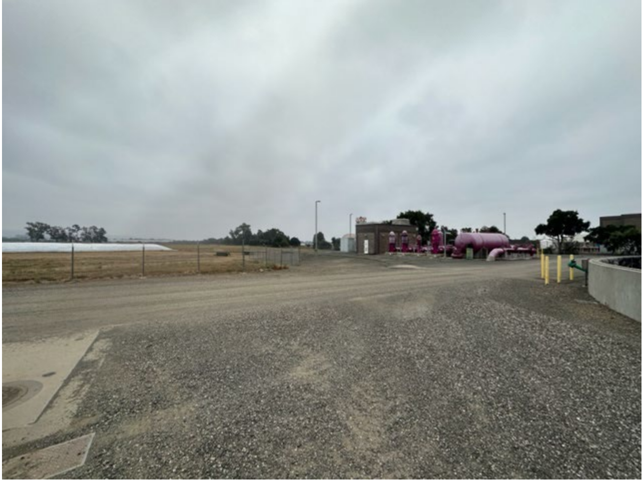
Photo 2: View of the Project Site Looking South West
