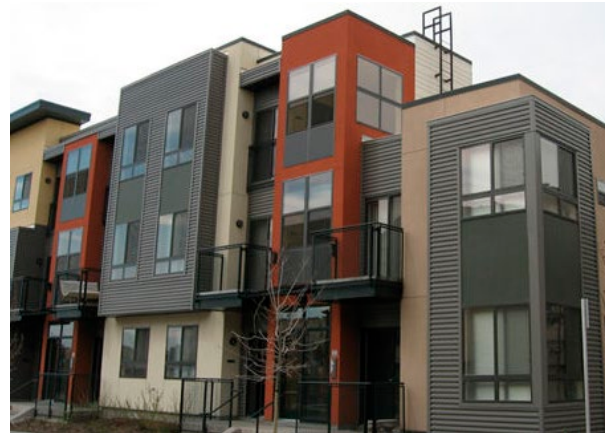
Color used to enhance façade. Source: ArchiExpo
