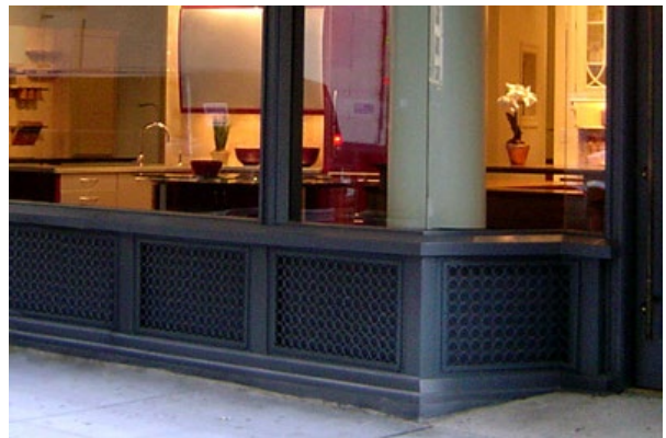
Bulkhead detailing on an urban storefront.
