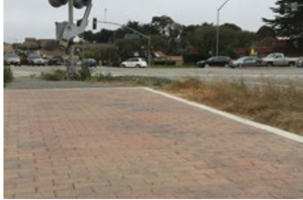
Permeable materials such as these interlocking pavers may be used to minimize runoff.
