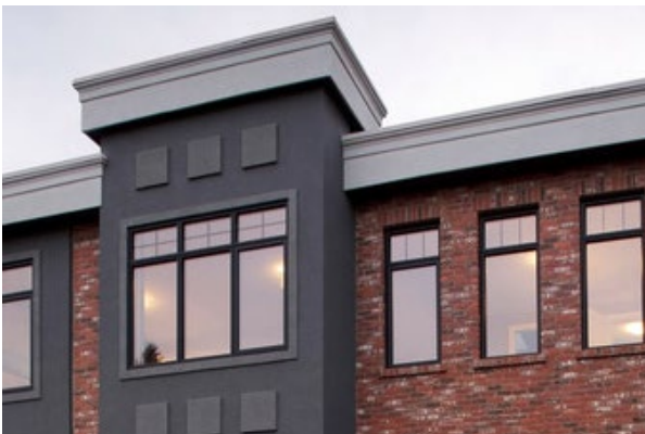
Cornice and parapet detailing.
