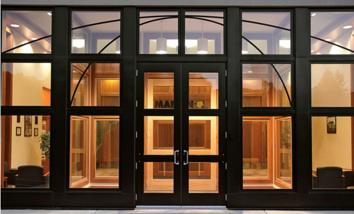
Building entry with transom window. Source: General Millwork Supply
