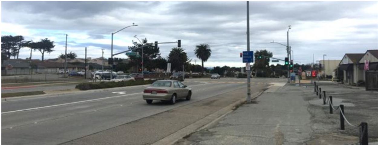
Figure 2-7. Typical portion of Del Monte Blvd with wide travel lanes for automobiles and missing sidewalks.
