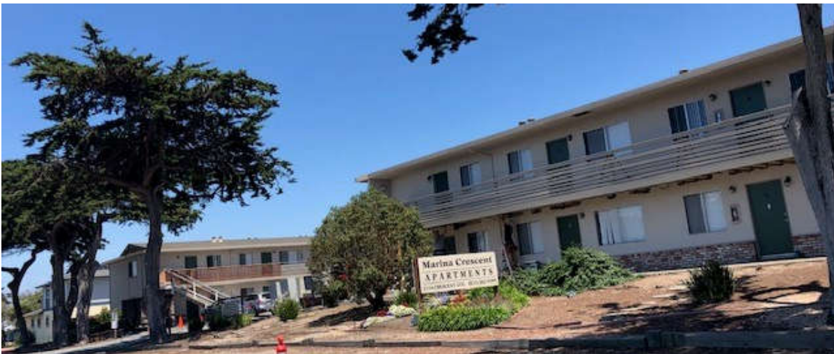
Photograph 2. Multi-family use on Crescent Avenue
