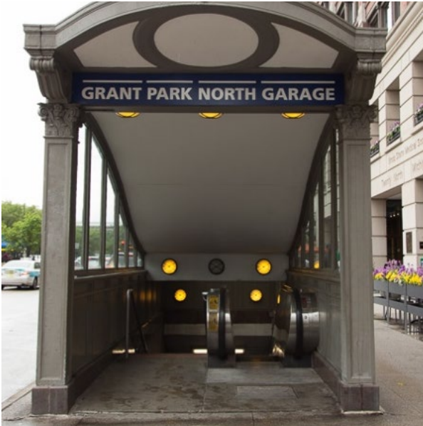
Pedestrian entrance to parking structure. Source: ParkWhiz
