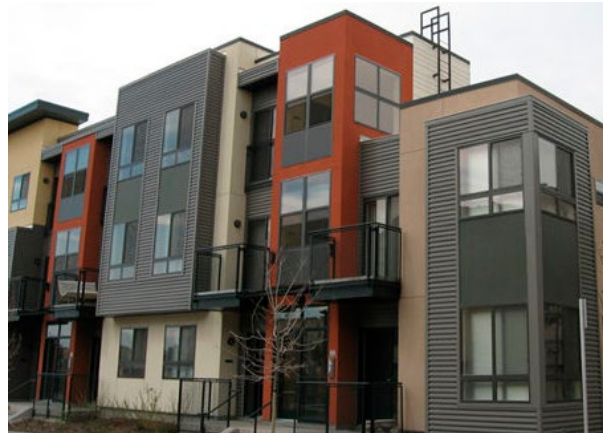
Color used to enhance façade.
