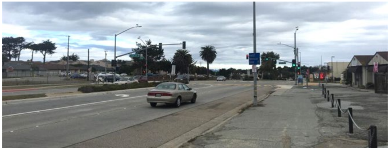
Figure 2-7. Typical portion of Del Monte Blvd with wide travel lanes for automobiles and missing sidewalks.
