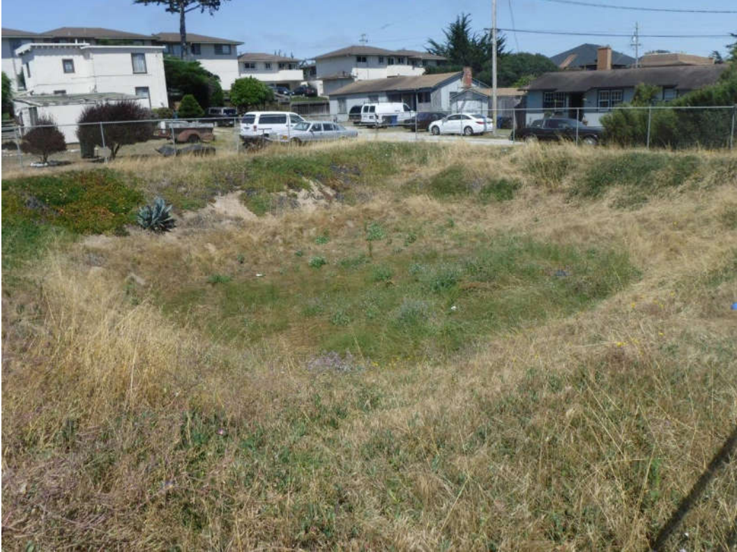
Photograph 1. A detention basin on Cypress Avenue, facing east
