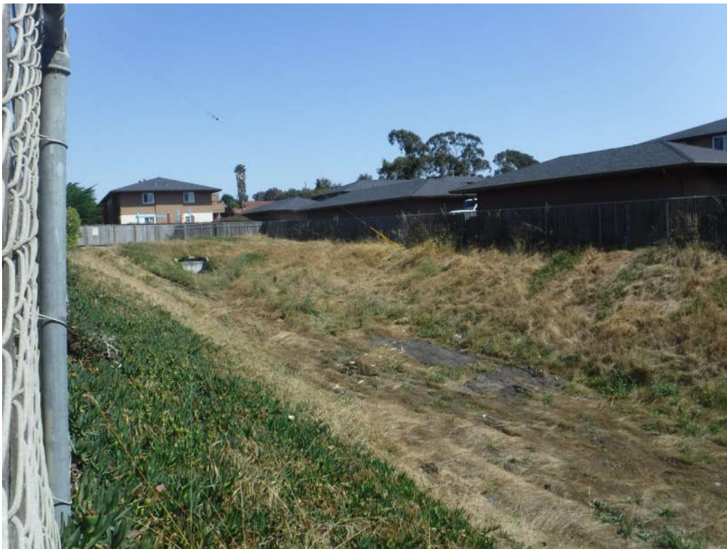
Photograph 8. The drainage south of Viking Avenue, facing east
