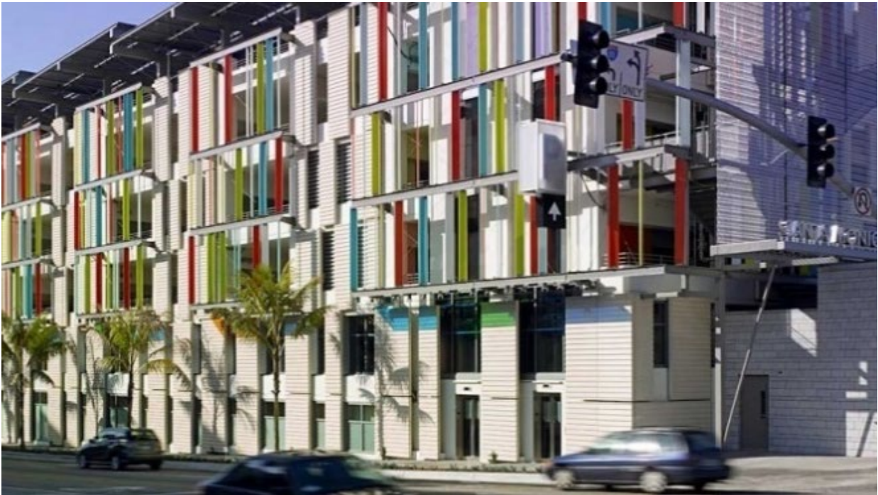
Articulation of parking structure façade. Façade may be articulated with interesting design elements and artwork. Source: Moore Ruble Yudell
