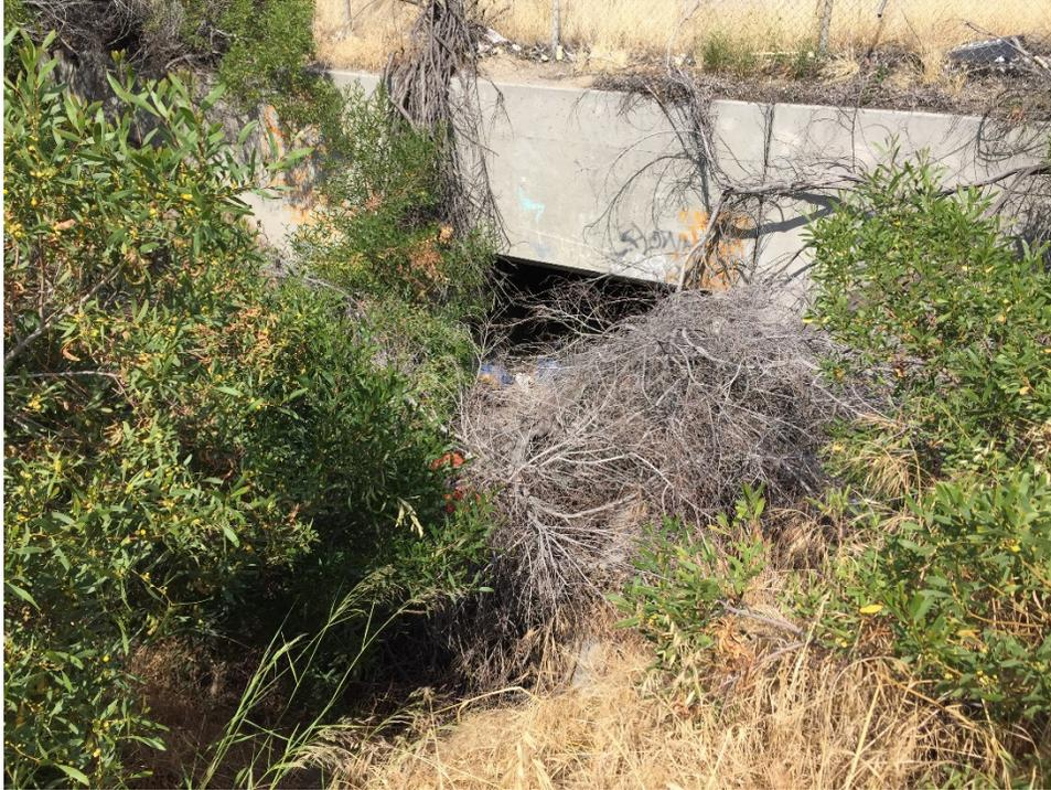
Photo 31 – A concrete culvert opening on the northwestern edge of the Property. Stormwater flows onto the Property from beneath the freeway.
